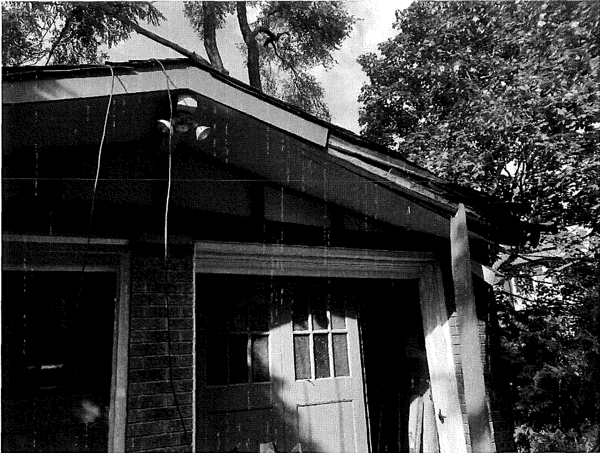
Photograph 2: Front Elevation - Original Brick (October 20, 2020)
