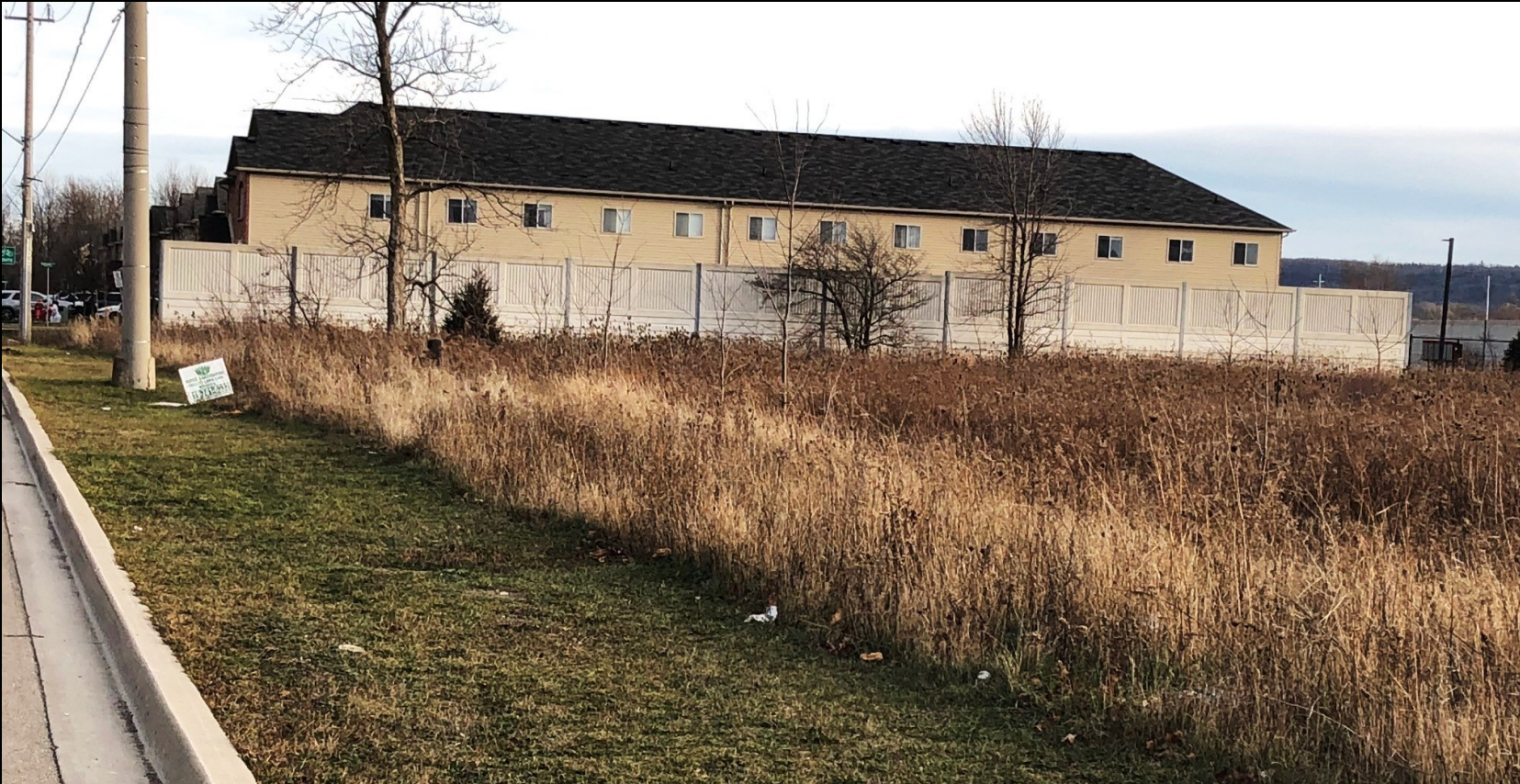
Property to the east
