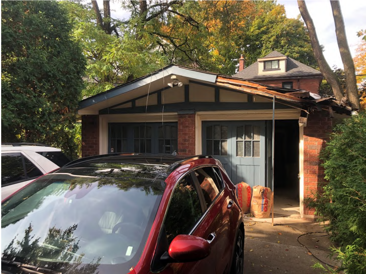
Image 1: Front of Building – Original Brick (October 20, 2020)
