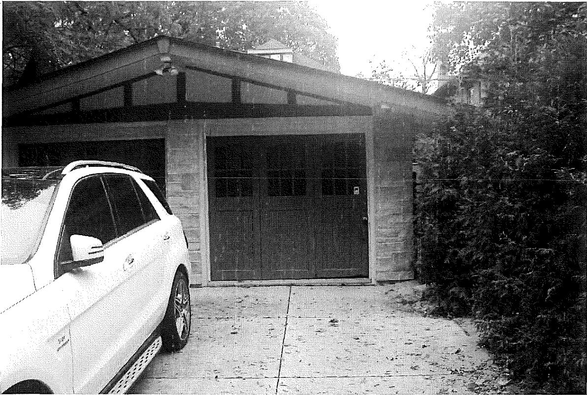
Photograph 4: New Wall Application (October 29, 2021)
