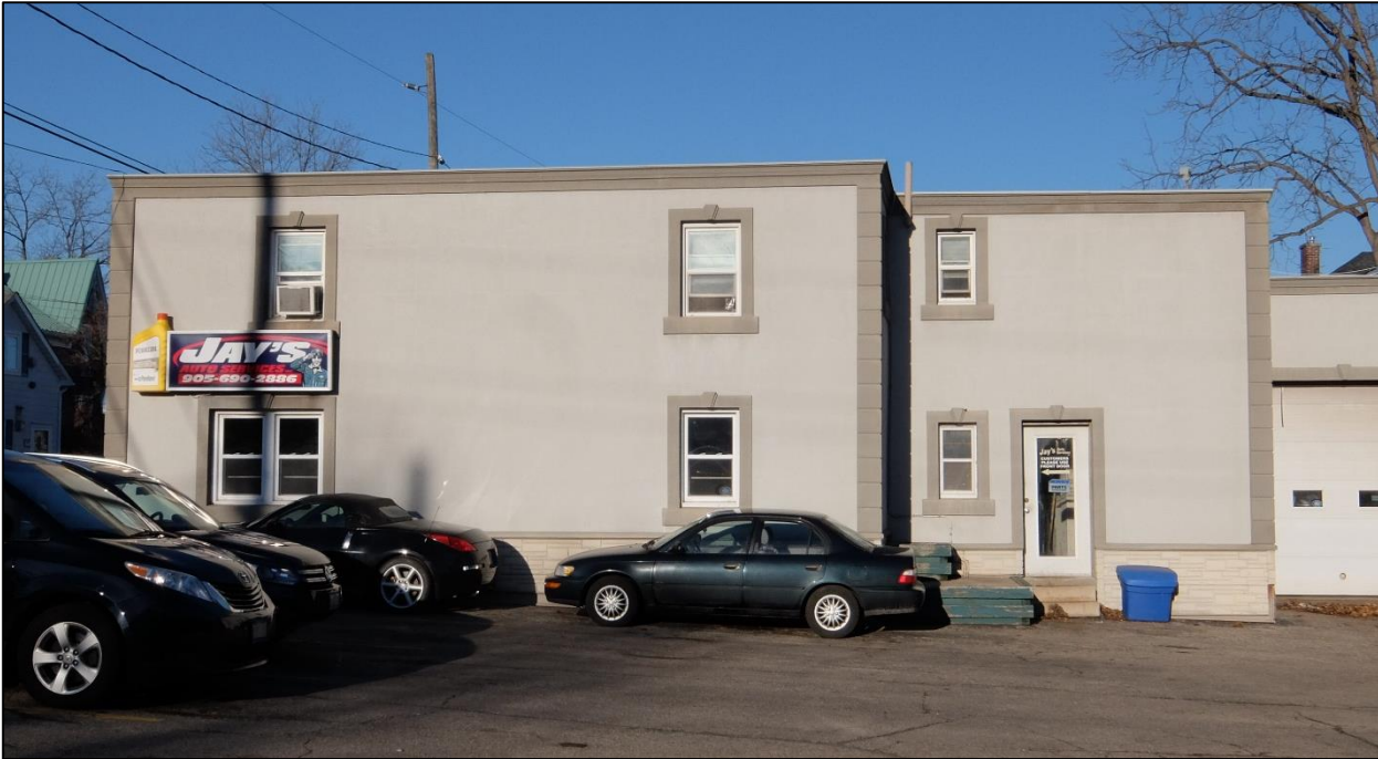
Image 5: 19 Flamboro Street side (south) facade clad in stucco, December 2021 (City of Hamilton)
