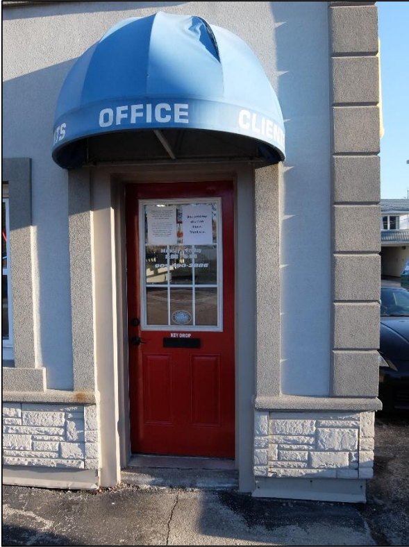
Image 9: Front commercial entrance, December 2021 (City of Hamilton)
