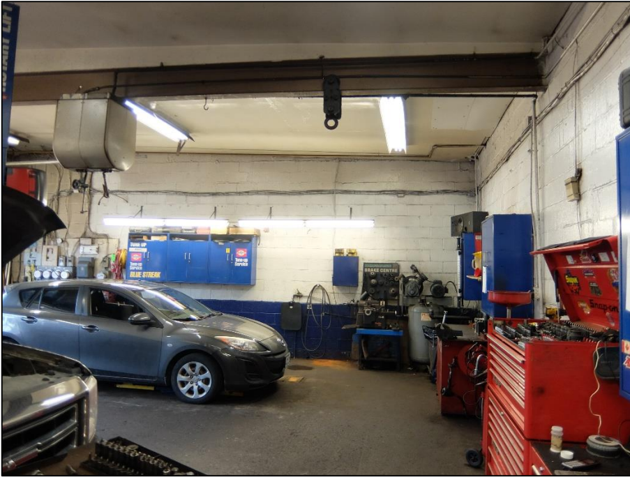
Image 11: First interior garage bay looking at north side concrete-block exterior wall, December 2021 (City of Hamilton)
