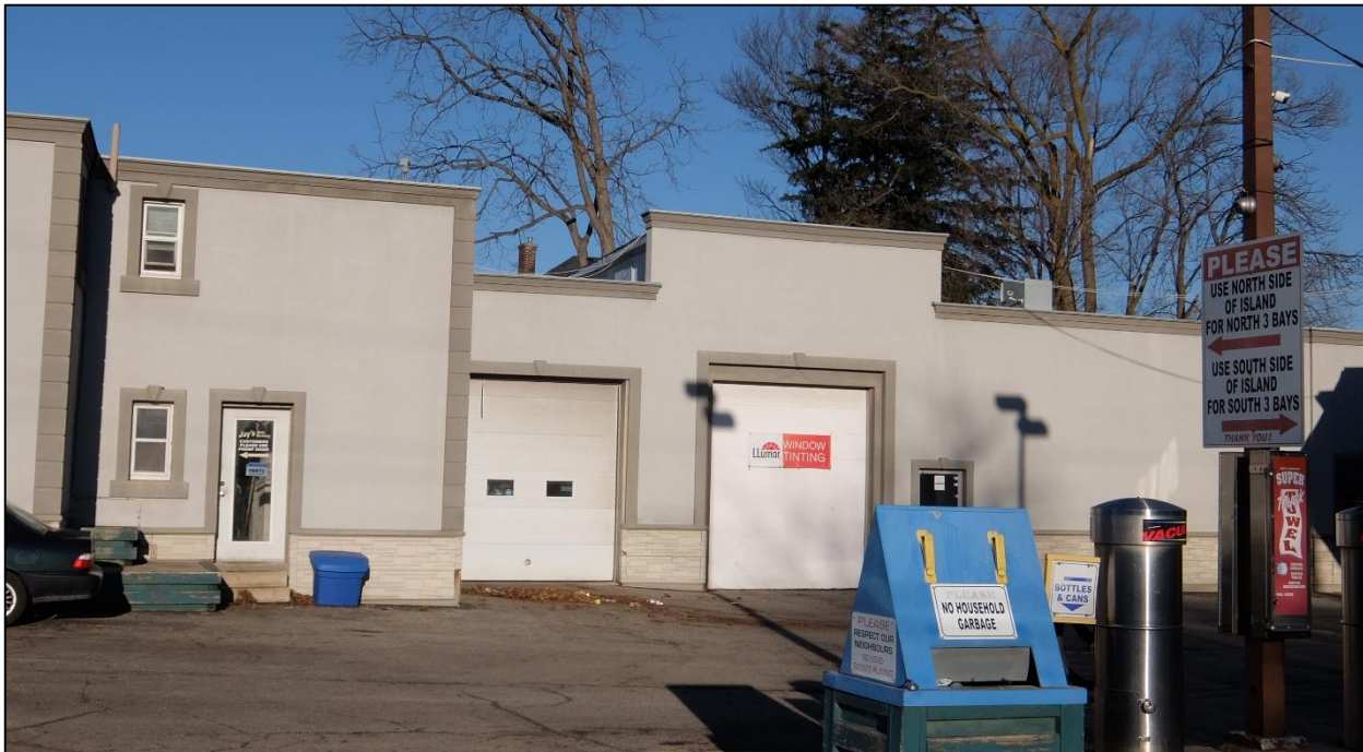
Image 6: 19 Flamboro Street rear addition, side (south) facade clad in stucco, December 2021 (City of Hamilton)
