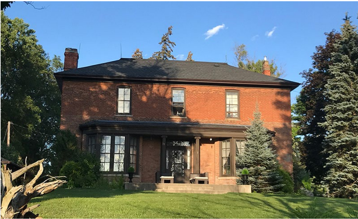
West façade showing the symmetrical façade, doorway with transom and side lights, the porch with Corinthian columns and the two hexagonal bay windows.
