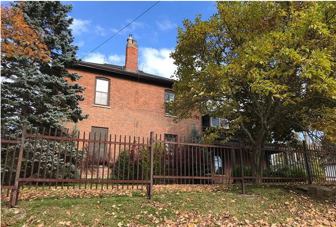
South façade facing Governor's Road showing one of two chimneys on the south and north sides of the house.
