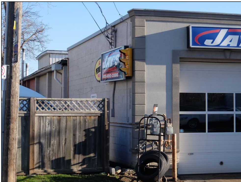
Image 8: 19 Flamboro Street side (north) concrete-block facade, December 2021 (City of Hamilton)
