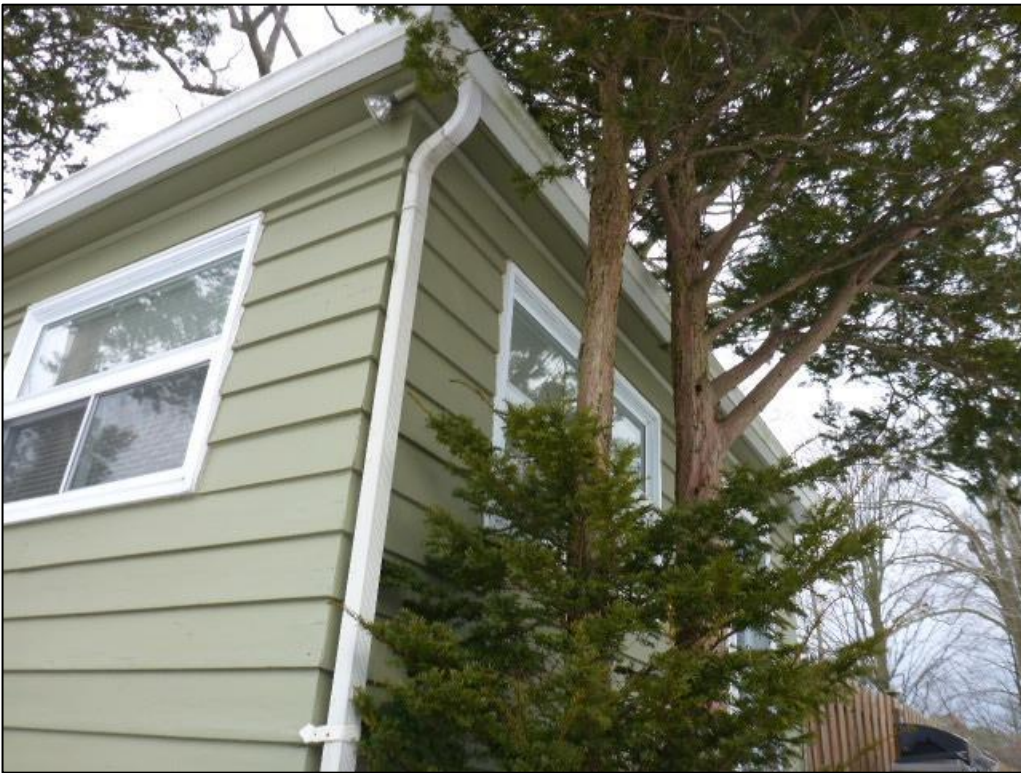
Image 4: Typical exterior siding and windows
