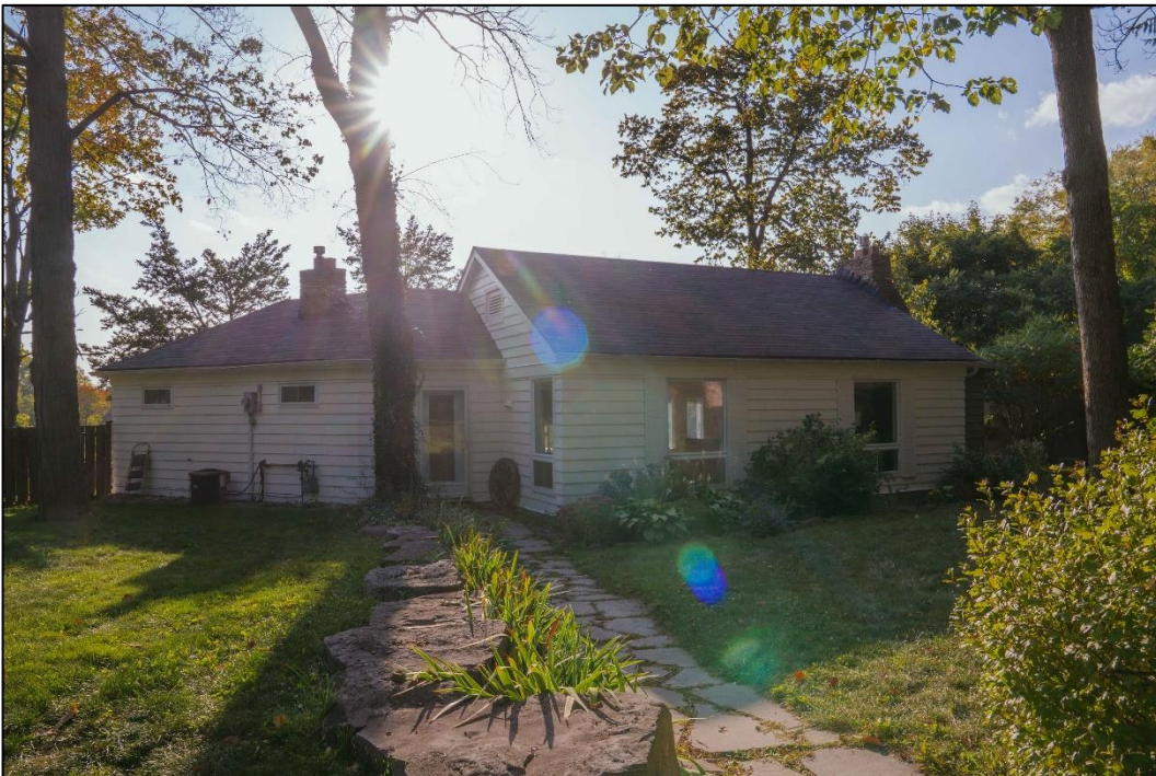
Image 2: Front façade, close-up
