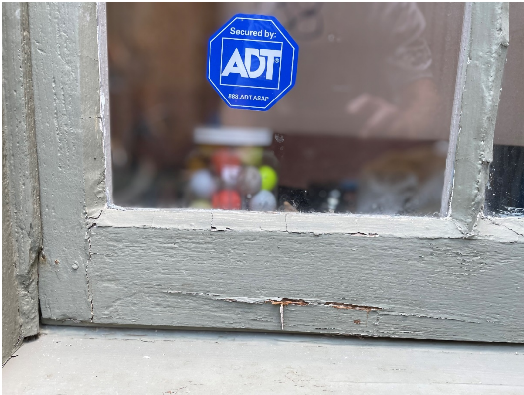
Existing window showing putty in poor condition, poorly fitted sash in frame. 7 windows were given to Jan Kamermans Hardware, Locks & Fastenings Specialist, 309 Caroline Street South, Hamilton. Jan uses the antique glass for his projects.
