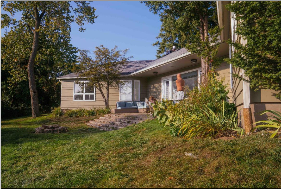
Image 3: Rear (west) exterior facades
