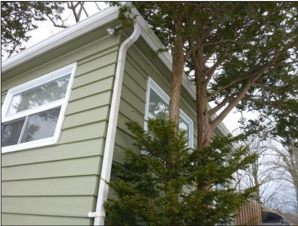
Image 4: Typical exterior siding and windows
