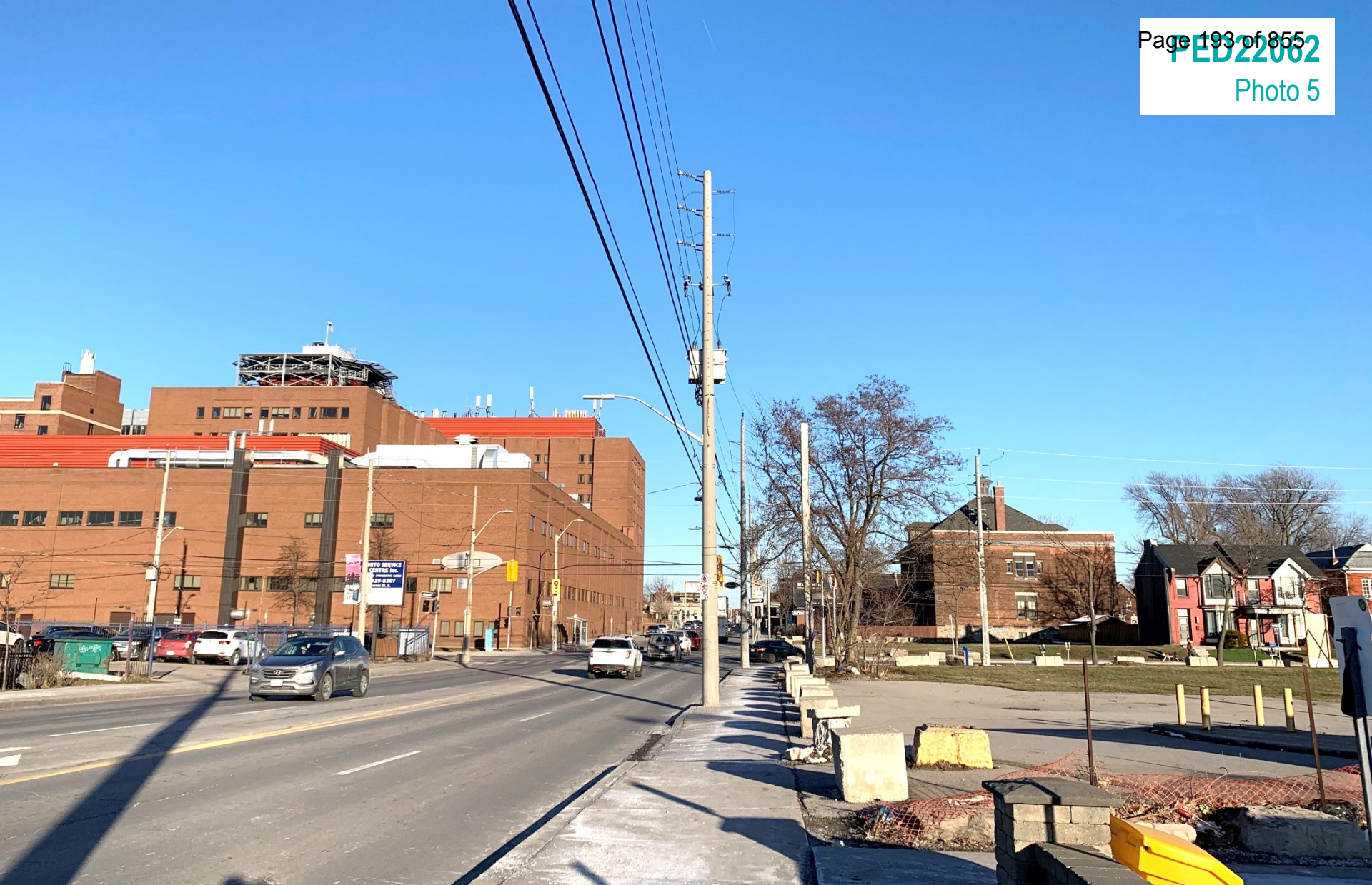
View of looking east on Barton Street East
