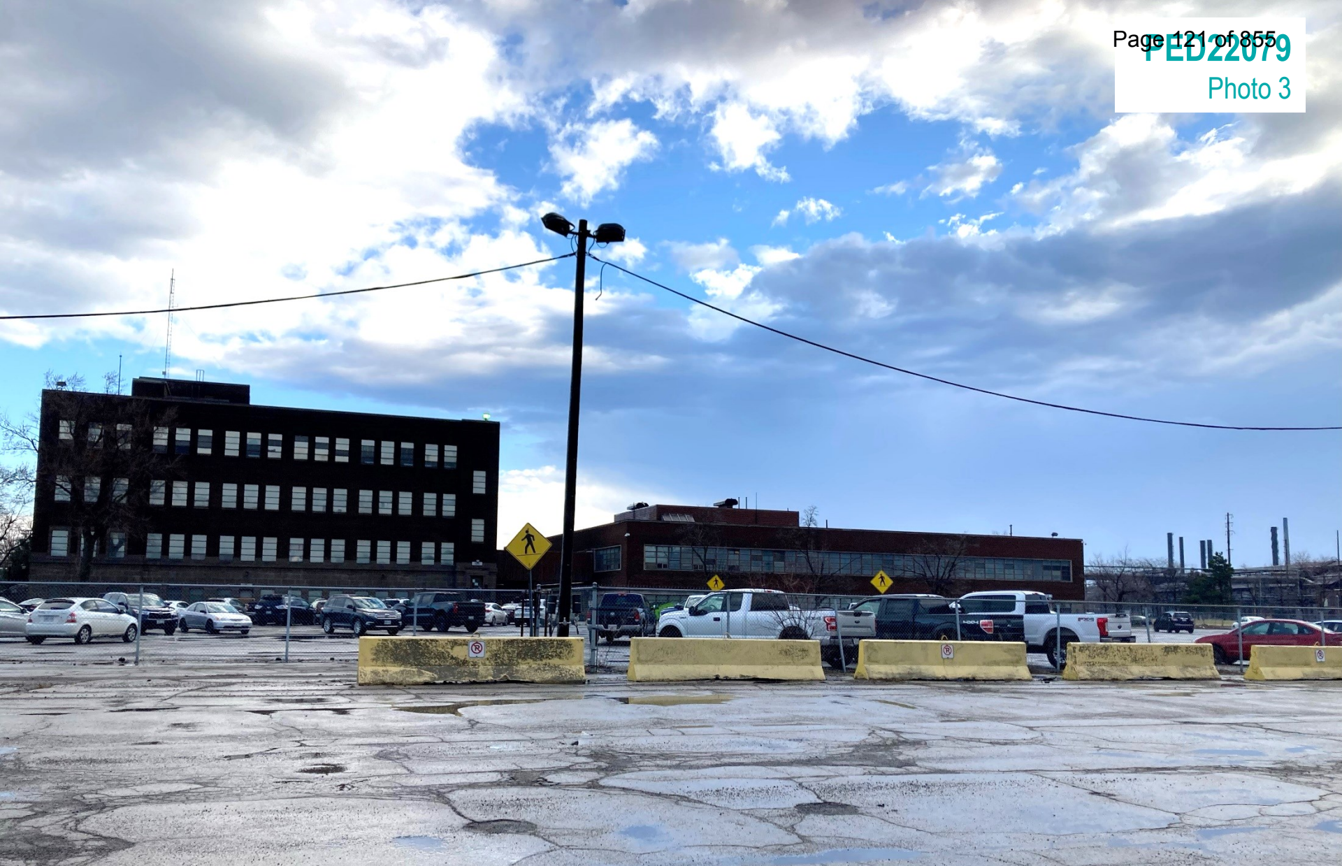
Looking north towards the Industrial lands
