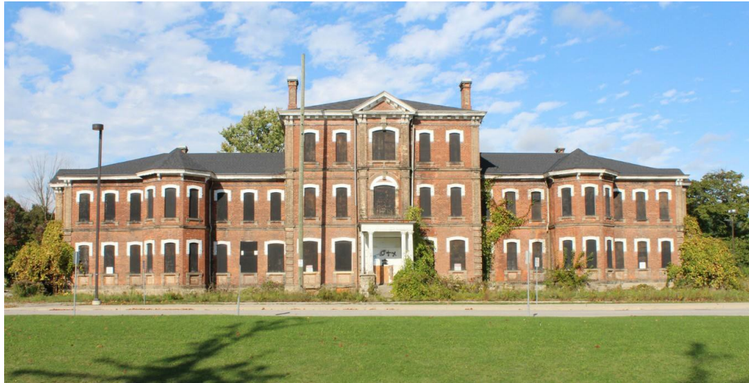
Front/ West Elevation of Century Manor
