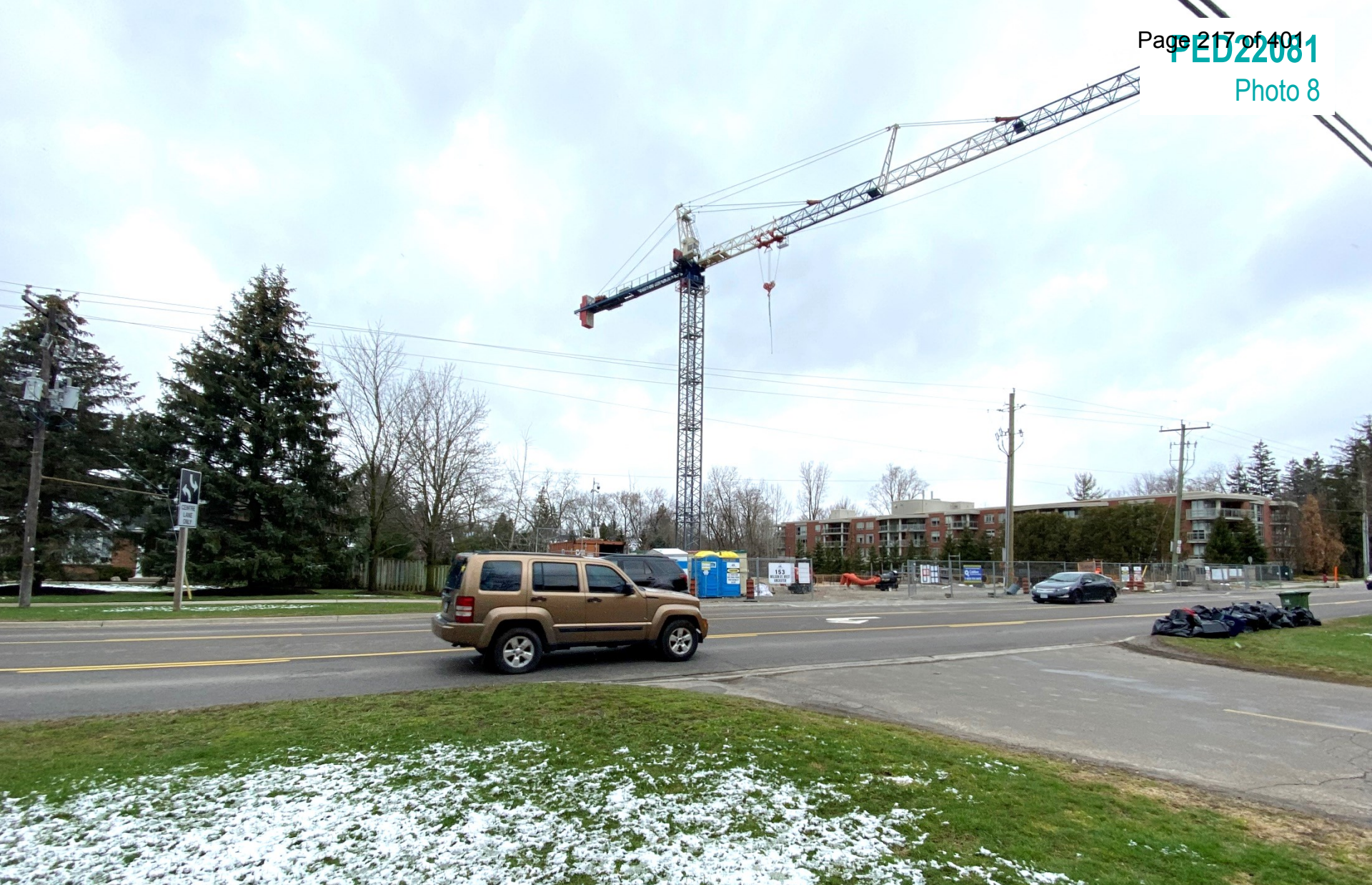
Building under construction at 153 Wilson Street West
