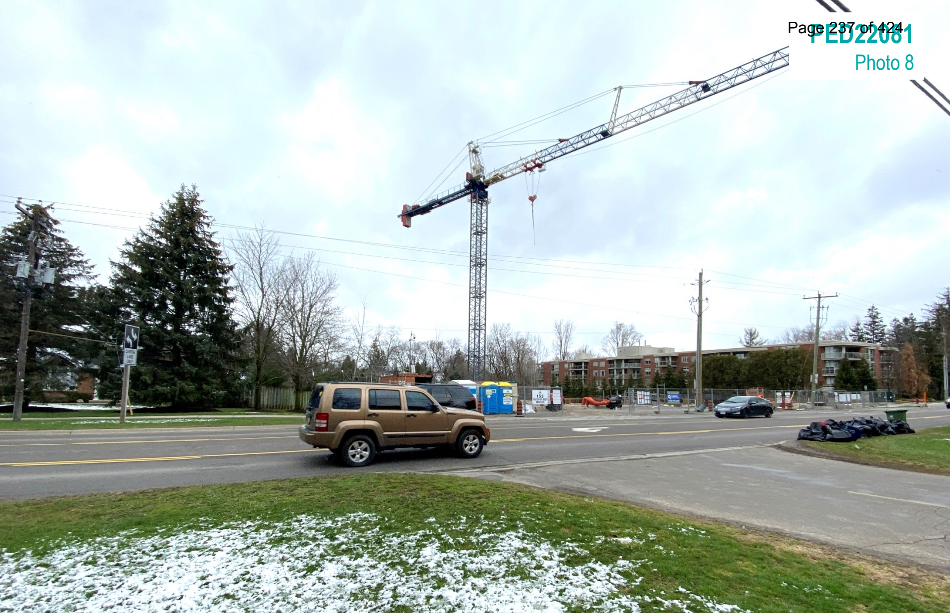
Building under construction at 153 Wilson Street West
