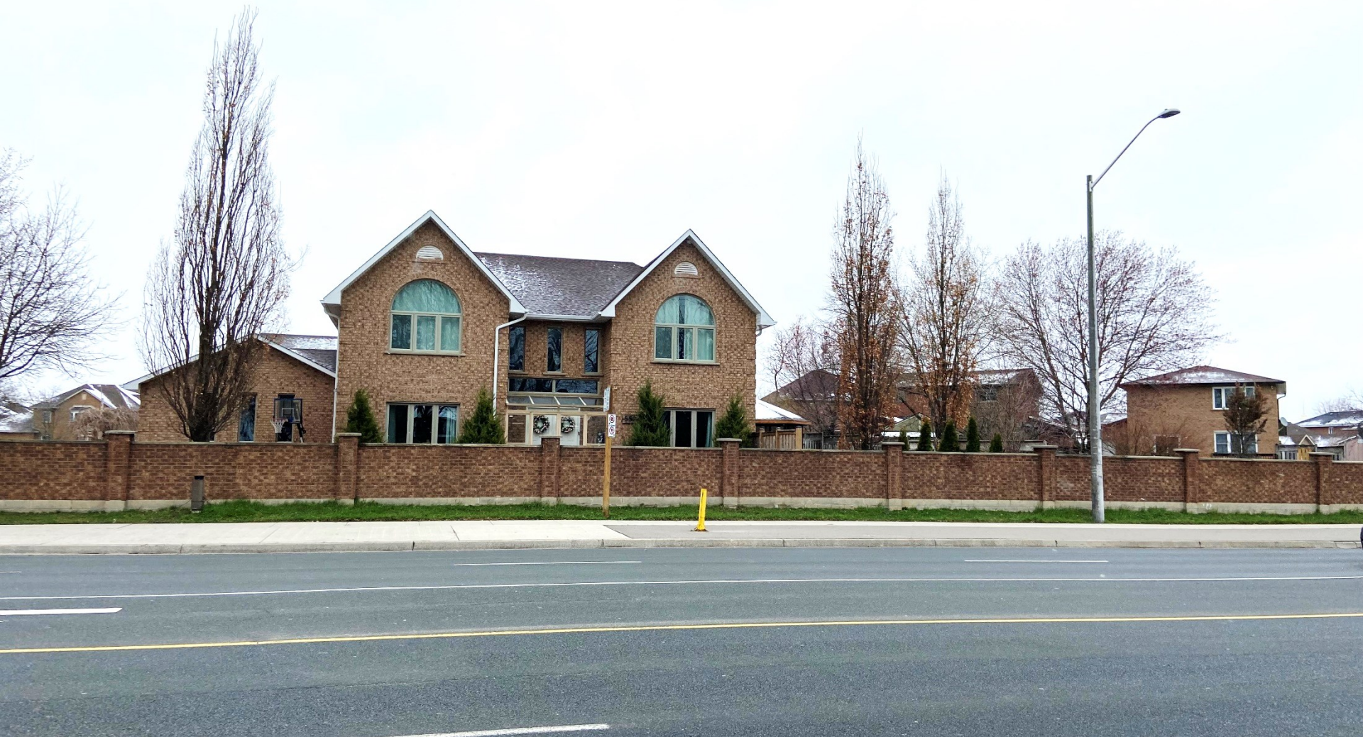
View looking north of Subject Lands
