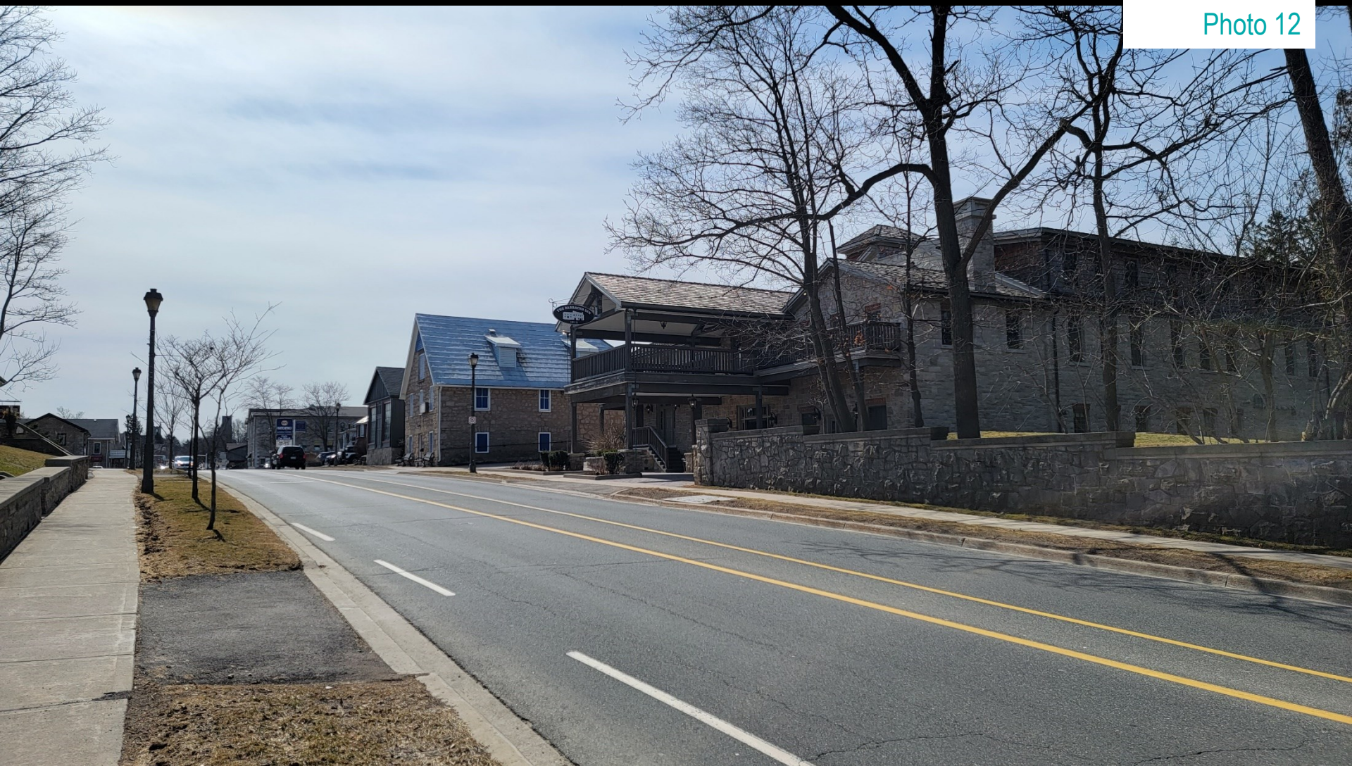
North of subject site along west side of Wilson Street East
