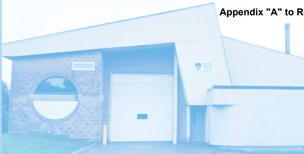
HPS Station 32, Limeridge Rd. E, Hamilton
