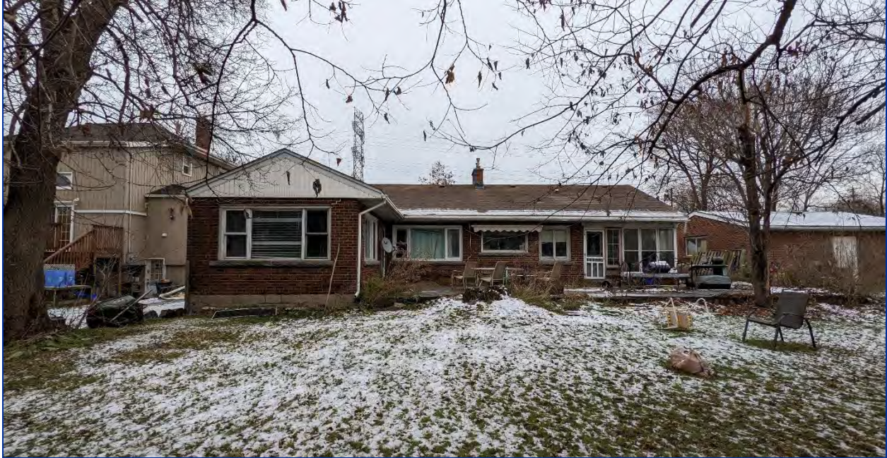
Figure 14: View of the west elevation of the residence and its rear addition
