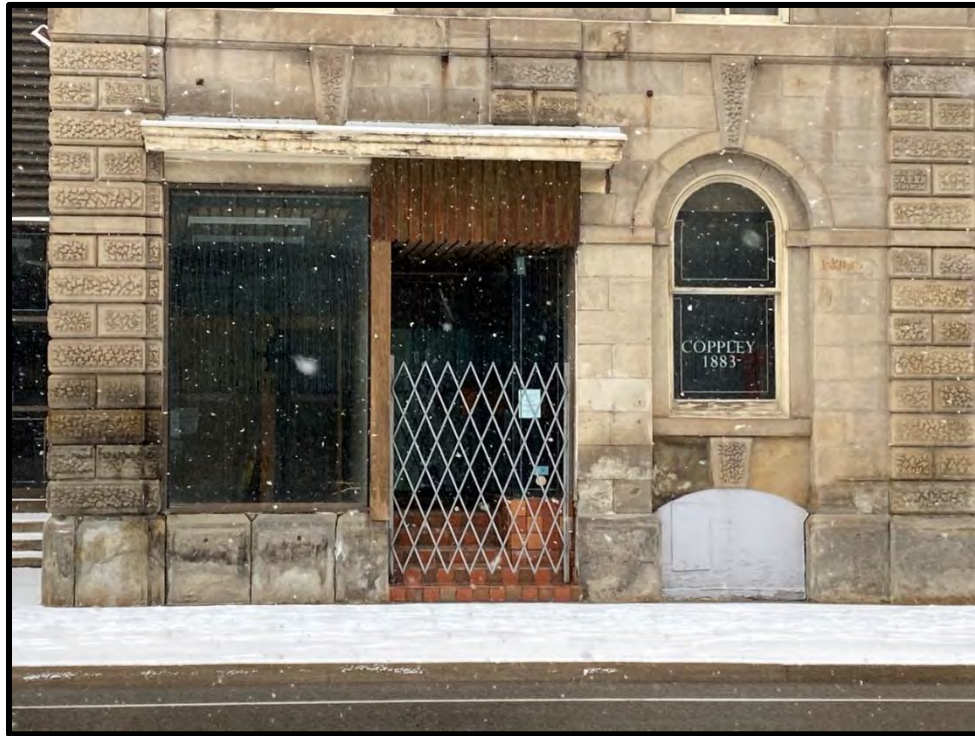
Image 5: York Street Entrance – Detail (Photo taken on December 8, 2021; Facing North)
