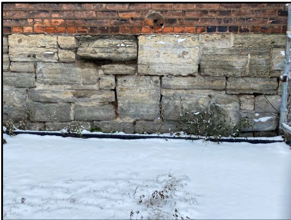
Image 44: Detail of Stone Foundation Brick Coursing on West Elevation (Photo taken on December 8, 2021; Facing East)
