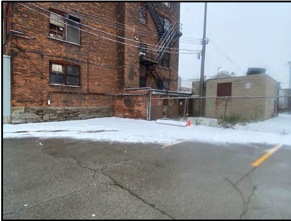
Image 49: North Elevation and Cinderblock Addition (Photo taken on December 8, 2021; Facing Southwest)
