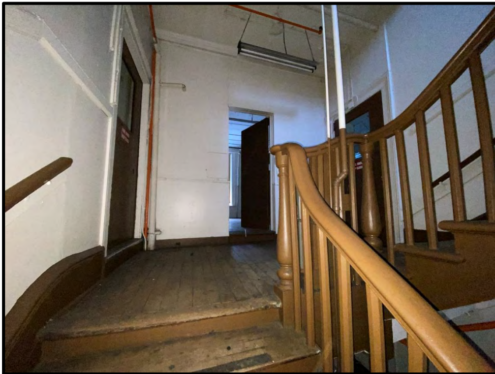
Image 98: Second Floor Stone Building – Landing (Photo taken on December 8, 2021)
