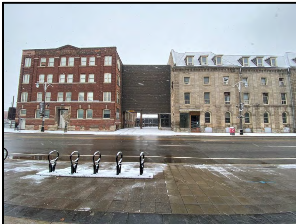
Image 36: York Street Front Façade Showing Entrance to Loading Area (Photo taken on December 8, 2021; Facing North)
