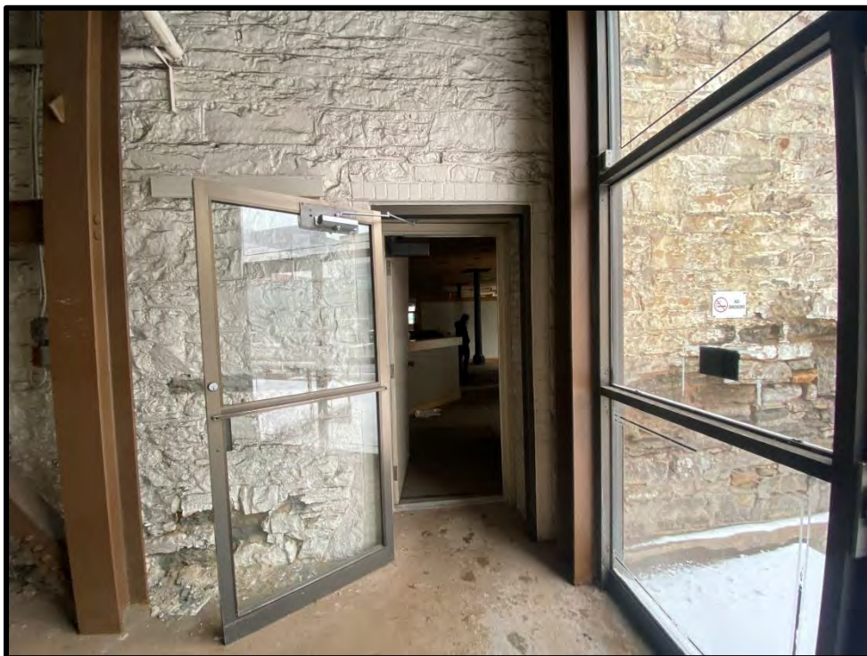
Image 56: West Elevation Entrance (Photo taken on December 8, 2021; Facing East)
