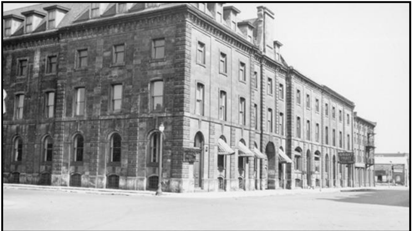
Plate 10: Stone Building at 56 York Boulevard (HPL LHA no date)
