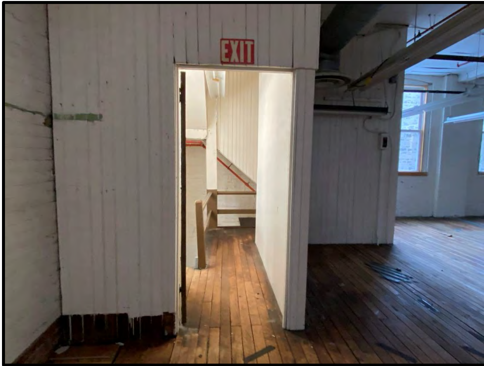
Image 177: Third Floor Brick Building – Stairwell (Photo taken on December 8, 2021; Facing East)
