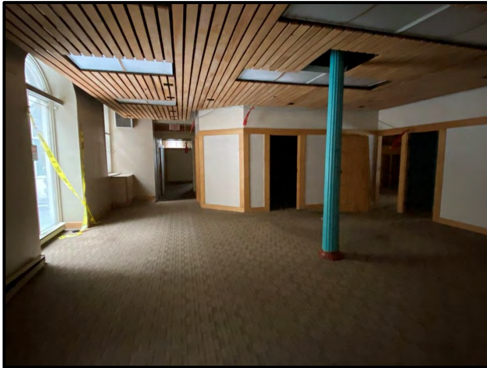
Image 69: First Floor – Interior (Measurements taken on December 8, 2021; Facing South)
