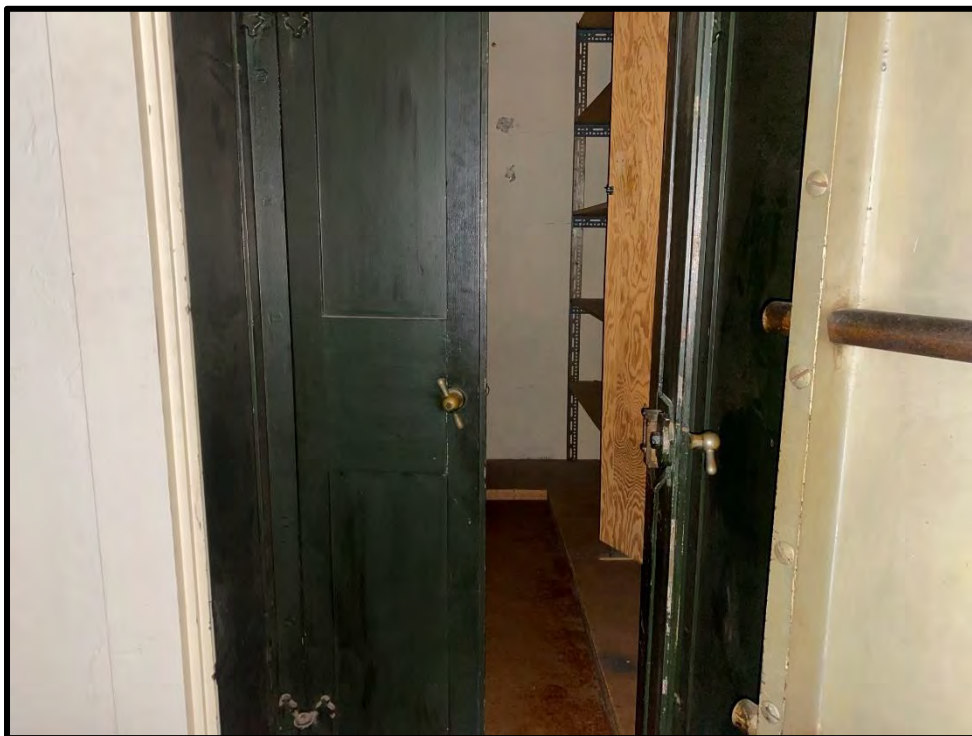
Image 82: First Floor North Addition – Vault Detail (Photo taken on December 8, 2021; Facing West)
