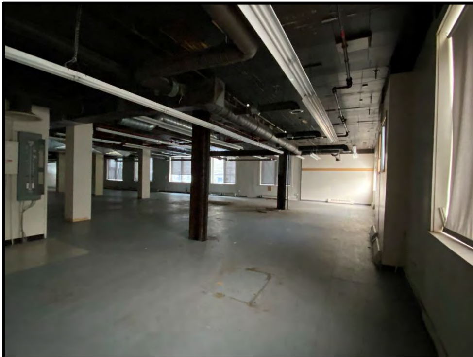
Image 160: First Floor Brick Building – Interior (Photo taken on December 8, 2021; Facing Northeast)
