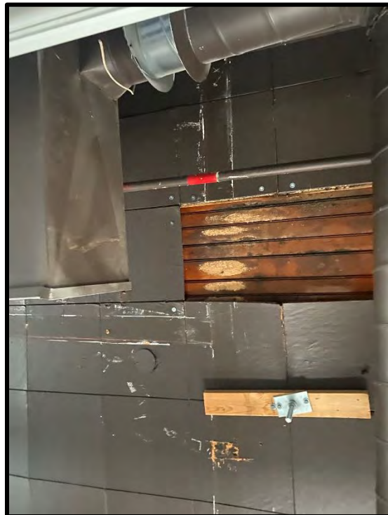
Image 164: First Floor Brick Building – Ceiling Detail (Photo taken on December 8, 2021)
