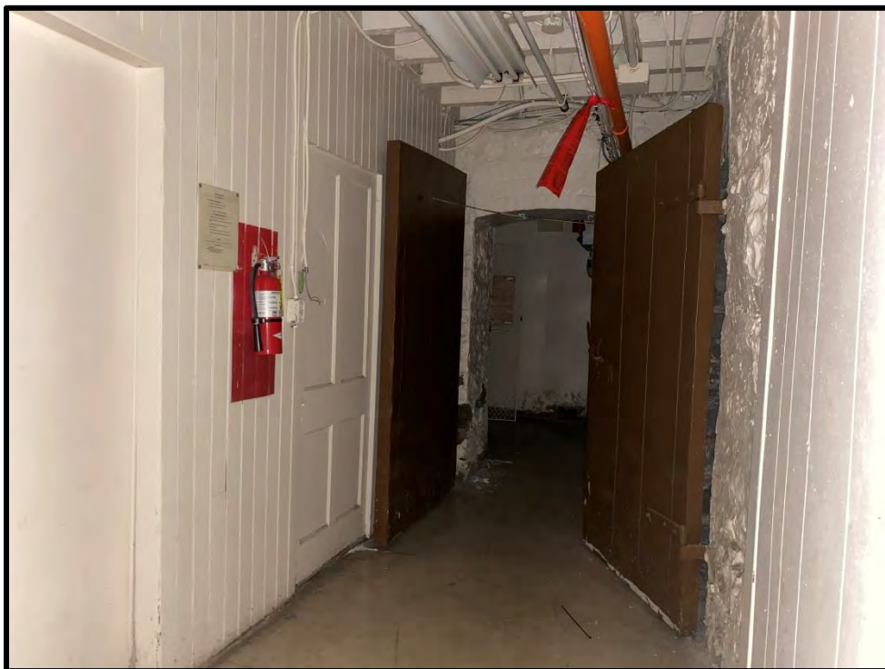
Image 180: Basement Brick Building – Entryway (Photo taken on December 8, 2021)
