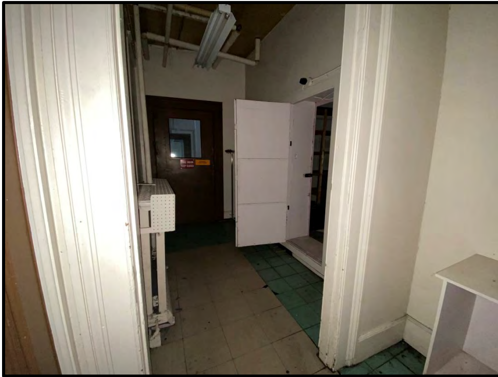
Image 121: Second Floor North Addition – Vault (Photo taken on December 8, 2021)
