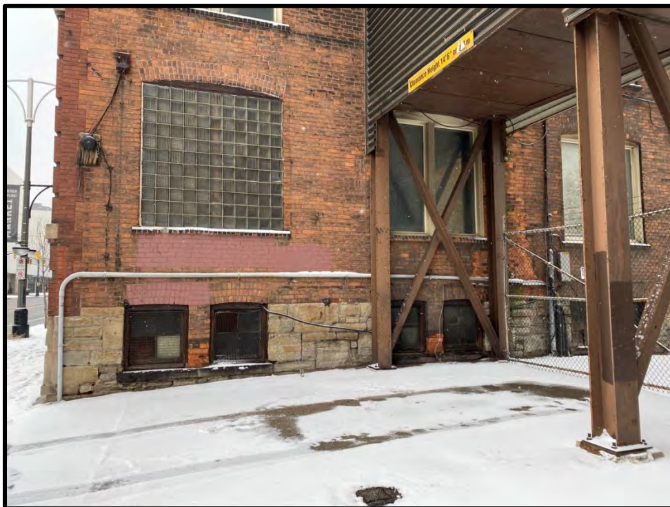
Image 54: Detail of East Elevation (Photo taken on December 8, 2021; Facing West)
