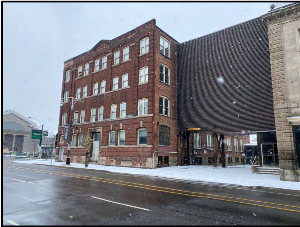
Image 53: South and East Elevations (Photo taken on December 8, 2021; Facing Northwest)
