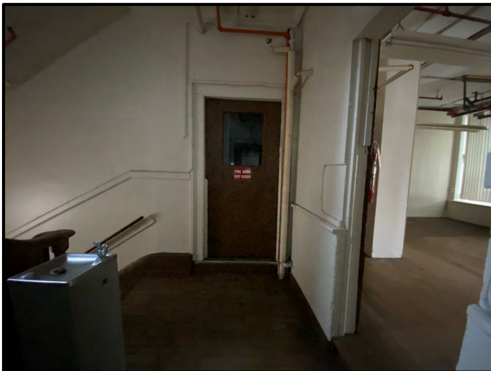
Image 100: Second Floor Stone Building – Interior (Photo taken on December 8, 2021)
