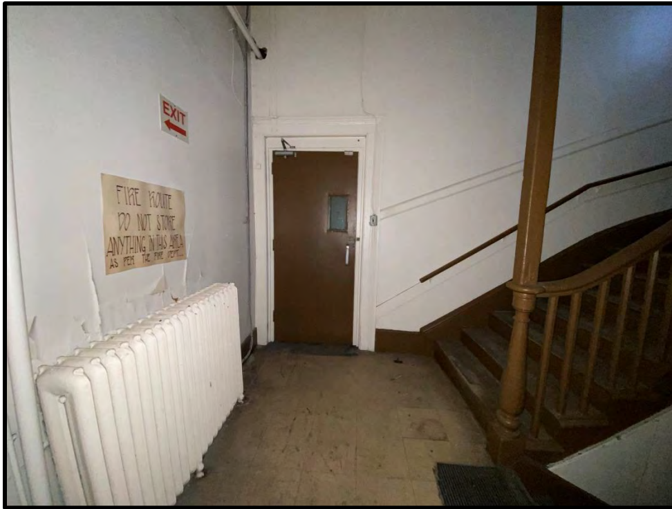
Image 93: First Floor North Addition – Stair Landing - Interior (Photo taken on December 8, 2021)
