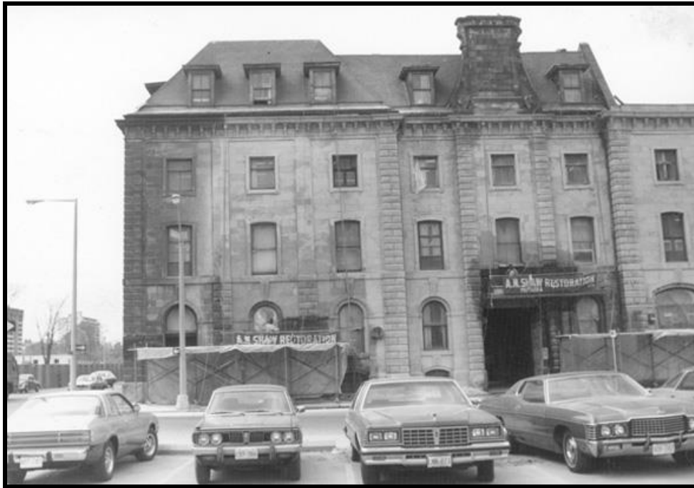
Plate 15: Restoration in Progress at 63-73 MacNab Street (HPL LHA 1978)
