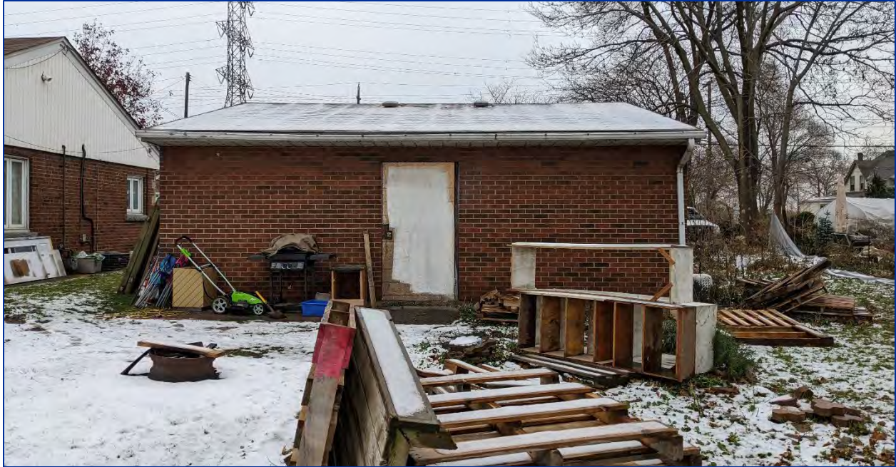
Figure 23: View of the west elevation of the detached garage
