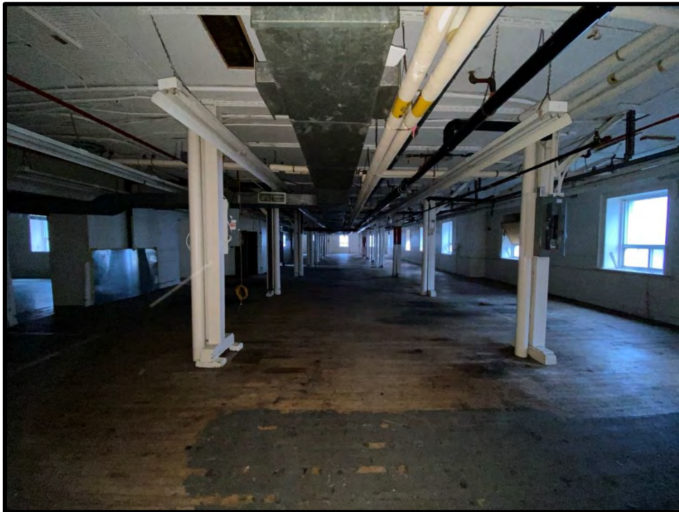
Image 130: Third Floor – Interior (Photo taken on December 8, 2021; Facing East)
