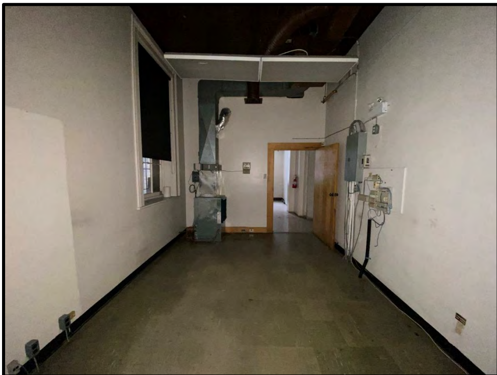
Image 86: First Floor North Addition – Interior (Photo taken on December 8, 2021; Facing West)
