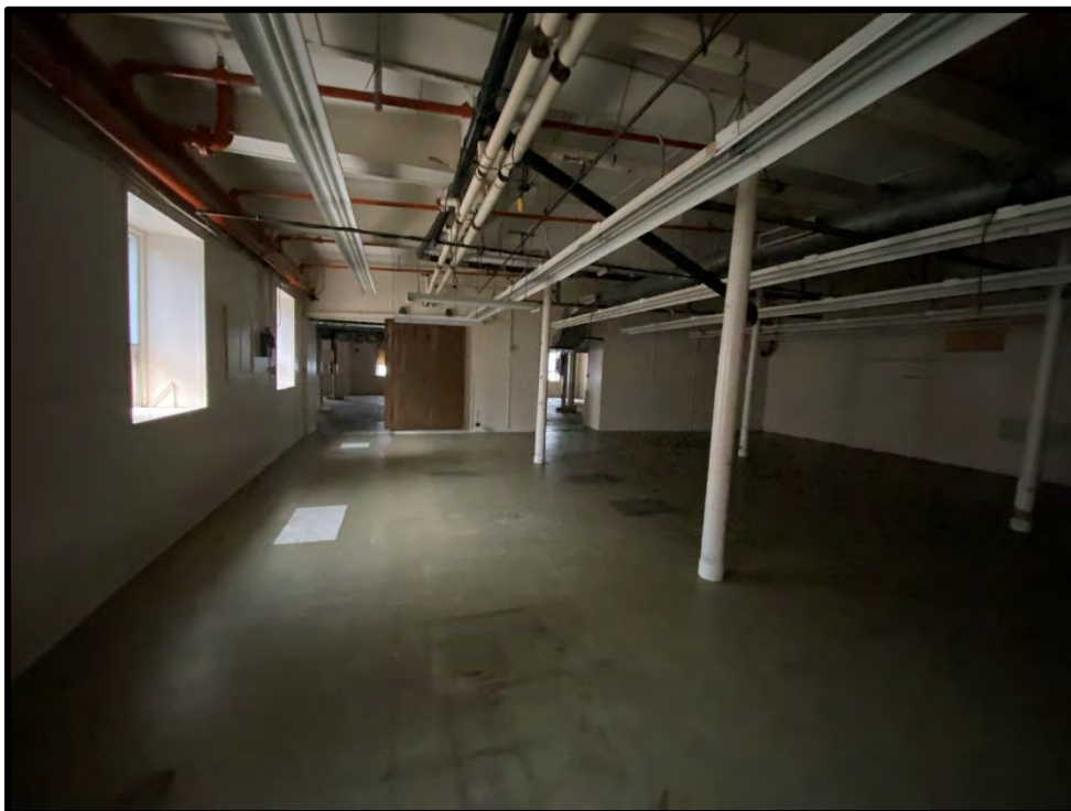
Image 128: Third Floor Stone Building – Interior (Photo taken on December 8, 2021; Facing West)
