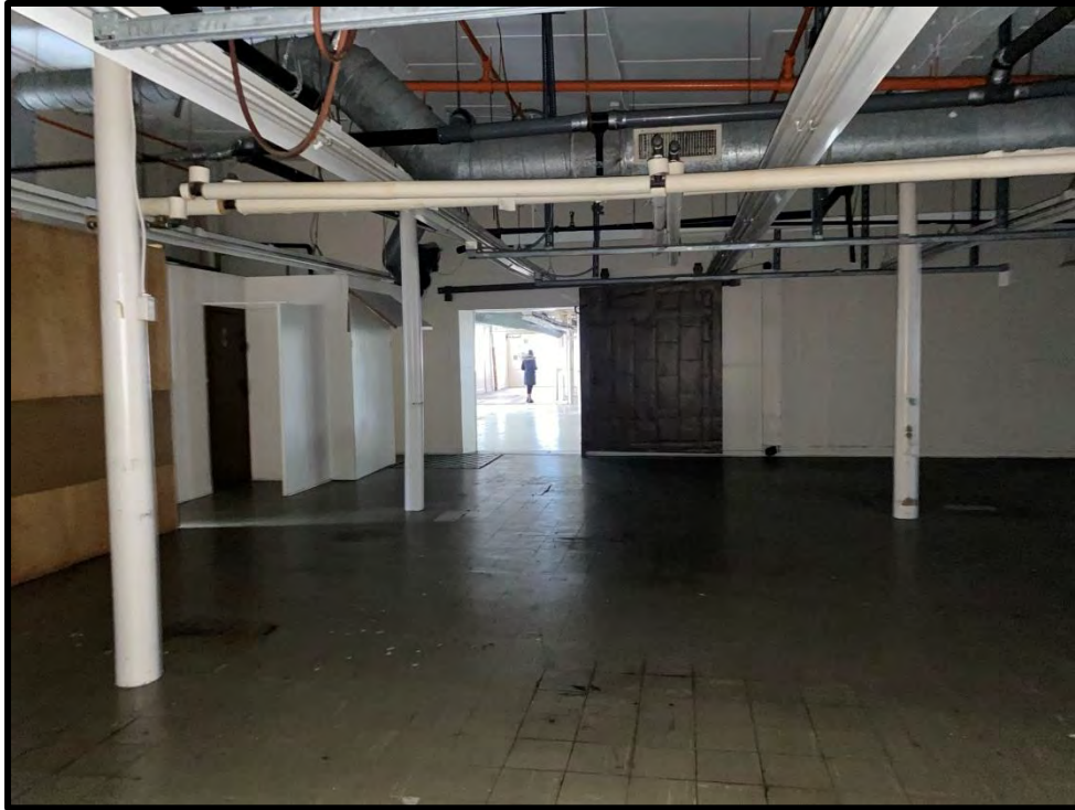
Image 125: Third Floor Stone Building – Interior (Photo taken on December 8, 2021; Facing West)
