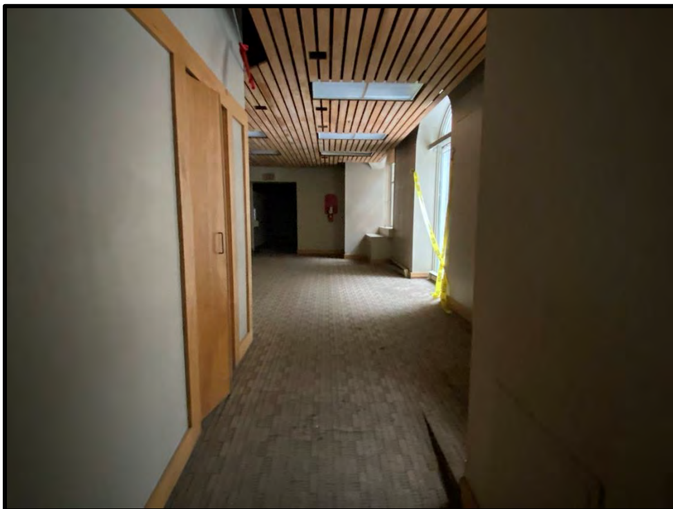
Image 68: First Floor – Interior (Photo taken on December 8, 2021; Facing North)
