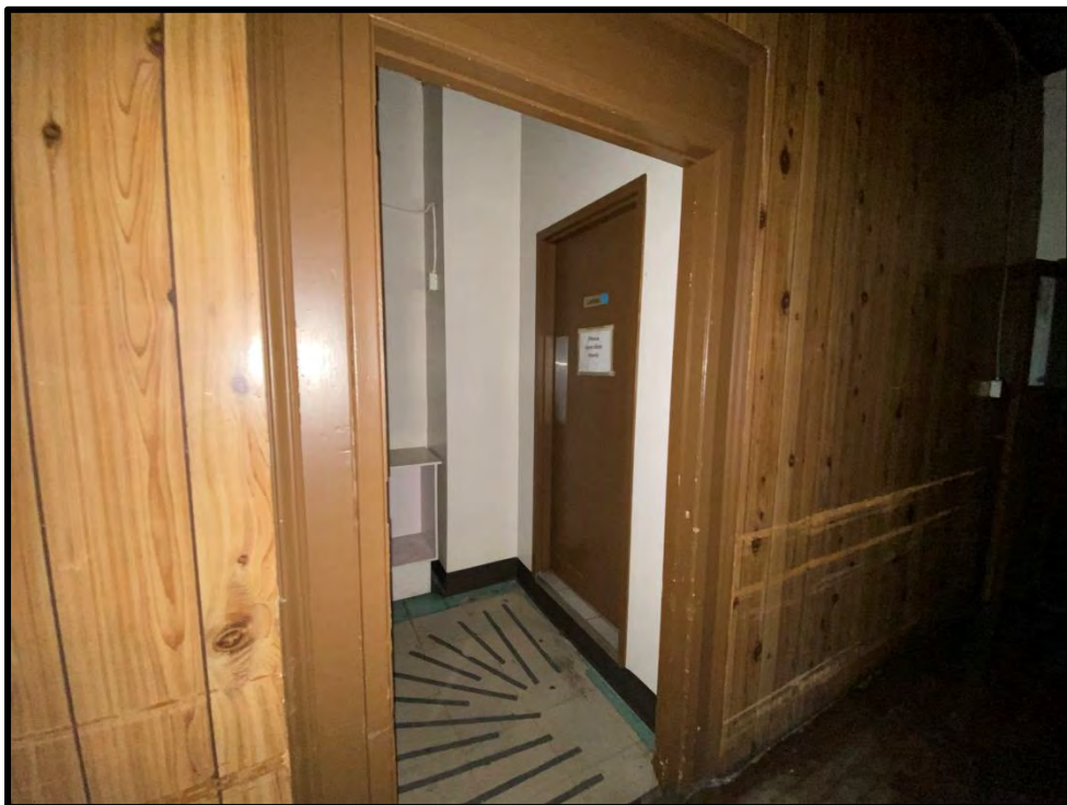
Image 120: Second Floor North Addition – Interior (Photo taken on December 8, 2021; Facing West)
