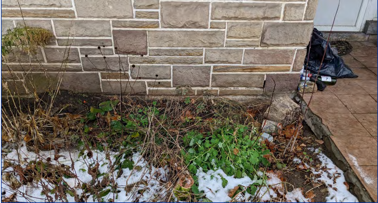
Figure 16: View of the residence's concrete foundation
