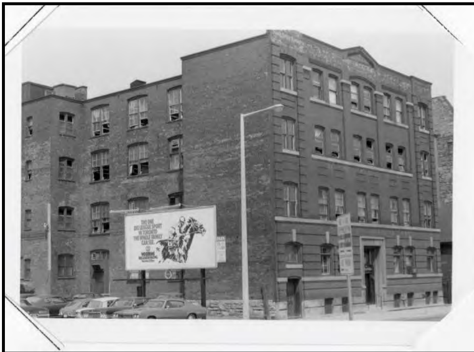
Plate 18: Brick Building at 56 York Boulevard, no date (Provided by the City of Hamilton)
