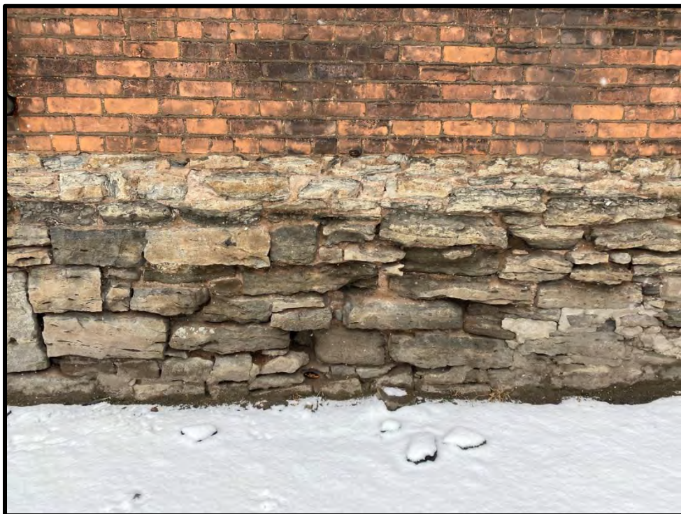
Image 52: Common Bond Brick Coursing and Uncoursed Stone Foundation – Detail (Photo taken on December 8, 2021; Facing South)
