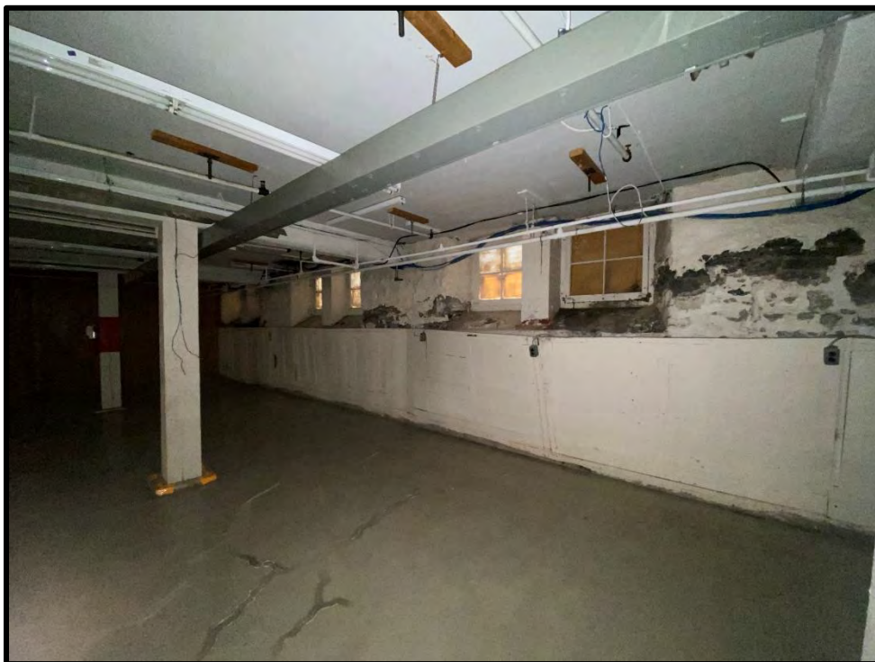
Image 184: Basement Brick Building – Interior (Photo taken on December 8, 2021)
