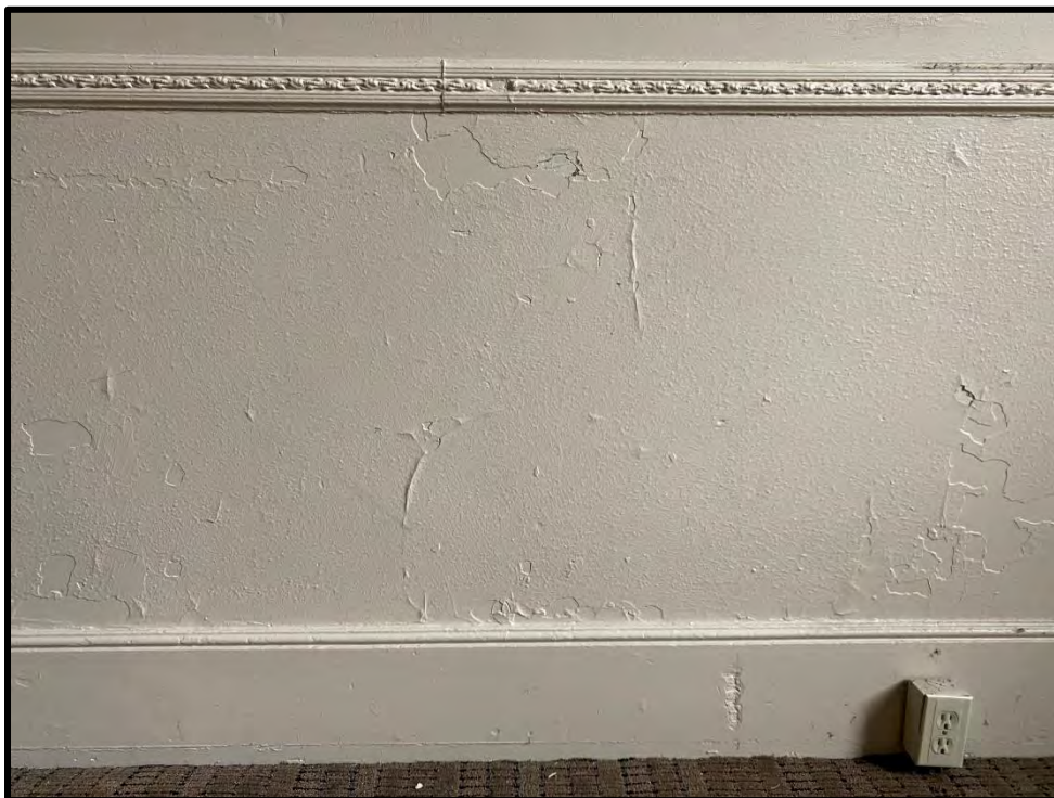
Image 64: First Floor – Interior Detail Chair Rail (Photo taken on December 8, 2021; Facing North)
