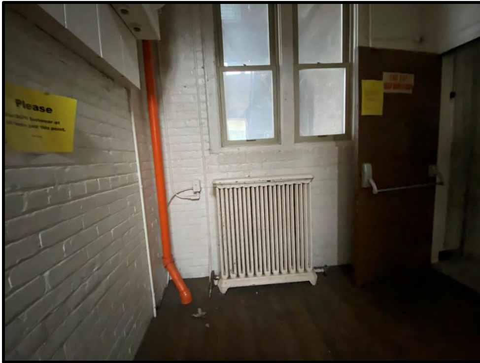
Image 157: First Floor Brick Building – Interior (Photo taken on December 8, 2021; Facing North)
