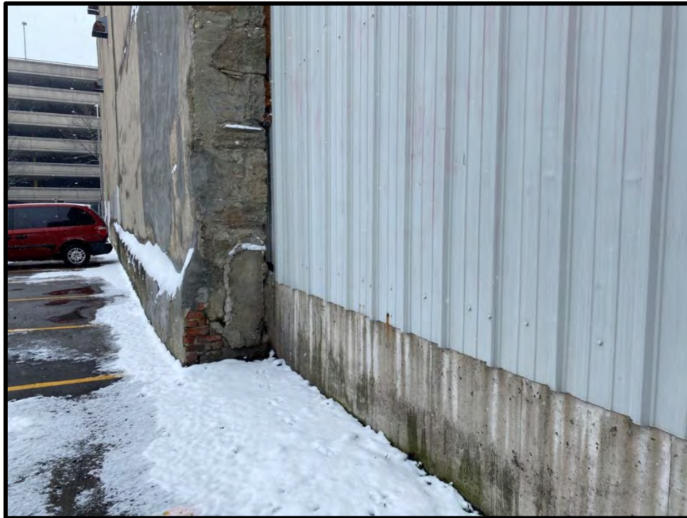
Image 19: Foundation and Concrete Walkway – Detail (Photo taken on December 8, 2021; Facing Southeast)
