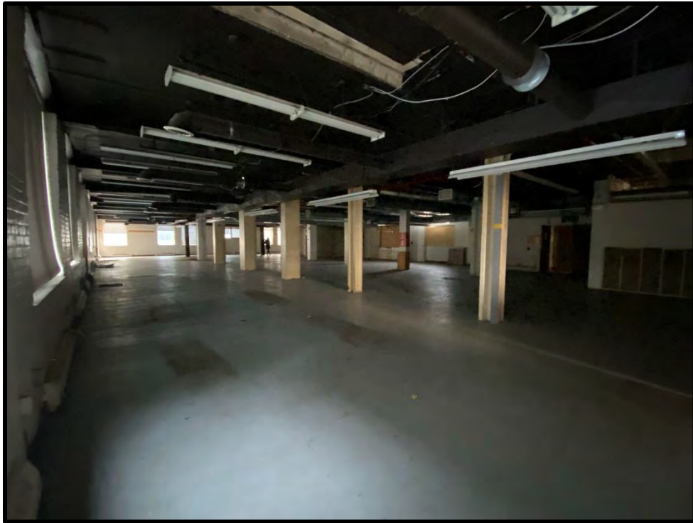
Image 165: First Floor Brick Building – Interior (Photo taken on December 8, 2021; Facing Southwest)
