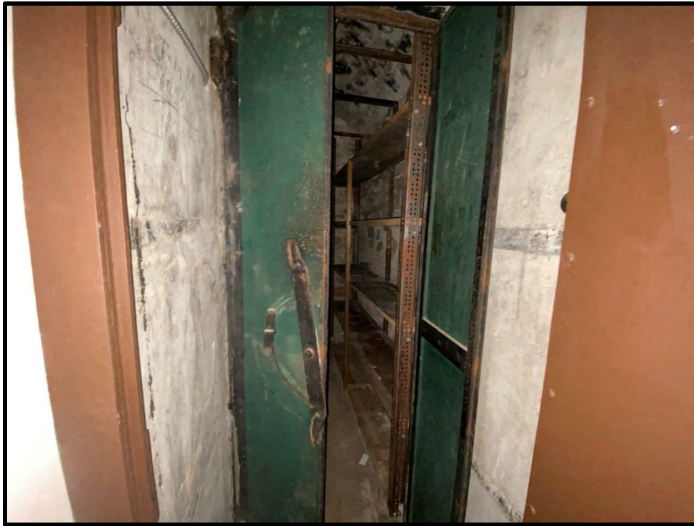
Image 155: Basement Stone Building – Vault Detail (Photo taken on December 8, 2021)
