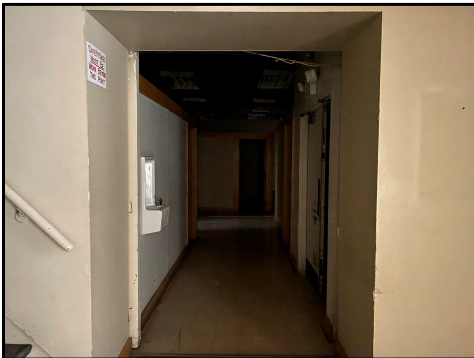
Image 76: First Floor Entrance to North Addition – Interior (Photo taken on December 8, 2021; North)
