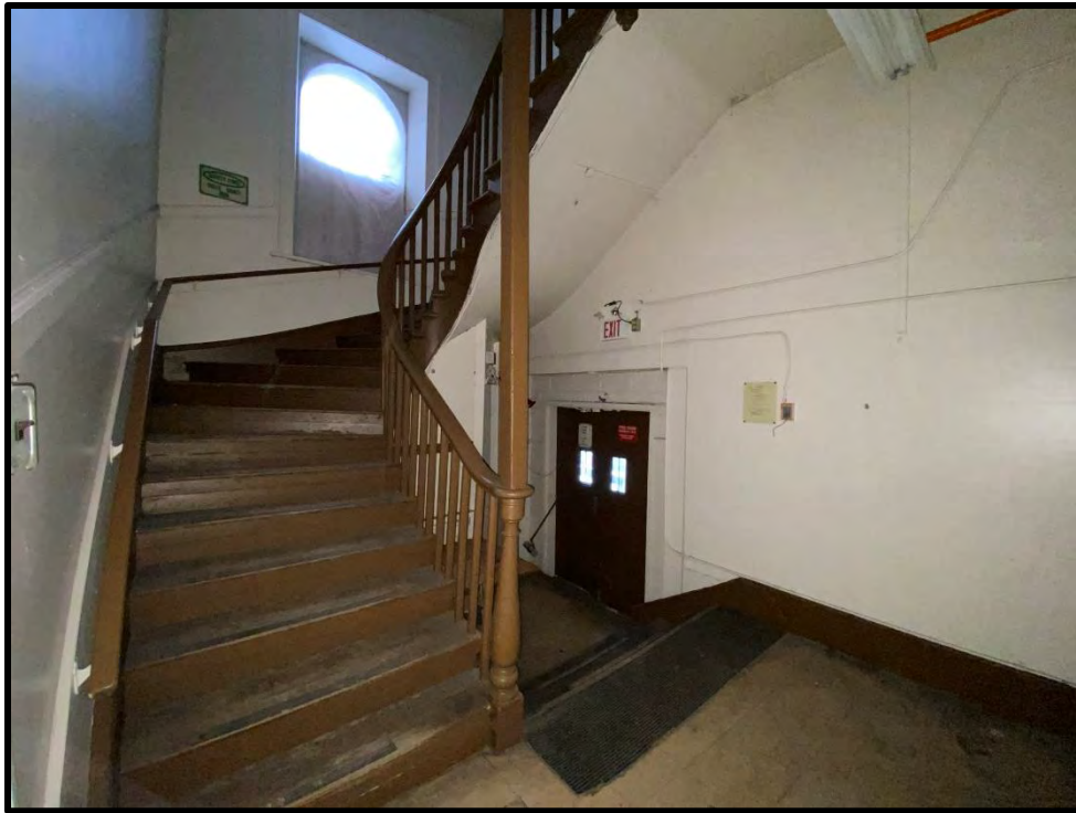
Image 95: First Floor North Addition – Staircase (Photo taken on December 8, 2021)
