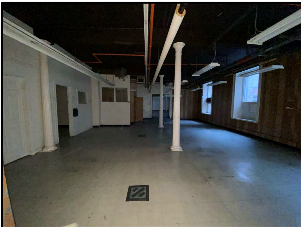
Image 112: Second Floor Stone Building – Interior (Photo taken on December 8, 2021; Facing North)
