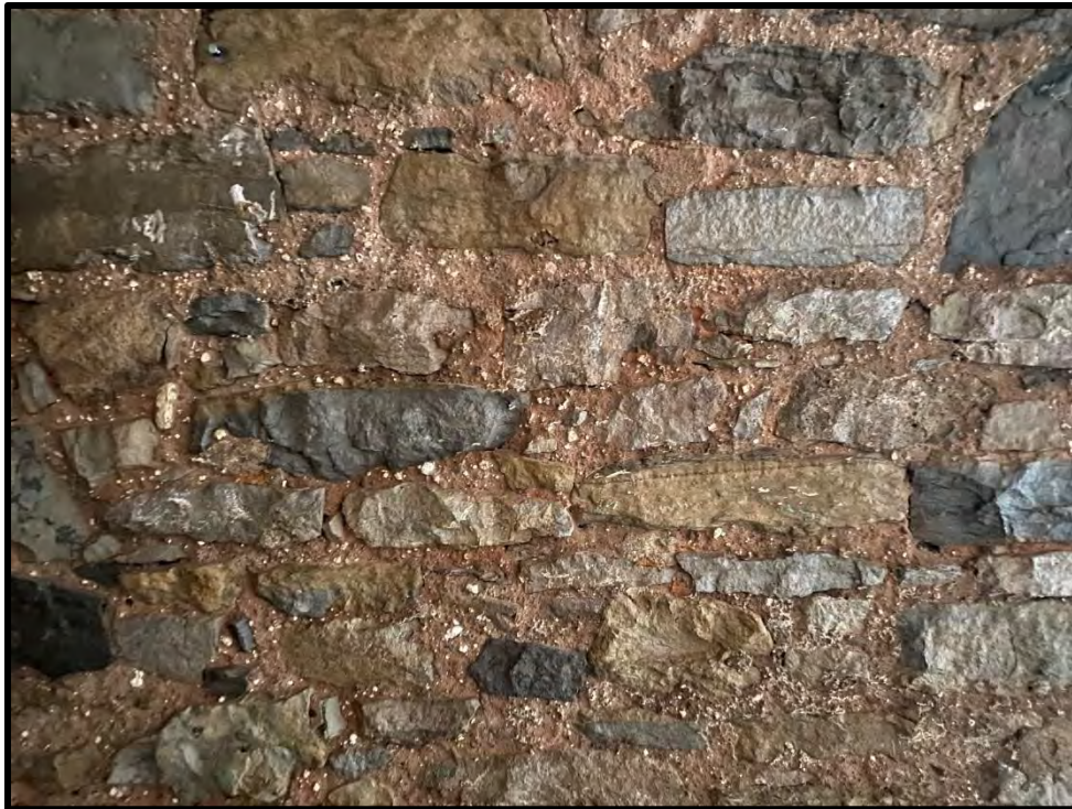
Image 73: Interior Stone Wall – Detail (Photo taken on December 8, 2021; Facing West)
