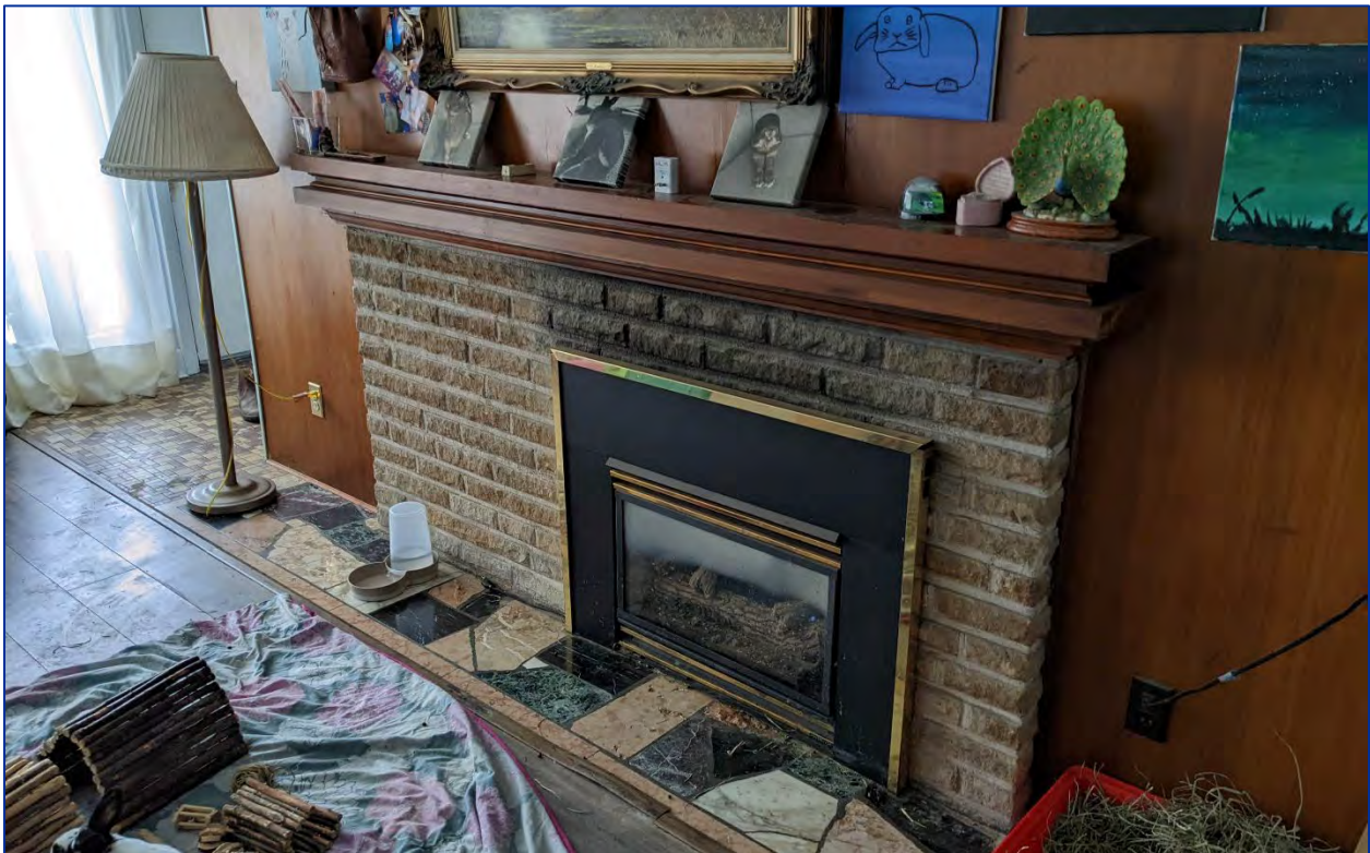
Figure 17: View of the fireplace and the front foyer floor
