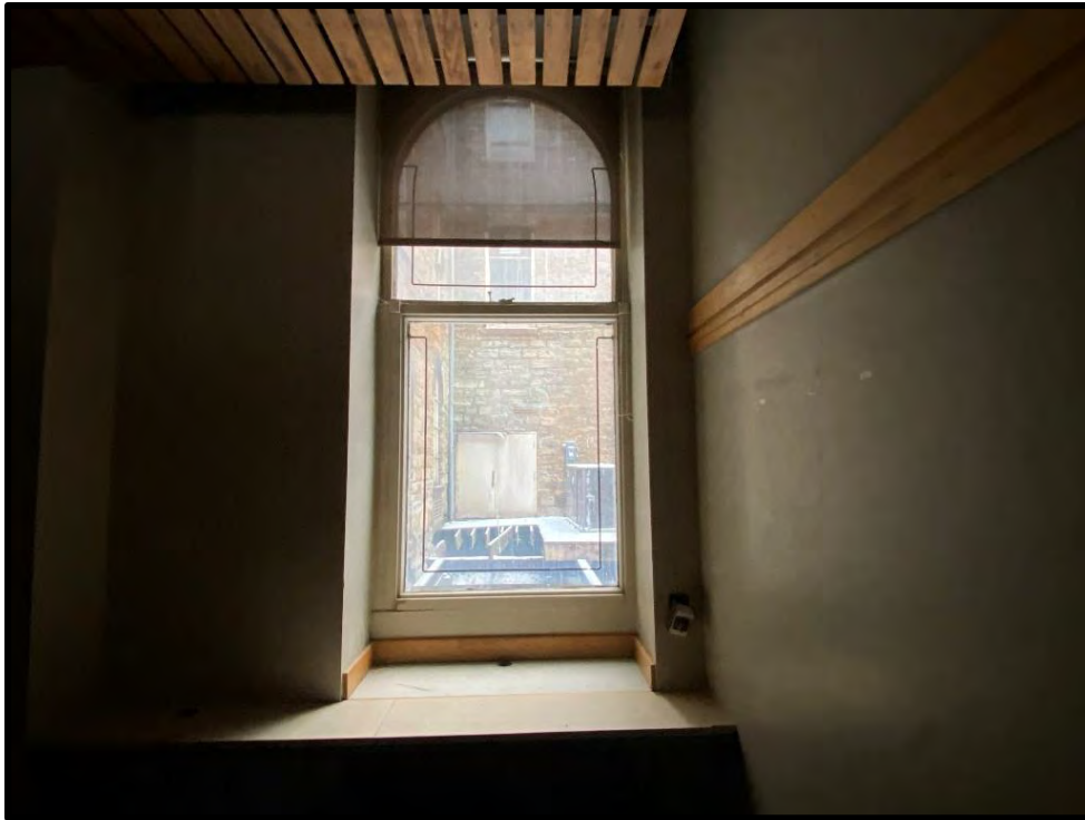
Image 67: First Floor – Interior (Measurements taken on December 8, 2021; Facing East)
