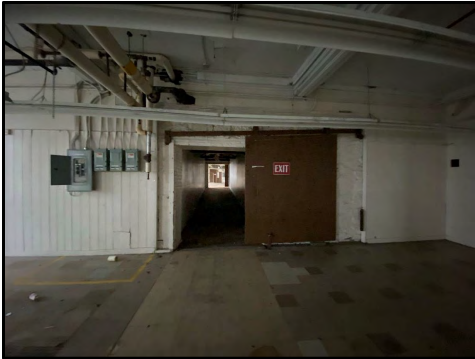
Image 109: Second Floor Stone Building – Walkway to Brick Building (Photo taken on December 8, 2021; Facing West)
