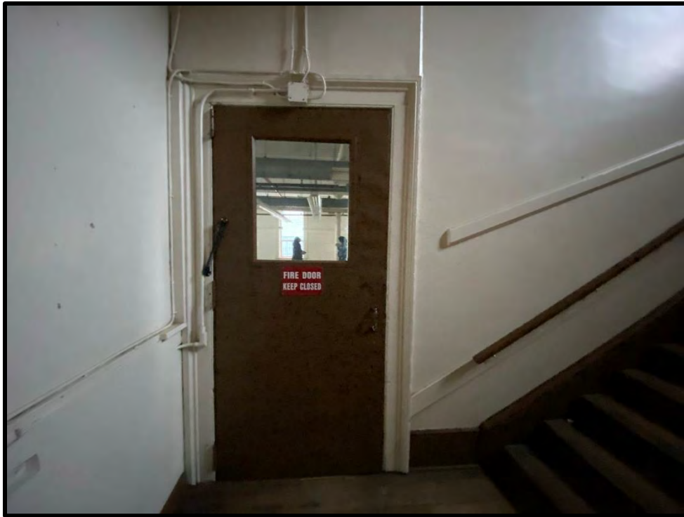
Image 101: Second Floor Stone Building – Interior (Photo taken on December 8, 2021)
