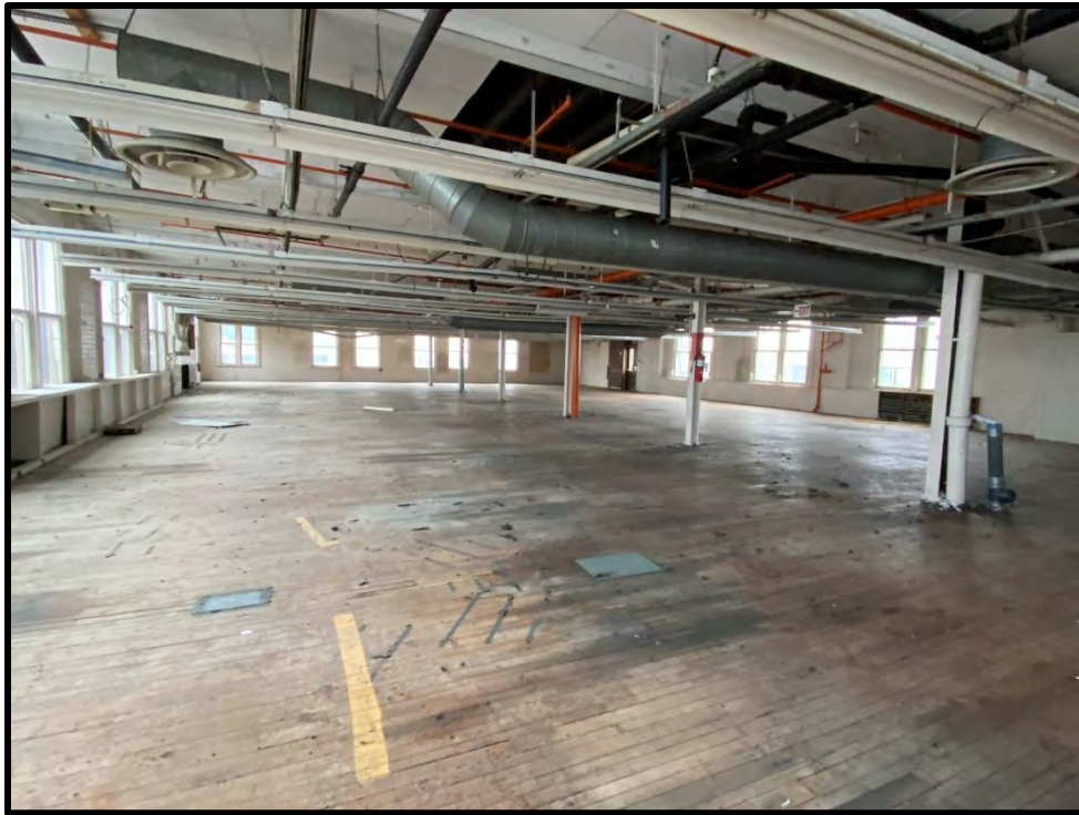
Image 175: Third Floor Brick Building – Interior (Photo taken on December 8, 2021; Facing South)
