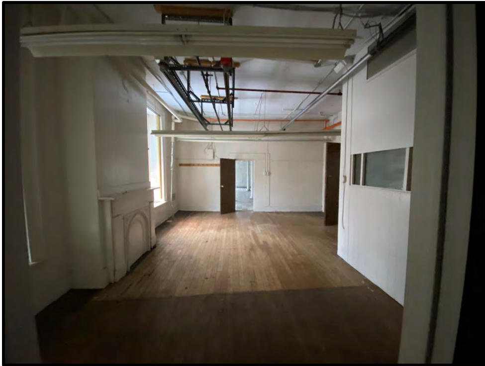
Image 103: Second Floor Stone Building – Interior (Photo taken on December 8, 2021; Facing South)
