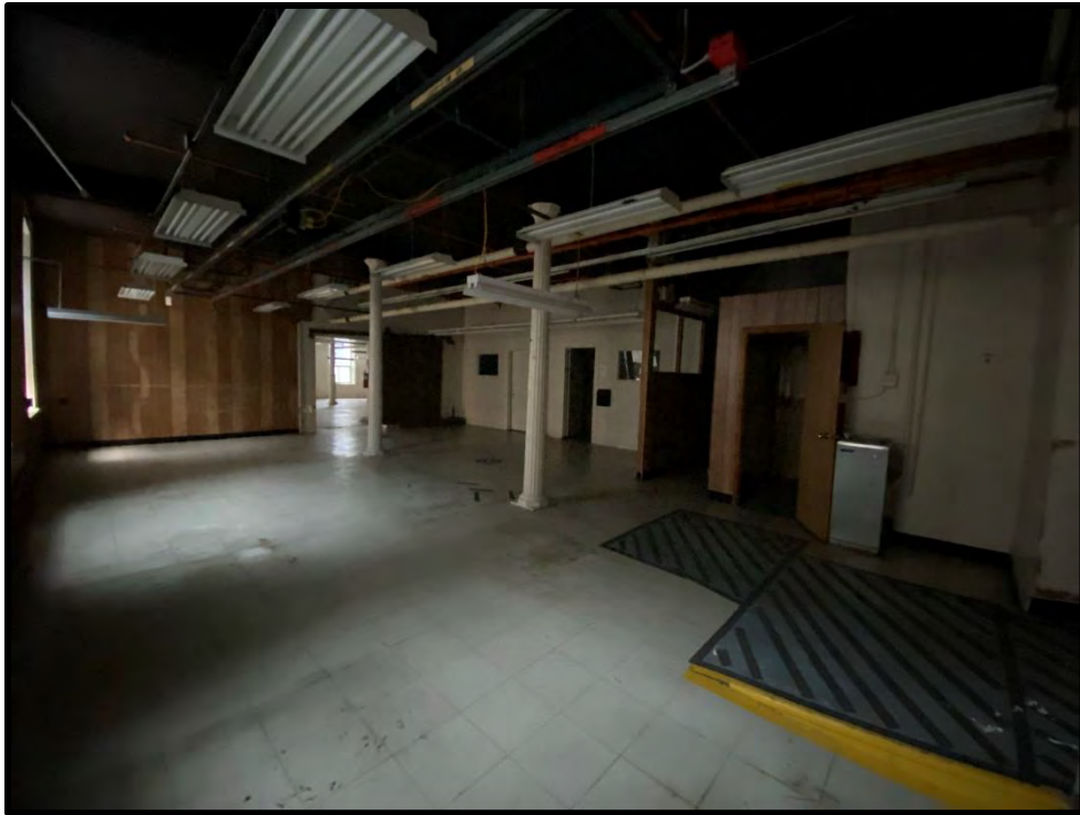
Image 111: Second Floor Stone Building – Interior (Photo taken on December 8, 2021; Facing Southwest)
