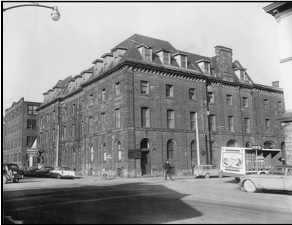
Plate 11: Stone Building at 56 York Boulevard (HPL LHA no date)
