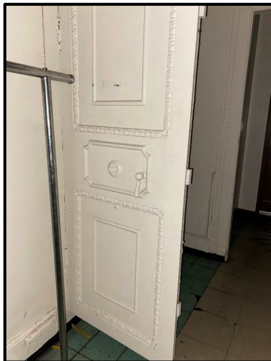
Image 122: Second Floor North Addition – Vault (Photo taken on December 8, 2021)
