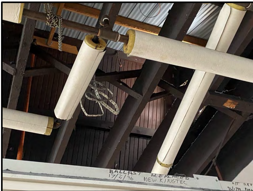
Image 176: Third Floor Brick Building – Ceiling Detail (Photo taken on December 8, 2021)
