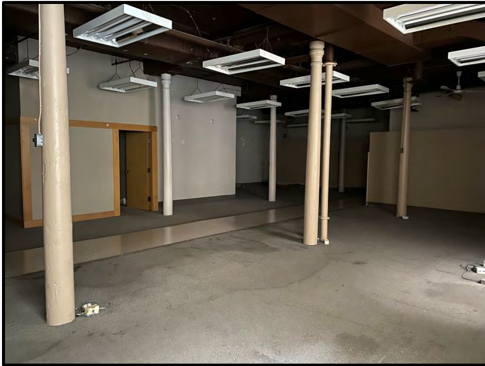
Image 79: First Floor North Addition – Interior (Photo taken on December 8, 2021; Facing Northeast)
