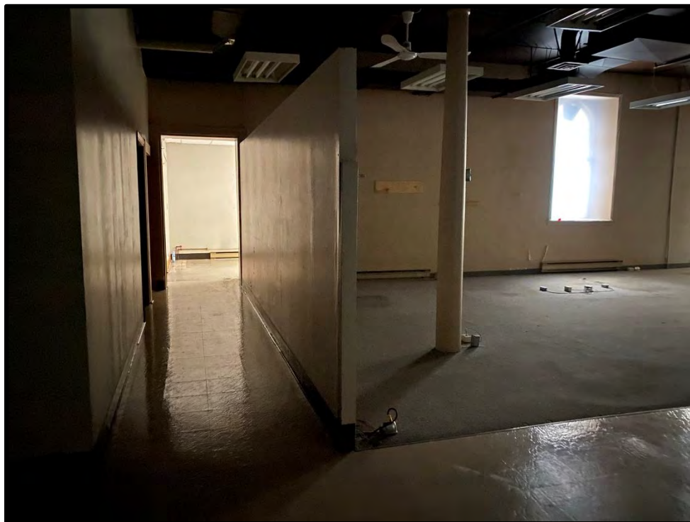
Image 84: First Floor North Addition – Interior (Photo taken on December 8, 2021; Facing South)
