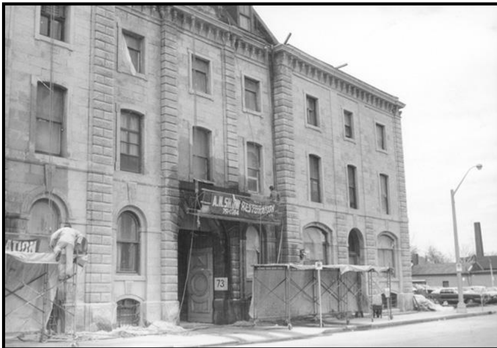
Plate 16: Restoration in Progress at 63-73 MacNab Street (HPL LHA 1978)
