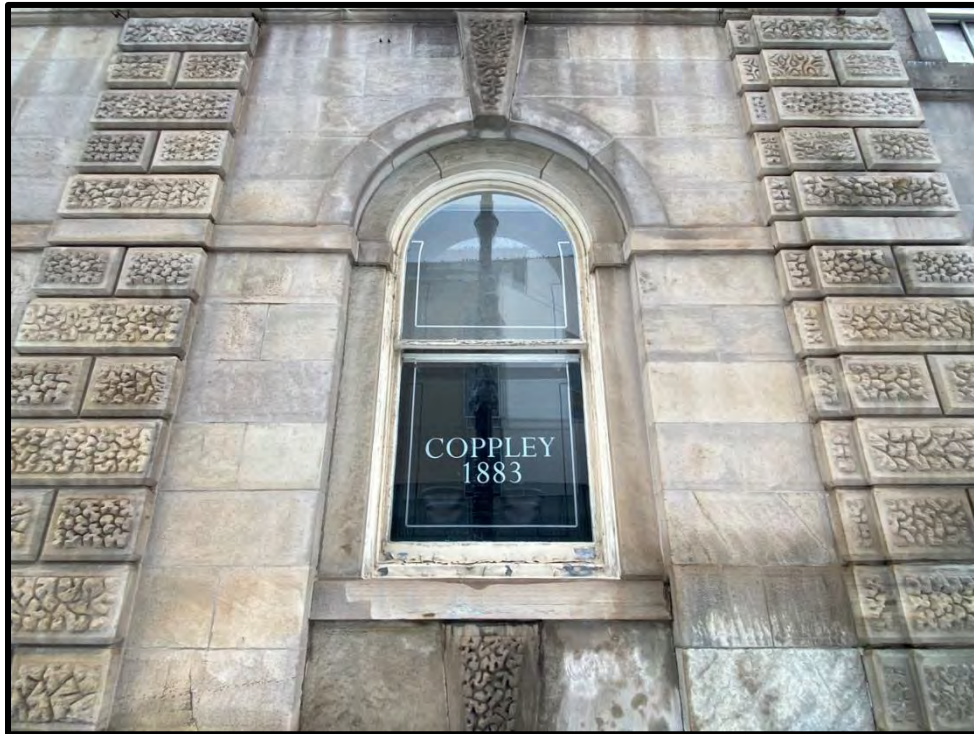
Image 7: First Storey Window Opening and Vermiculated Ashlar Pilasters – Detail (Photo taken on December 8, 2021; Facing North)
