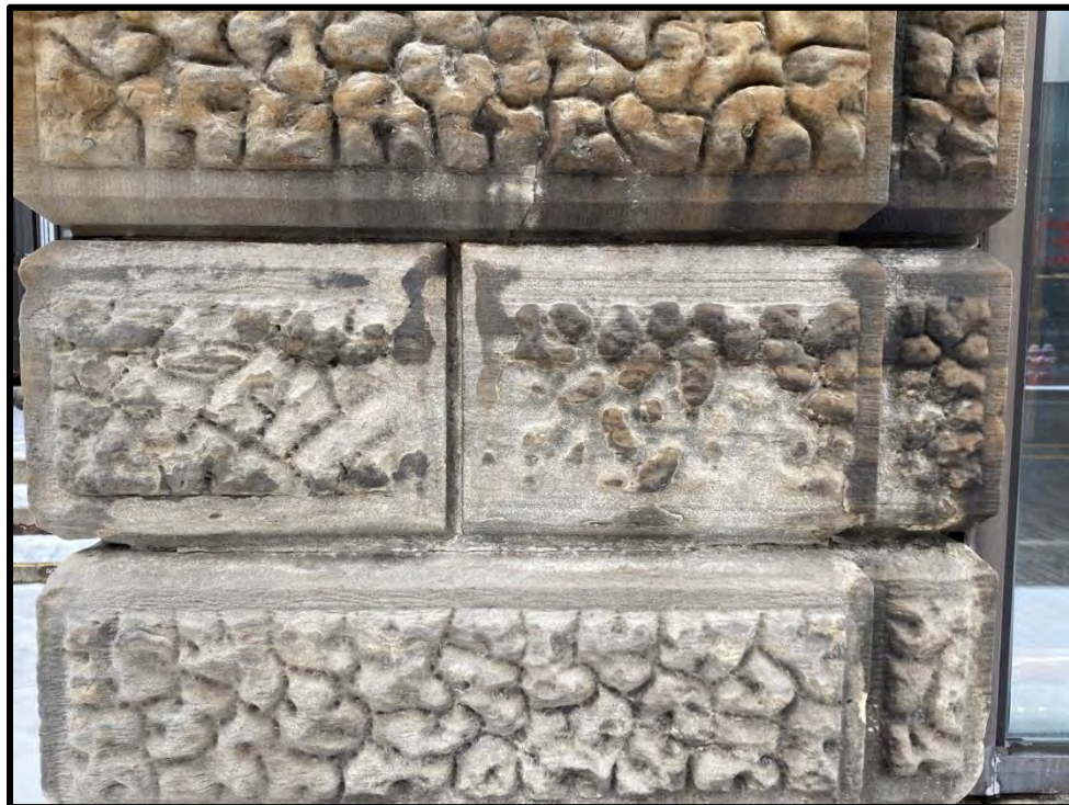
Image 6: Vermiculated Stone Pilaster – Detail (Photo taken on December 8, 2021; Facing North)
