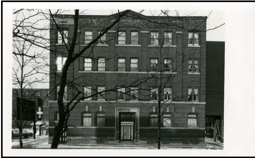
Plate 19: Brick Building at 56 York Boulevard, no date (Provided by the City of Hamilton)
