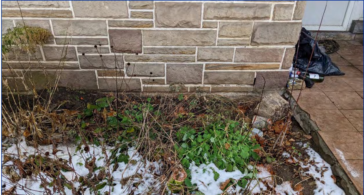
Figure 16: View of the residence's concrete foundation
