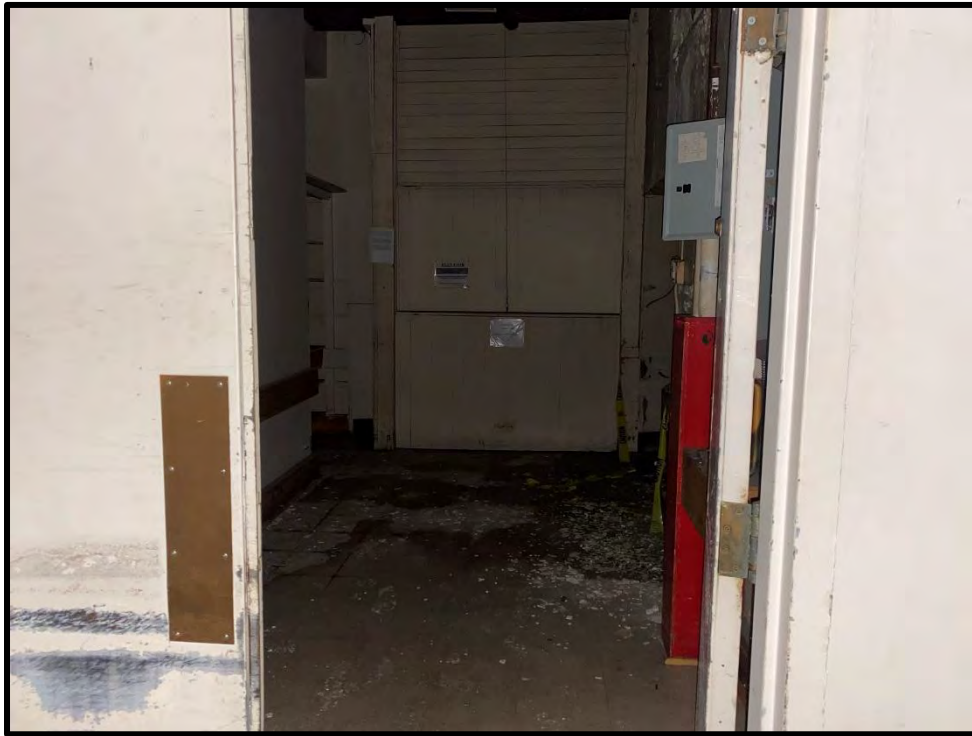
Image 77: First Floor North Addition – Interior (Photo taken on December 8, 2021; Facing North)
