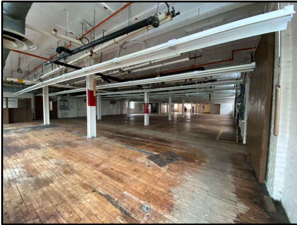
Image 169: Second Floor Brick Building – Interior (Photo taken on December 8, 2021; Facing Northeast)
