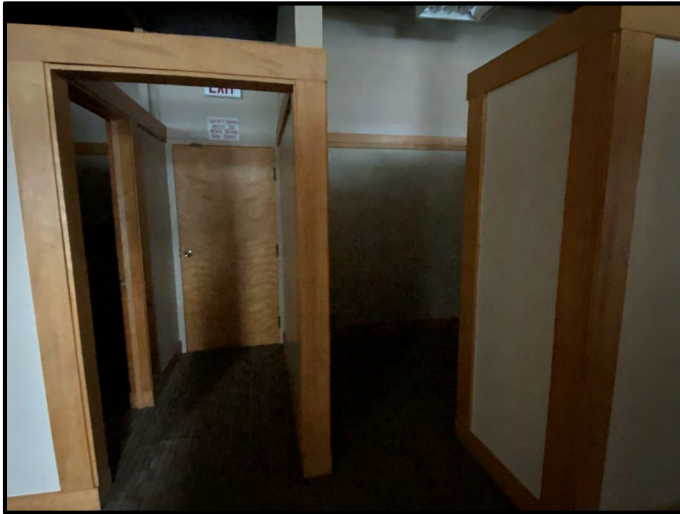
Image 65: First Floor – Interior (Photo taken on December 8, 2021; Facing North)
