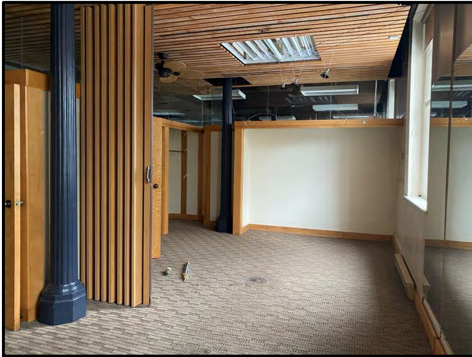
Image 59: First Floor – Interior (Photo taken on December 8, 2021; Facing Northeast)
