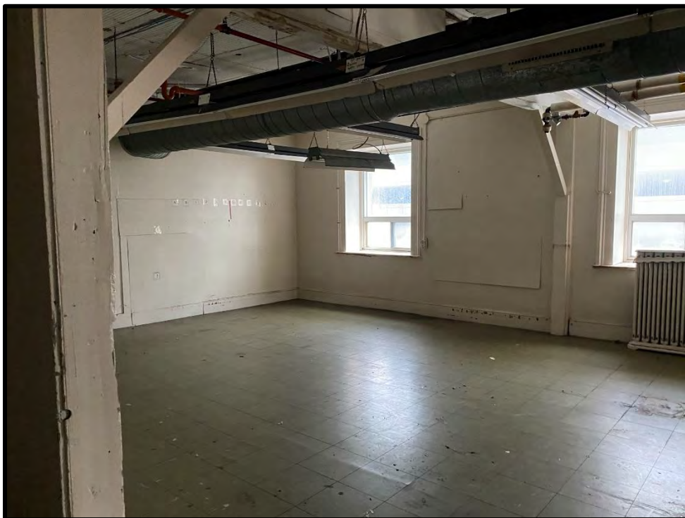
Image 124: Third Floor Stone Building – Interior (Photo taken on December 8, 2021; Facing Northeast)
