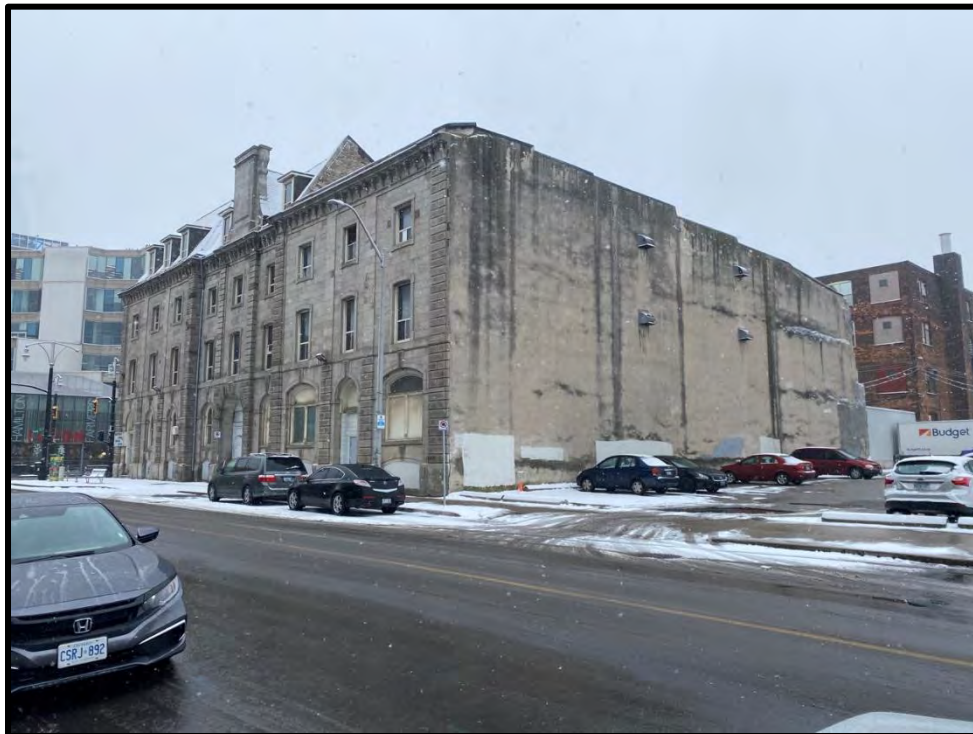
Image 20: North and East Elevations (Photo taken on December 8, 2021; Facing Southwest)
