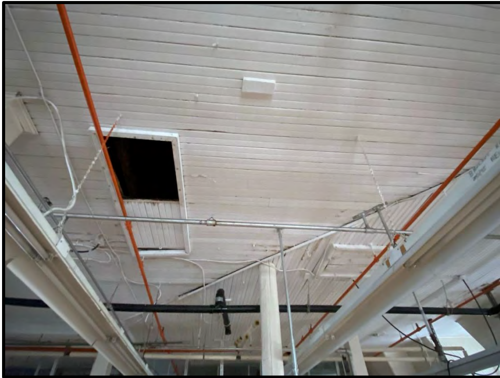
Image 139: Fourth Floor Stone Building – Ceiling (Photo taken on December 8, 2021)
