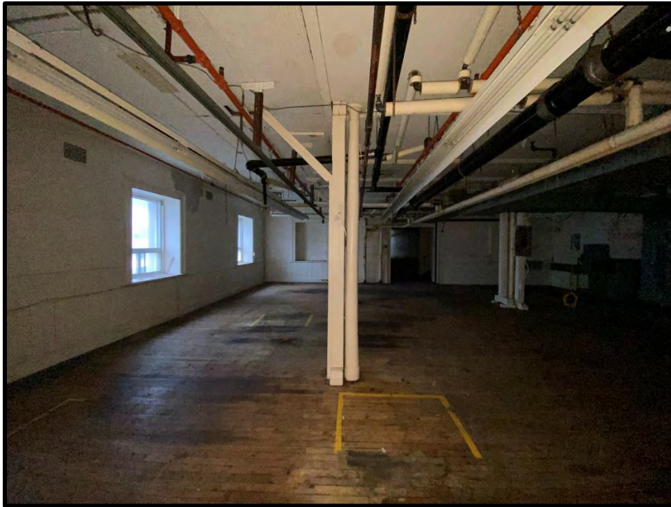
Image 131: Third Floor – Interior (Photo taken on December 8, 2021; Facing West)
