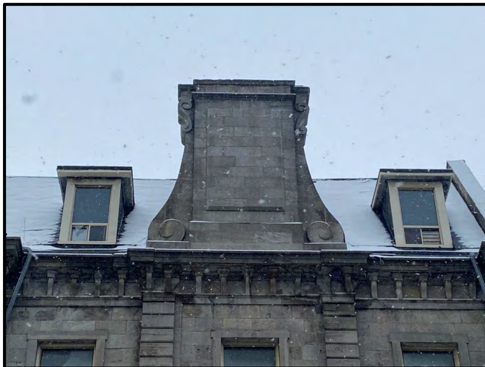
Image 24: East Elevation Chimney, Brackets and Dormers Detail (Photo taken on December 8, 2021; Facing West)
