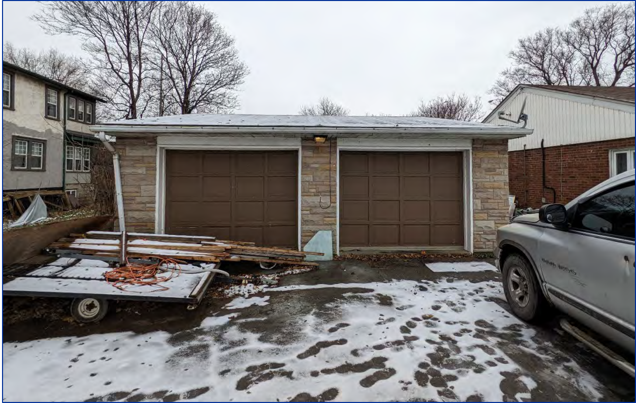
Figure 21: View of the east elevation of the detached garage
