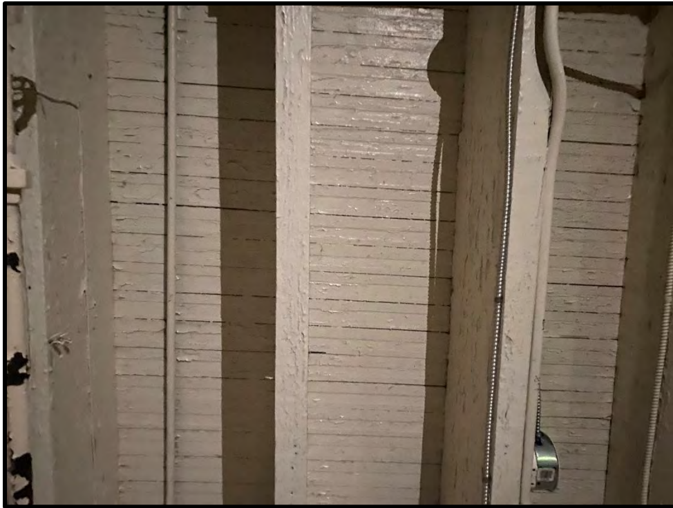
Image 179: Basement Brick Building – Ceiling (Photo taken on December 8, 2021)
