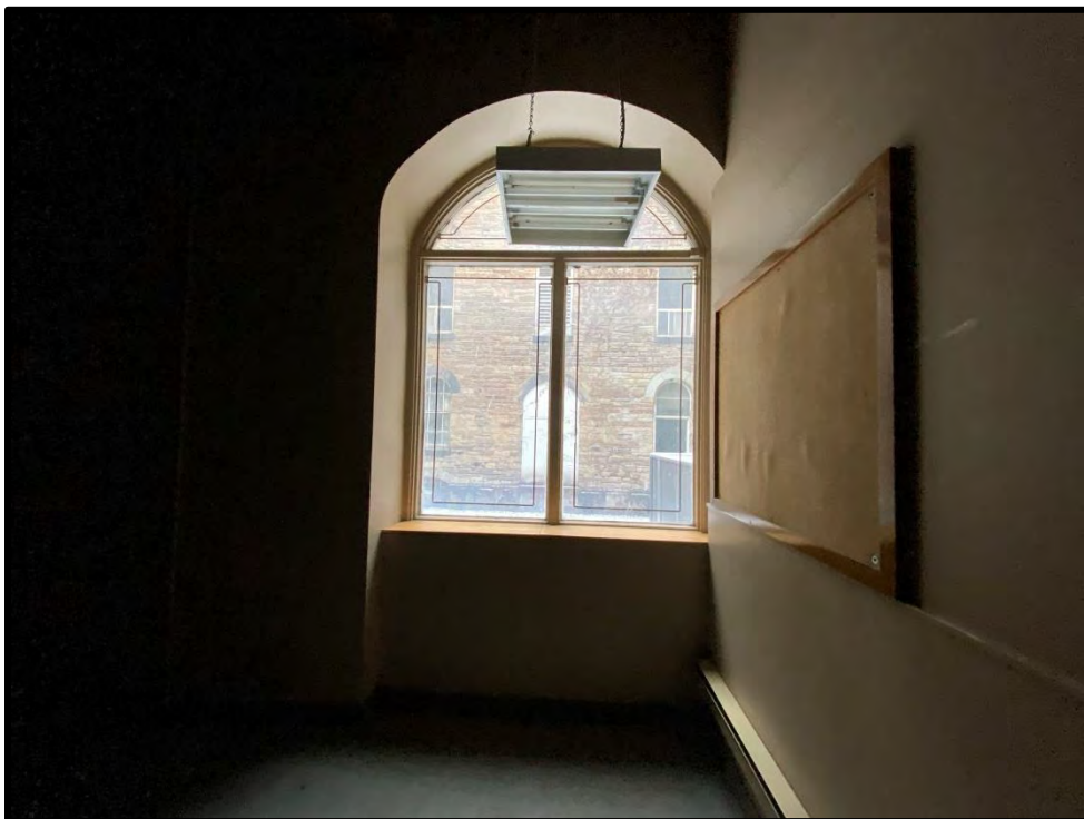
Image 88: First Floor North Addition – Interior (Photo taken on December 8, 2021; Facing South)
