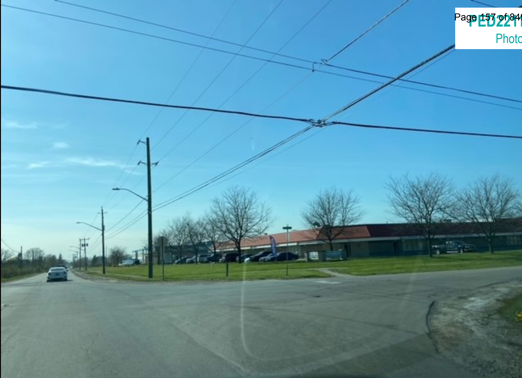
Employment uses on north side of Barton Street at Glover Road
