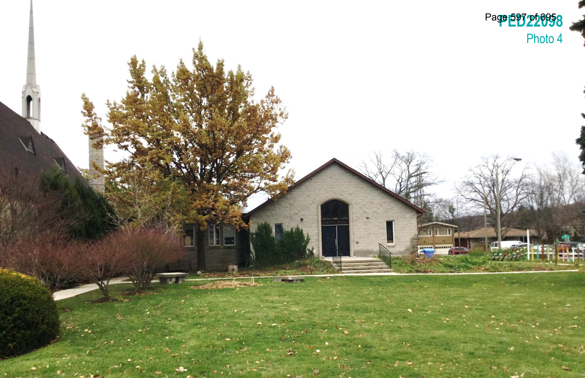
Existing Place of Worship at 1107 Main Street West, as seen from Cline Avenue South looking east
