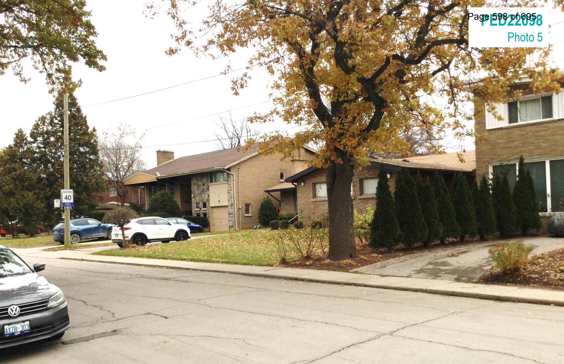
Properties at 9, 15 and 19 Dow Avenue located to the east of the subject property, as seen from Dow Avenue looking north east
