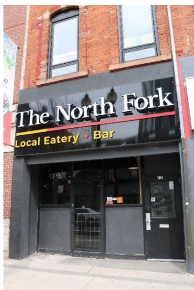
215 King Street East, Hamilton (Source: CDSB staff)
