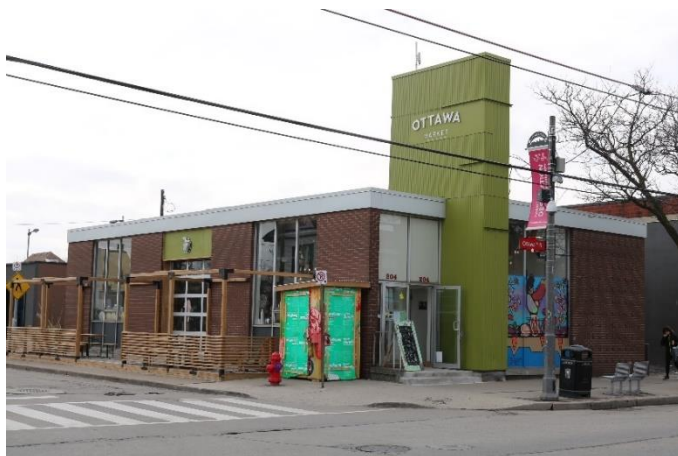
204 Ottawa Street North, Hamilton (Source: CDSB Staff)
