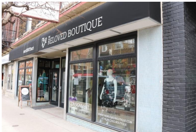
226-228 James Street North, Hamilton (Source: CDSB staff)
