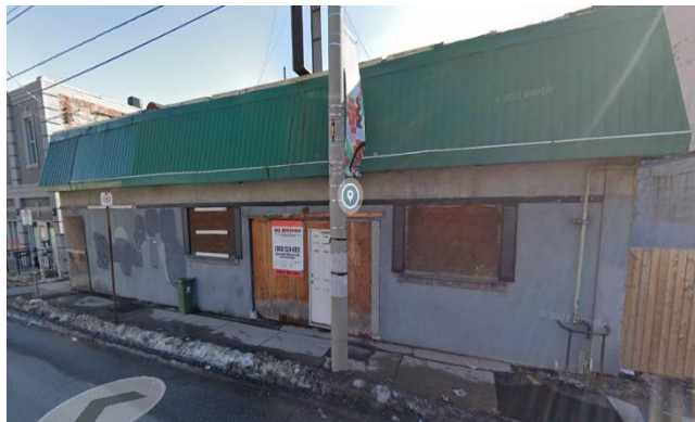
440 Barton Street East-Before Renovations (Source: Google Street View)
