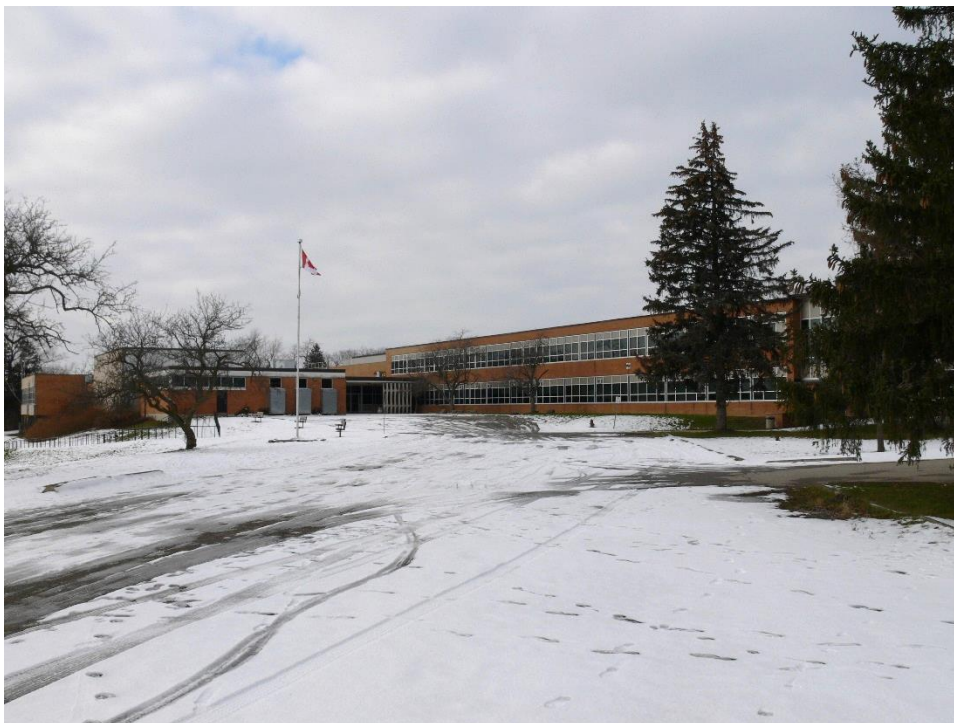
Plate 11: Looking northwest along the drive that accesses the south elevation of the East Wing.
