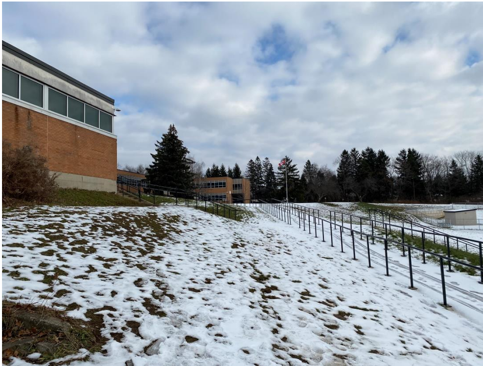
Plate 1: Looking east towards the south elevation of the East Wing (left) and running track in the athletic field (right)
