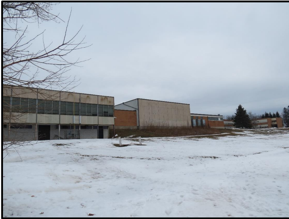
Image 21: South Elevation of East Wing addition (Photo taken on March 13, 2019; Facing Northeast)
