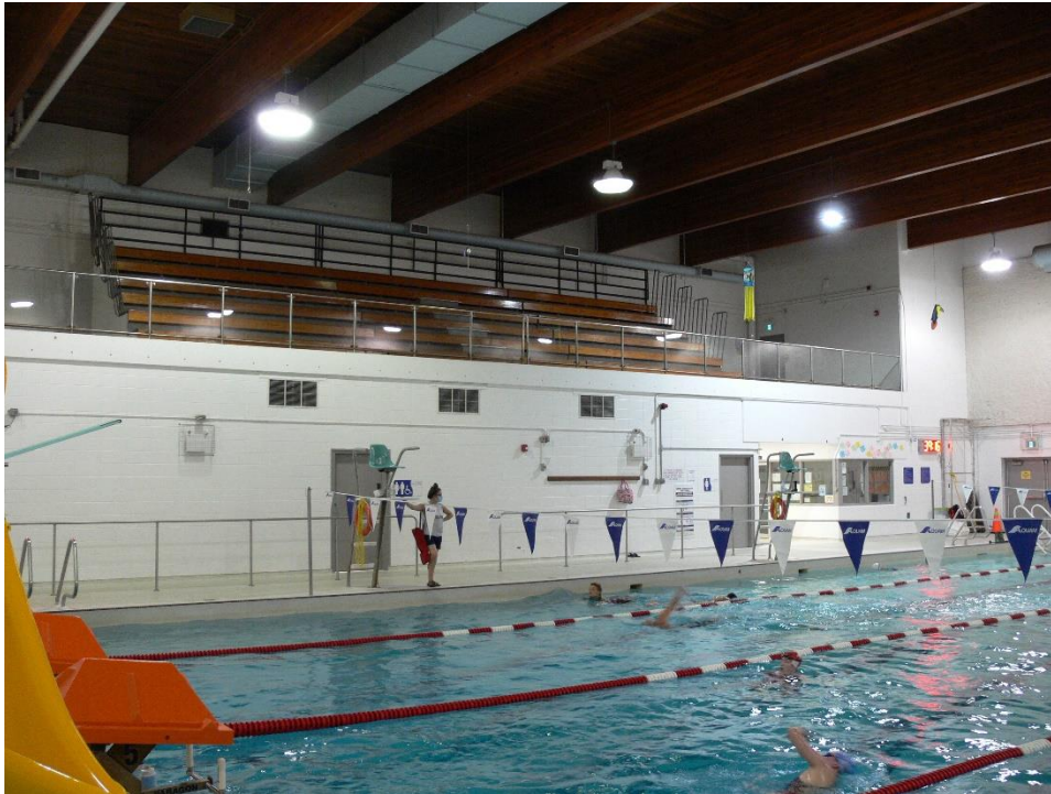
Plate 46: Main pool room and observation deck
