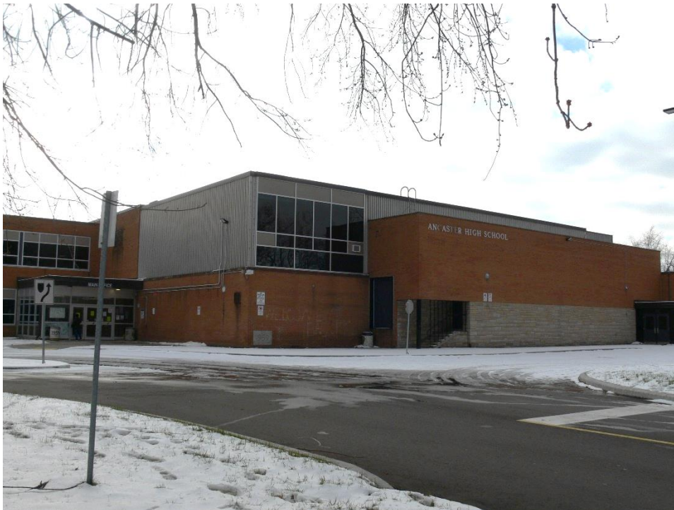
Plate 27: 1959 school building with 1964 roof addition
