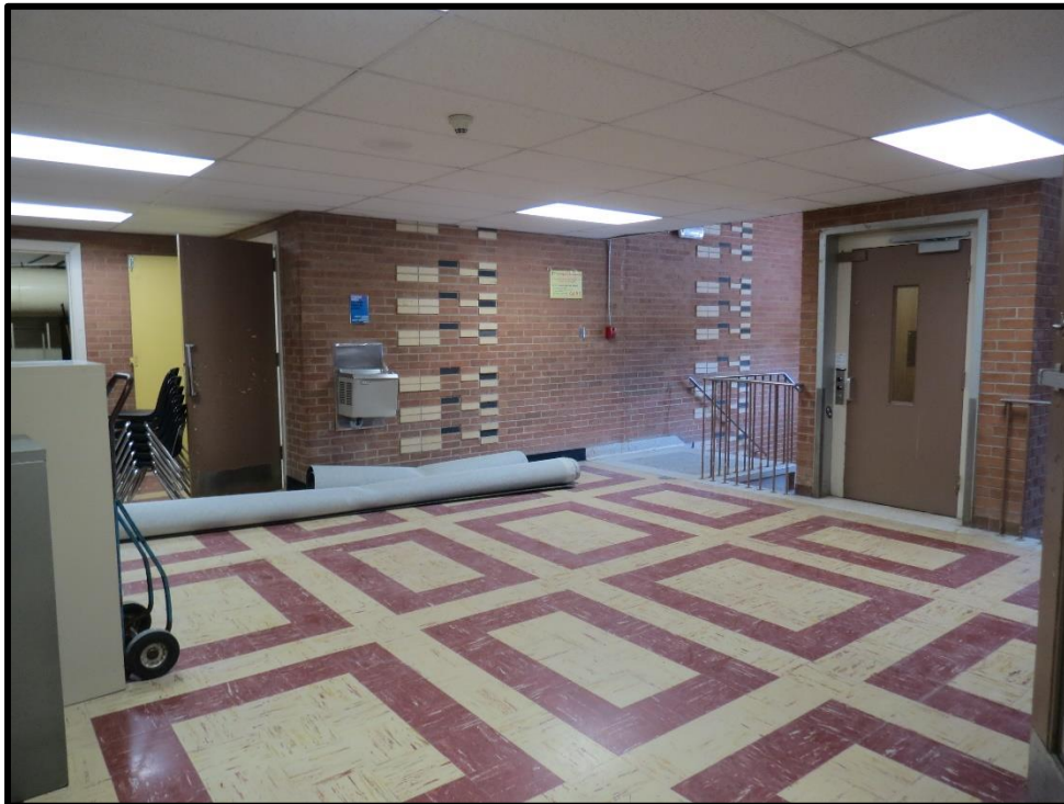
Image 48: Second Floor Foyer - West Wing (Photo taken on March 13, 2019)
