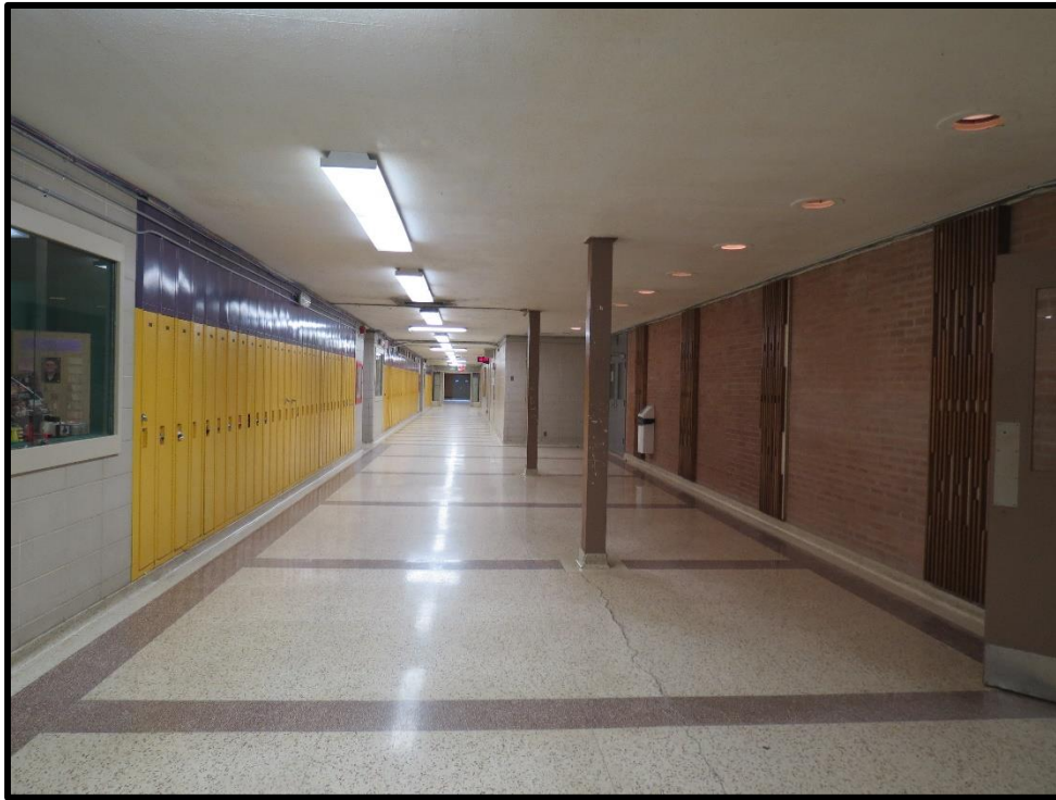
Image 53: View of Hall with labs/shops - West Wing (Photo taken on March 13, 2019)
