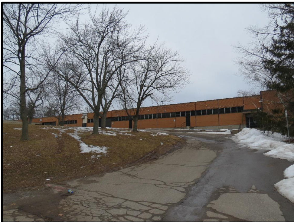
Image 20: West Elevation of East Wing (Photo taken on March 13, 2019; Facing Northeast)
