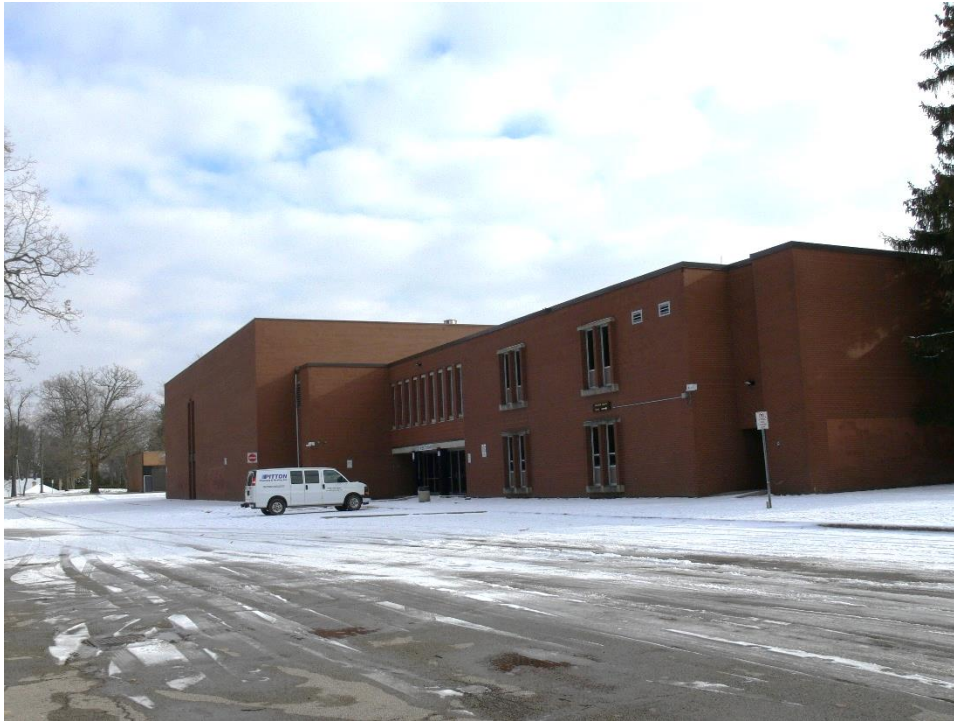
Plate 29: North elevation of the West Wing
