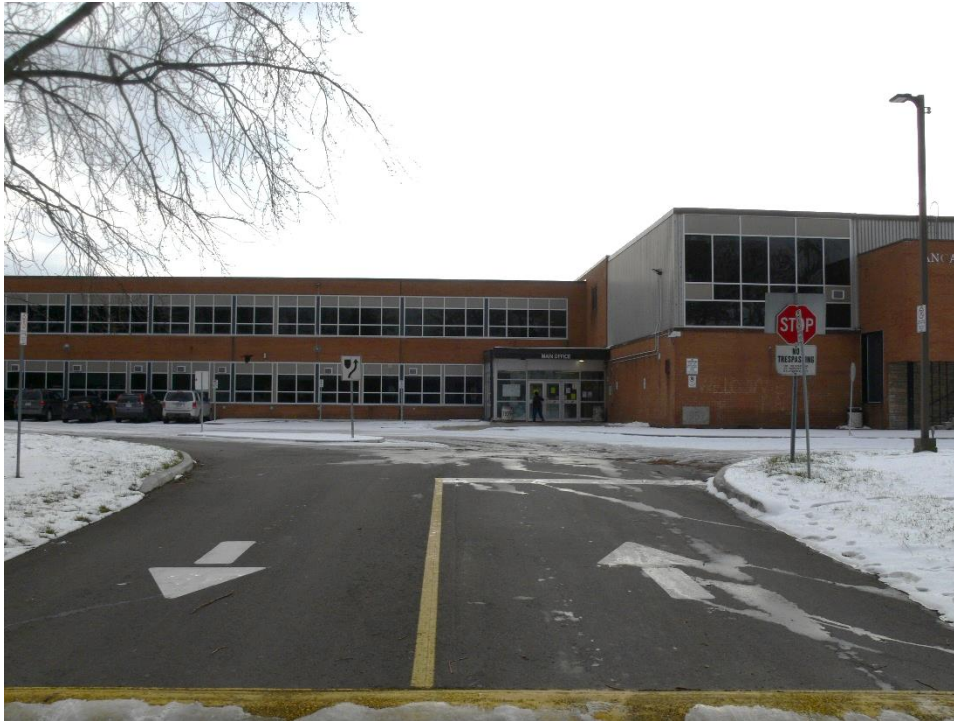
Plate 26: North elevation and main entrance of the East Wing
