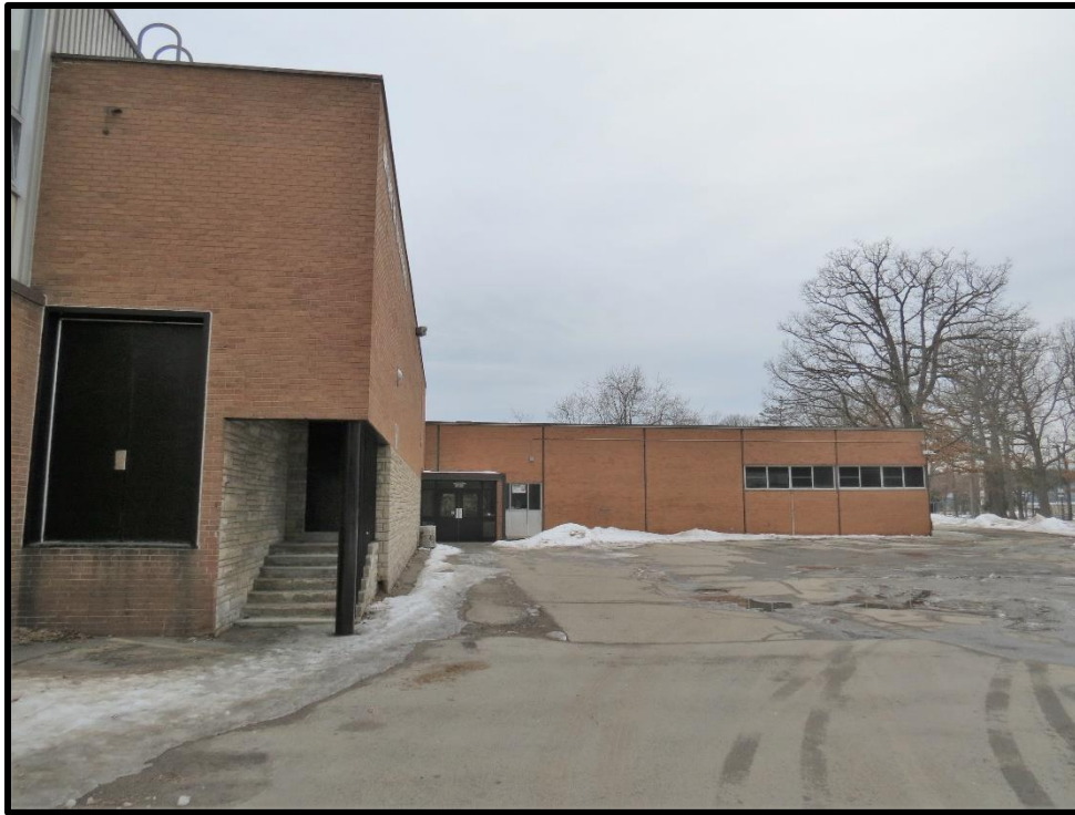
Image 8: Detail of Secondary Entryways of Façade (Photo taken on March 13, 2019; Facing West)
