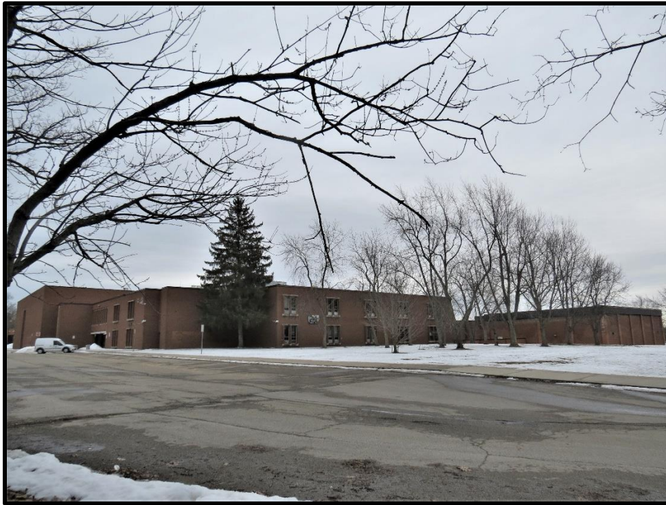
Image 14: Northwest corner of Ancaster High School (Photo taken on March 13, 2019; Facing Southeast)
