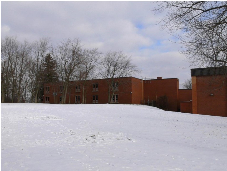
Plate 30: West elevation of the West Wing
