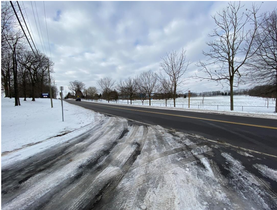
Plate 50: Looking northwest on Jerseyville Road West towards the Robert E. Wade Ancaster Community Park
