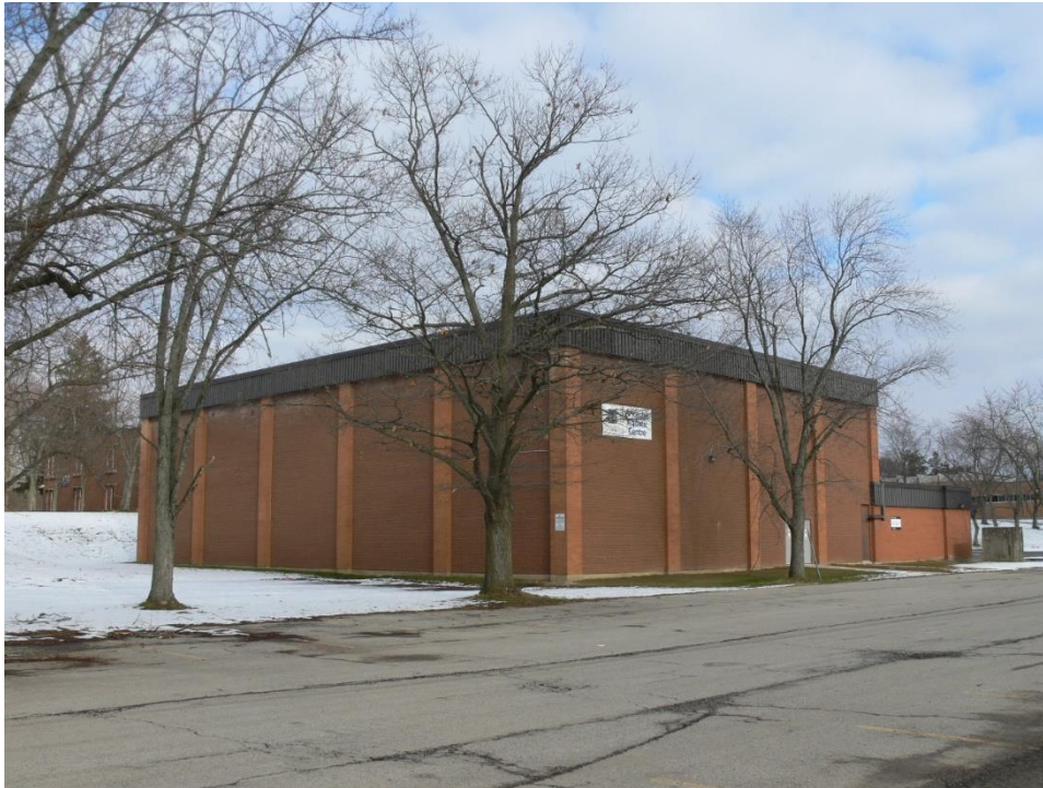
Plate 32: West and south elevations of the main pool building of the Ancaster Aquatic Centre
