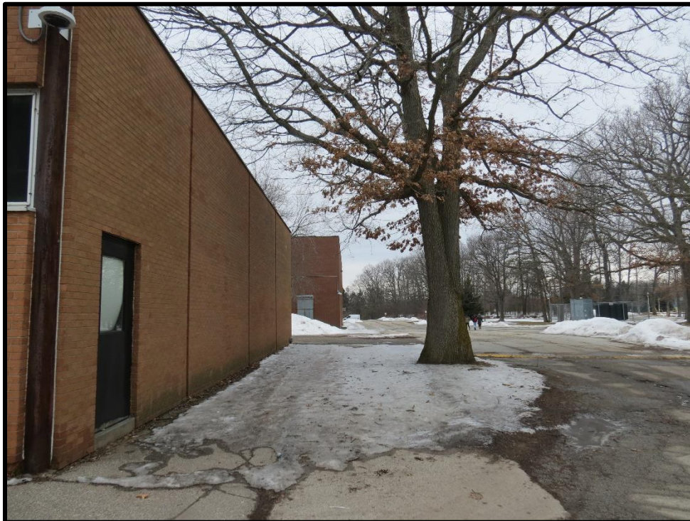
Image 9: North Elevation of West Wing (Photo taken on March 13, 2019; Facing West)
