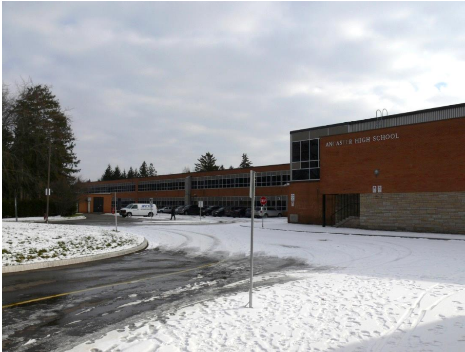
Plate 14: Looking southeast towards the north elevation of the East Wing and parking lot
