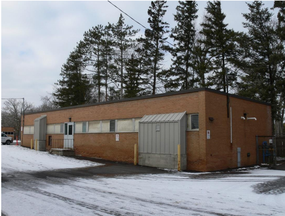
Plate 34: South and east elevations of the 1959 utility building
