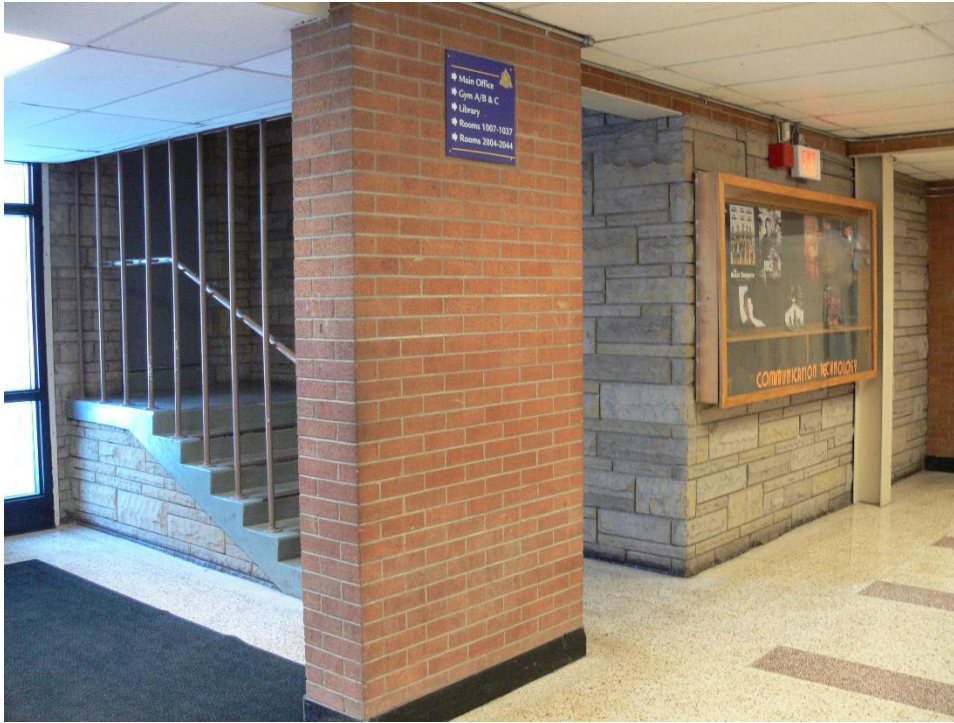
Plate 39: Enclosed portion of the original 1959 school building
