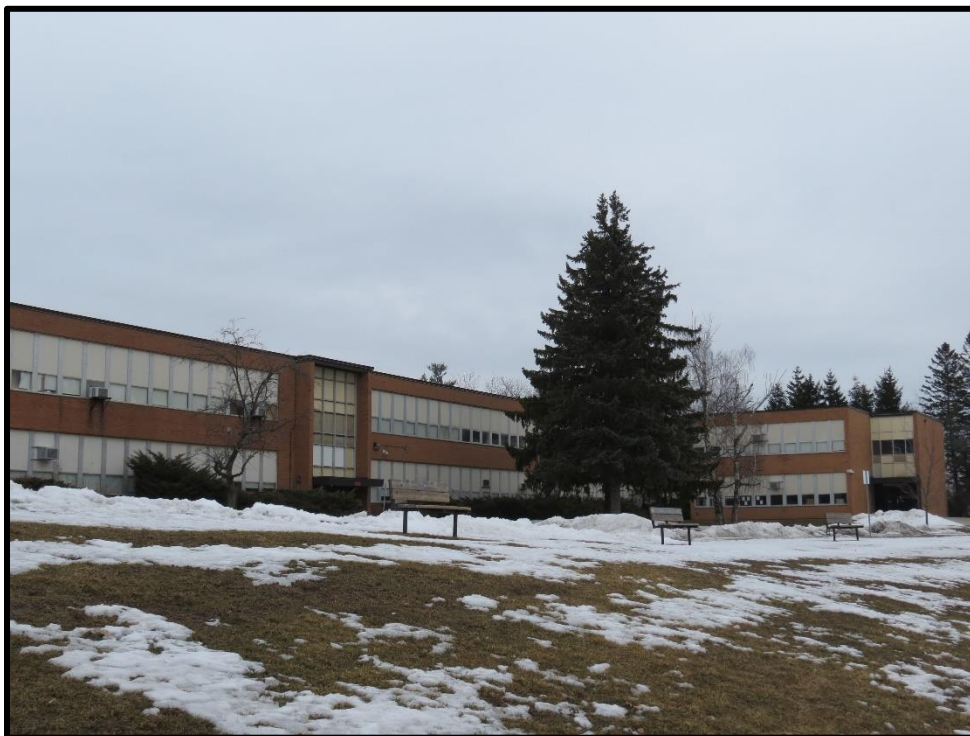
Image 22: South Elevation of East Wing – Original portion and 1960-1961 addition (Photo taken on March 13, 2019; Facing Northeast)
