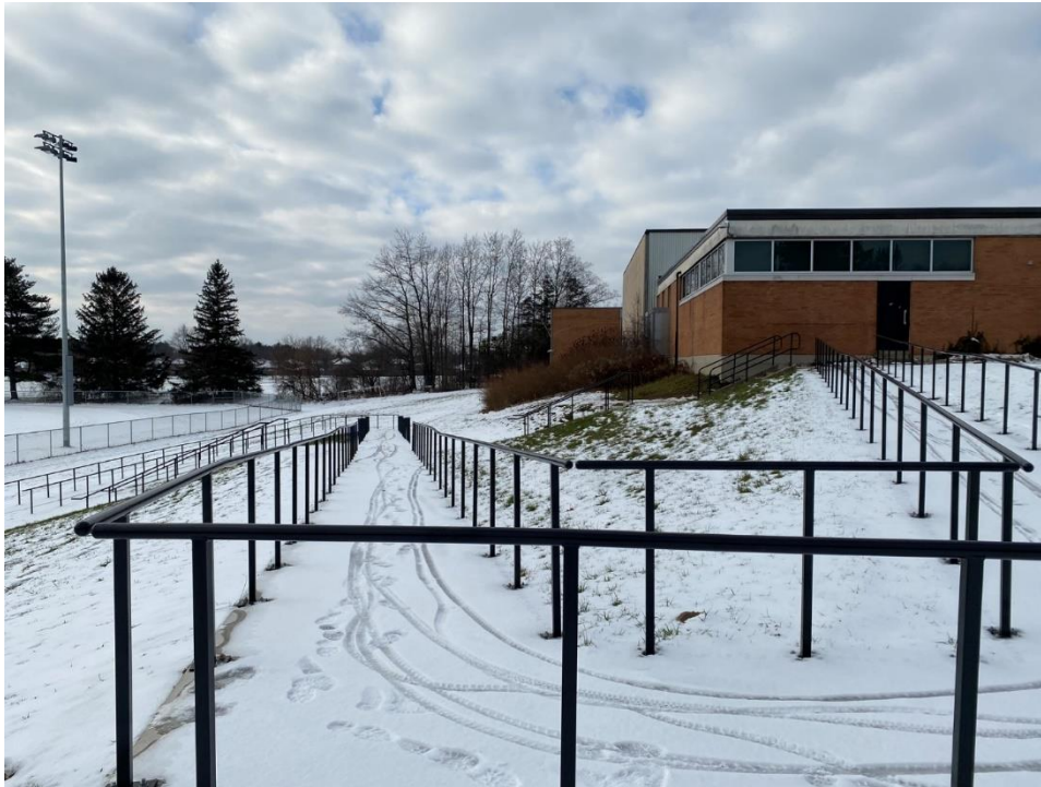
Plate 18: Looking west towards pedestrian ramp to the athletic fields that weaves down the slope in the topography south of the school building
