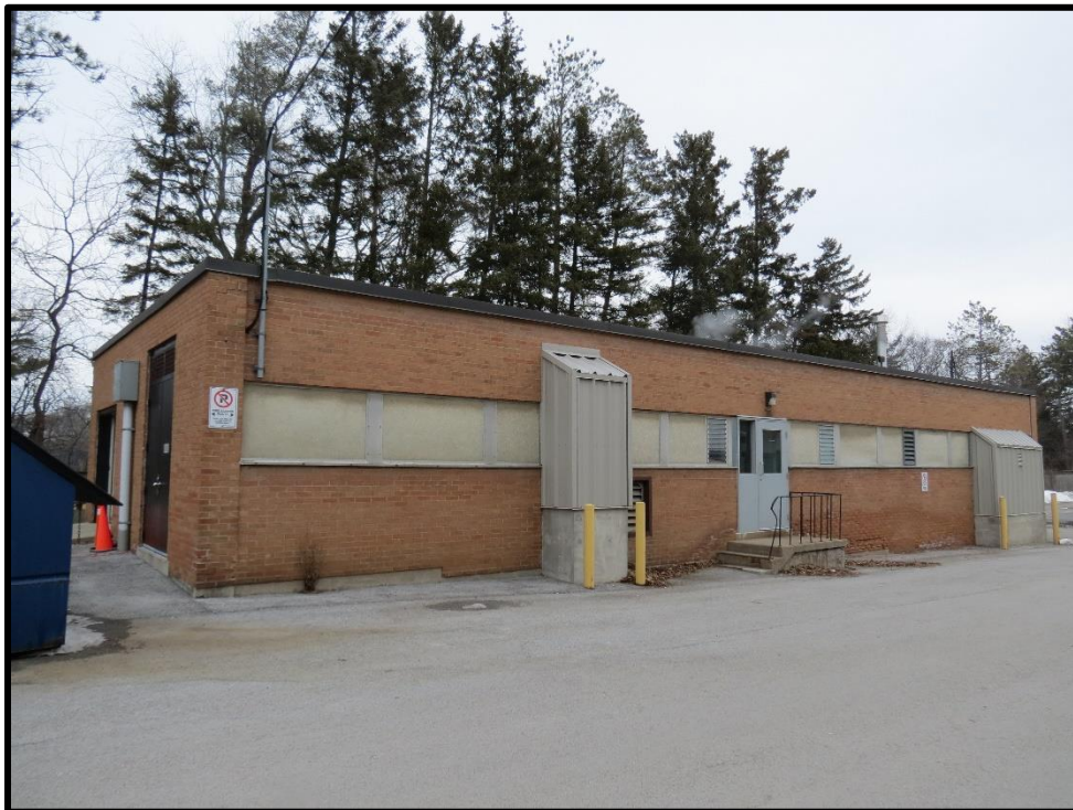
Image 7: Boiler/Garage structure in North (Photo taken on March 13, 2019; Facing Northeast)
