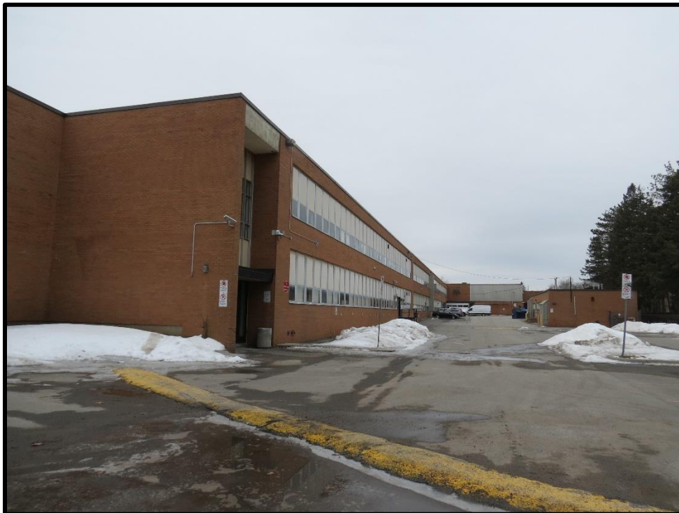
Image 5: View of East Wing façade – Ancaster High School (Photo taken on March 13, 2019; Facing West)
