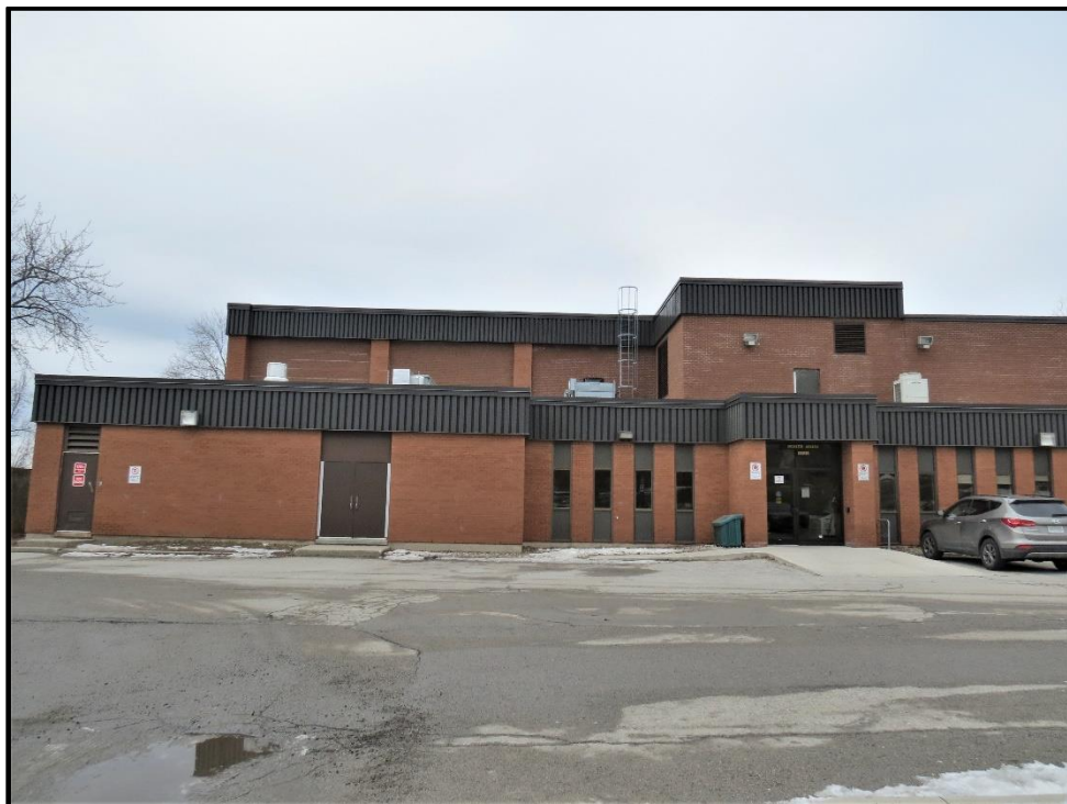
Image 18: East elevation of Aquatic Centre (Photo taken on March 13, 2019; Facing West)
