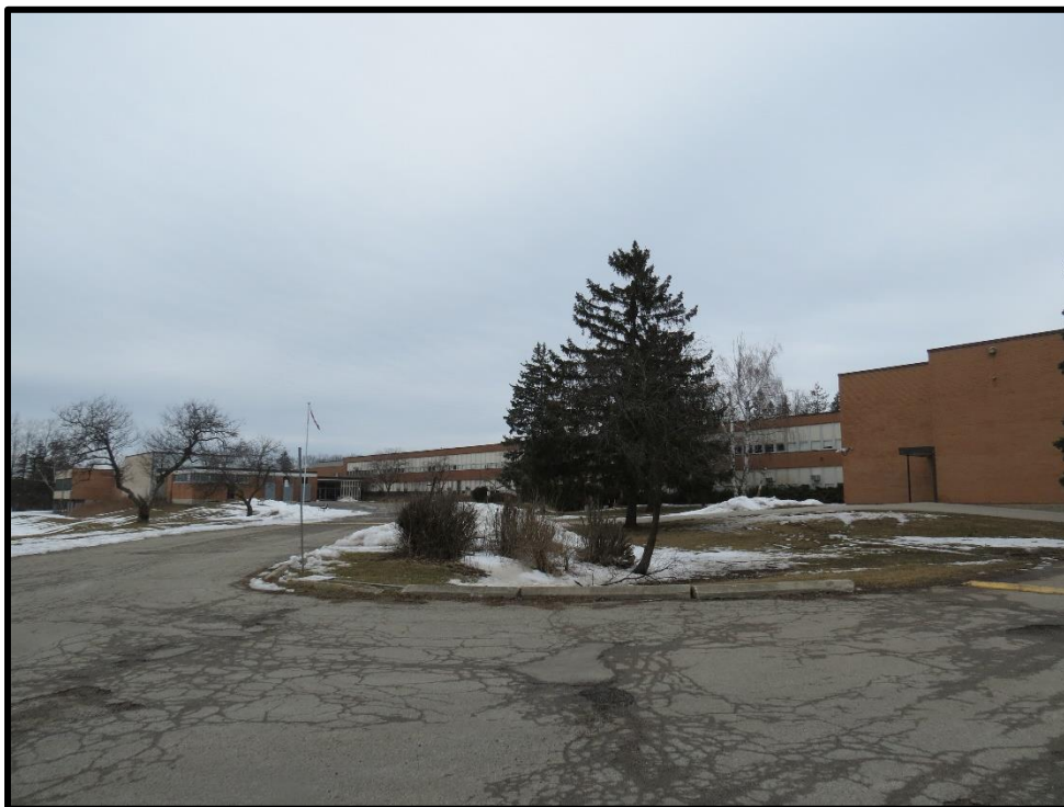
Image 24: West Elevation of Addition (Photo taken on March 13, 2019; Facing West)
