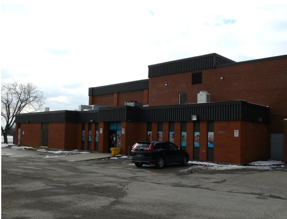
Plate 33: Entrance to the Ancaster Aquatic Centre
