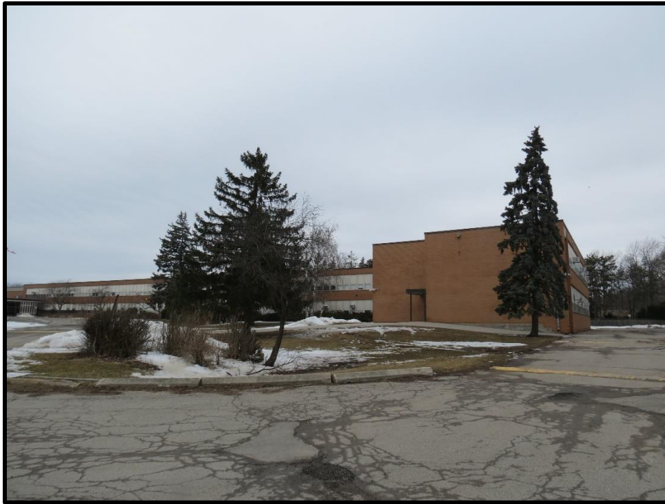
Image 23: South Elevation and Southeast corner of East Wing – Original portion and 1960-1961 addition (Photo taken on March 13, 2019; Facing Northwest)
