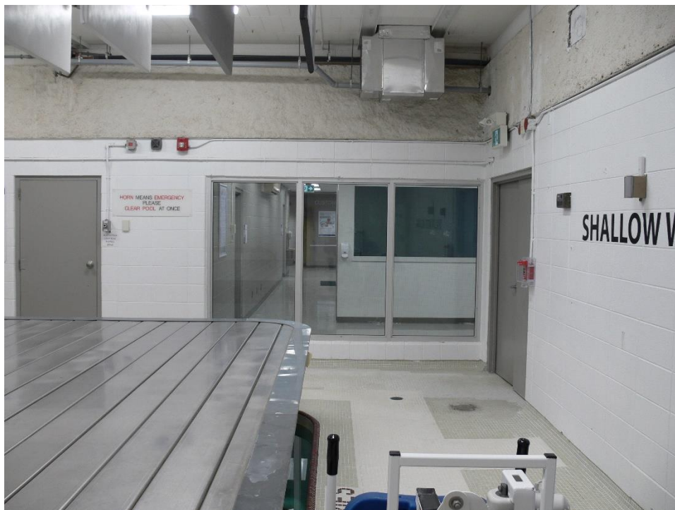
Plate 47: Smaller pool room with interior windows to the corridors
