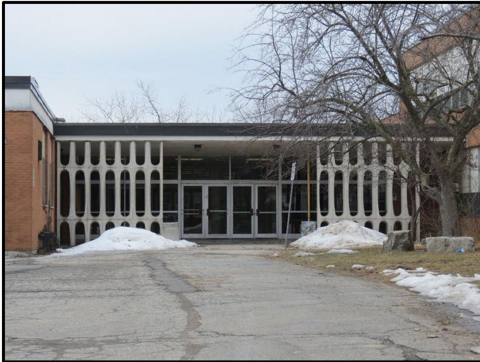
Image 25: Detail of entryway – West Elevation of Addition (Photo taken on March 13, 2019; Facing West)
