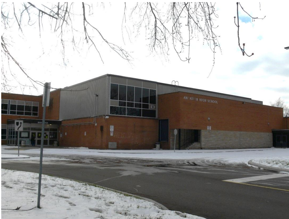
Plate 27: 1959 school building with 1964 roof addition
