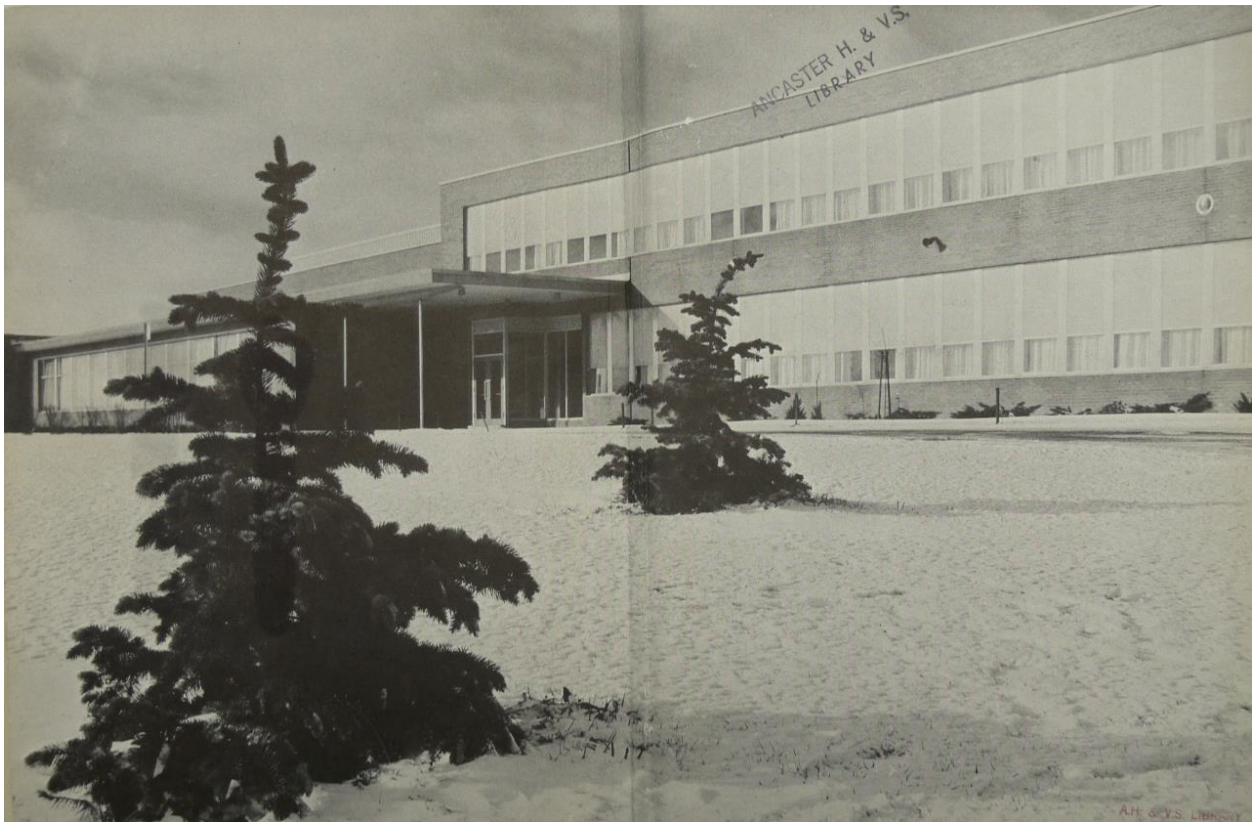
Figure 10: South entrance to Ancaster High School in 1962, prior to later additions that would reconfigure the entryway (1962 Quest Yearbook, Hamilton-Wentworth District School Board Educational Archives)
