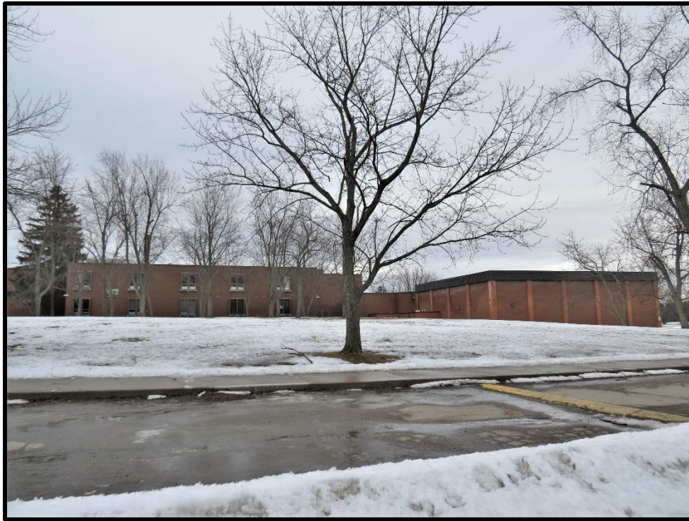
Image 15: West Elevation of Ancaster High School and Aquatic Centre (Photo taken on March 13, 2019; Facing East)
