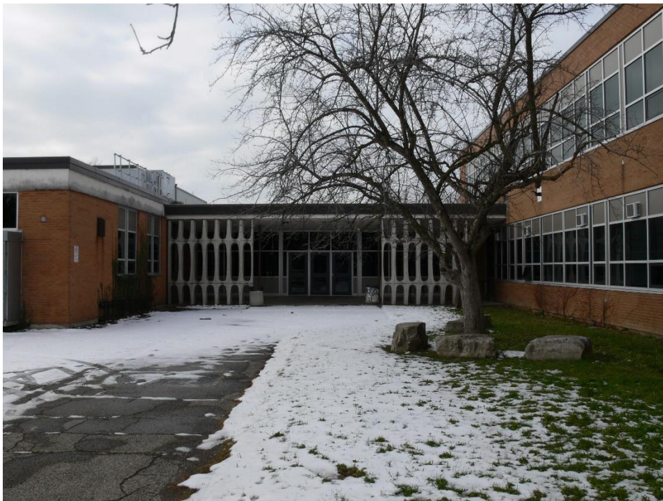
Plate 23: Detail of the reconfigured entrance with concrete screen
