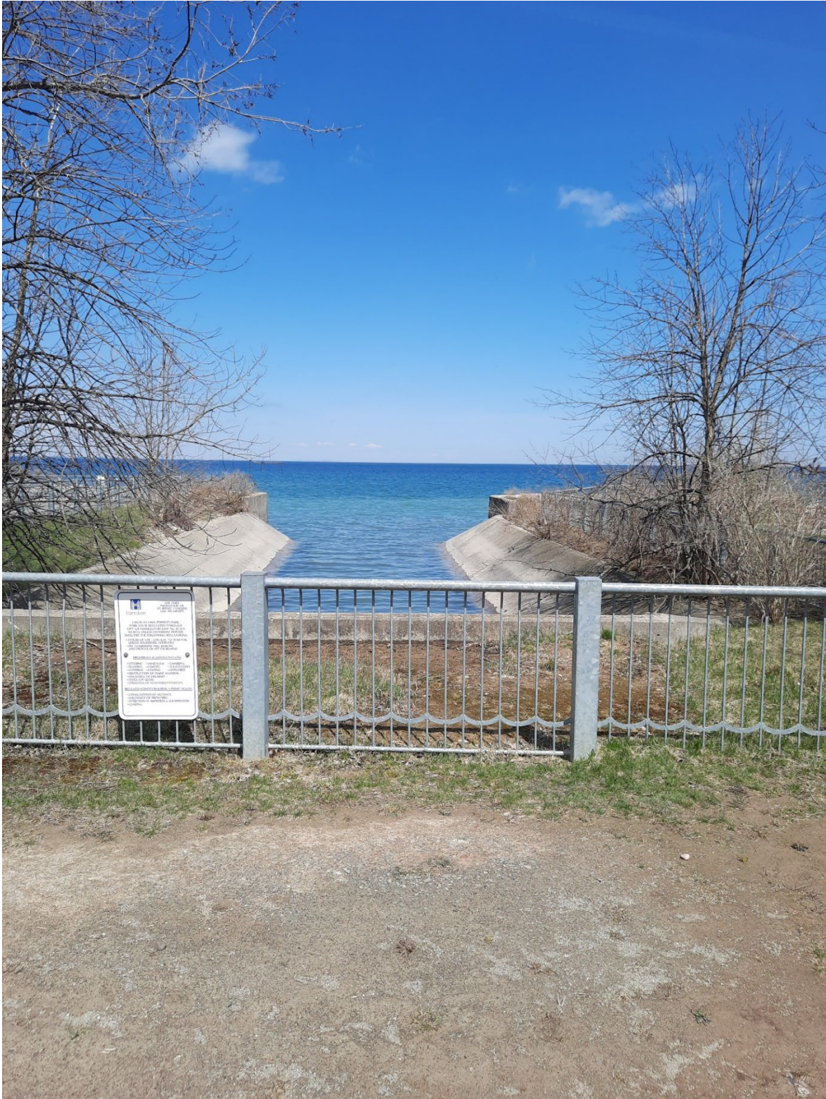
(Facing North, Lake Ontario Storm Water Outfall)
