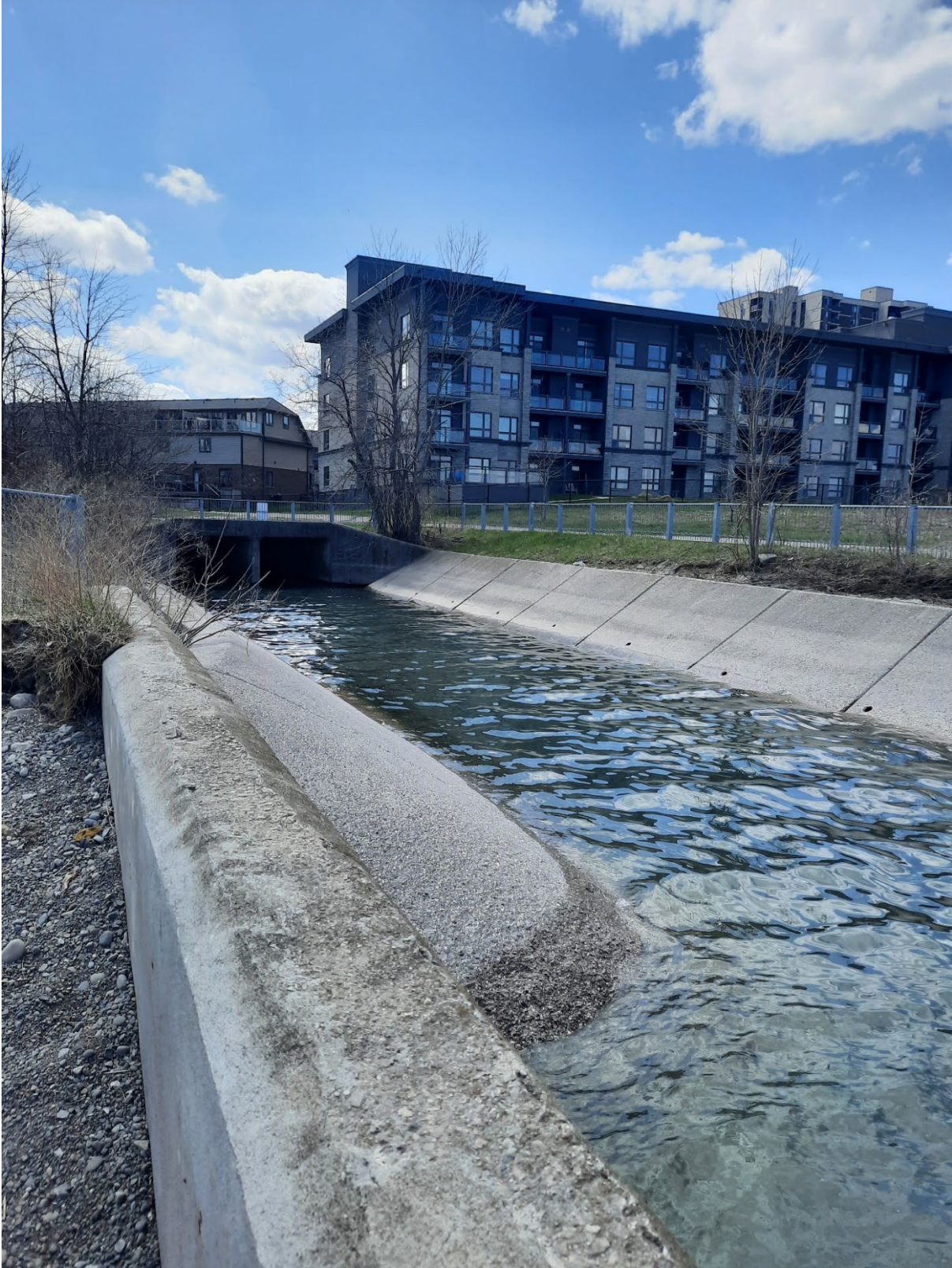
(Facing South, Storm Water Outfall adjacent to waterfront)
