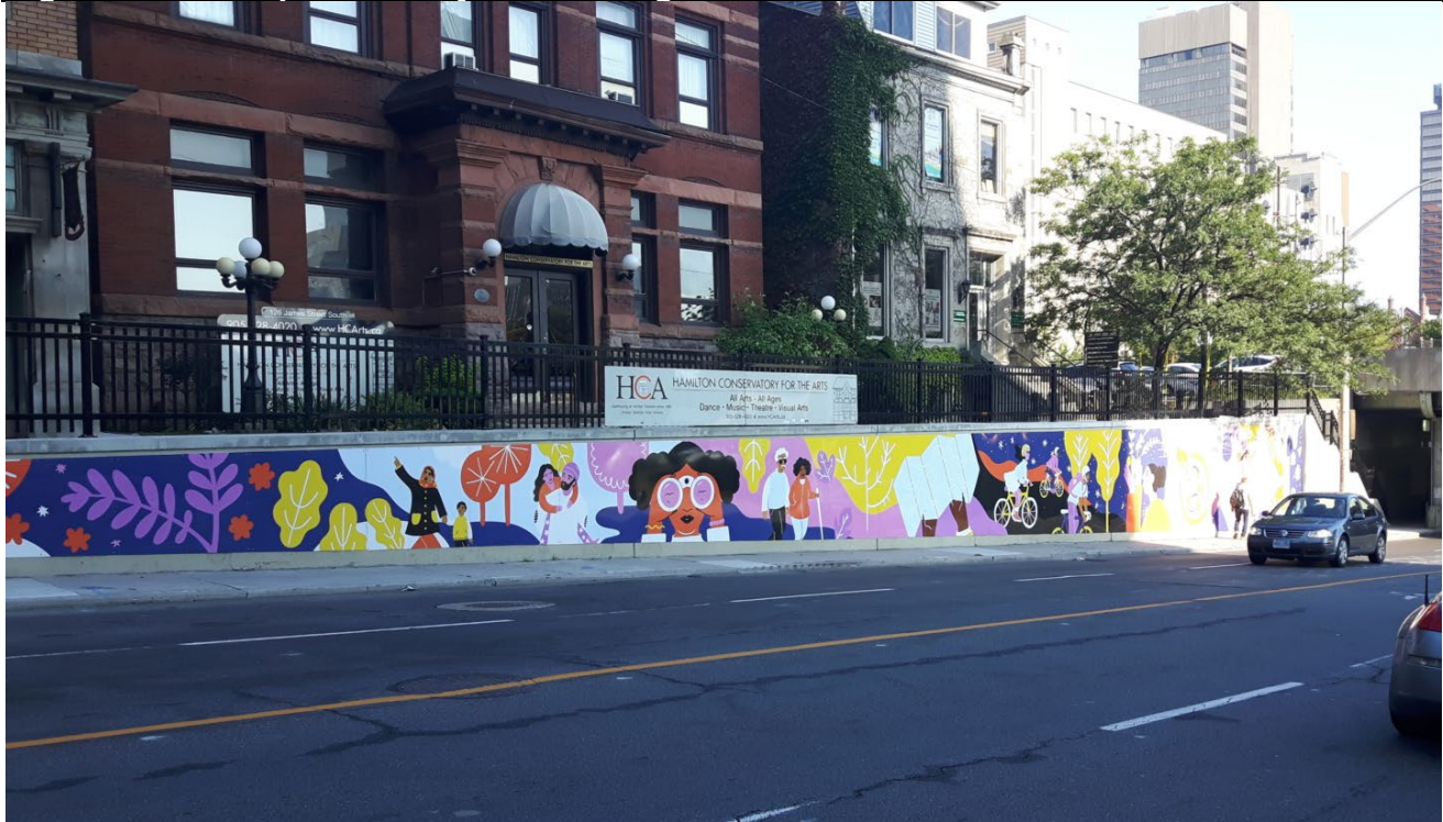
Figure 22: Example of a Major Retaining Wall on James St South
