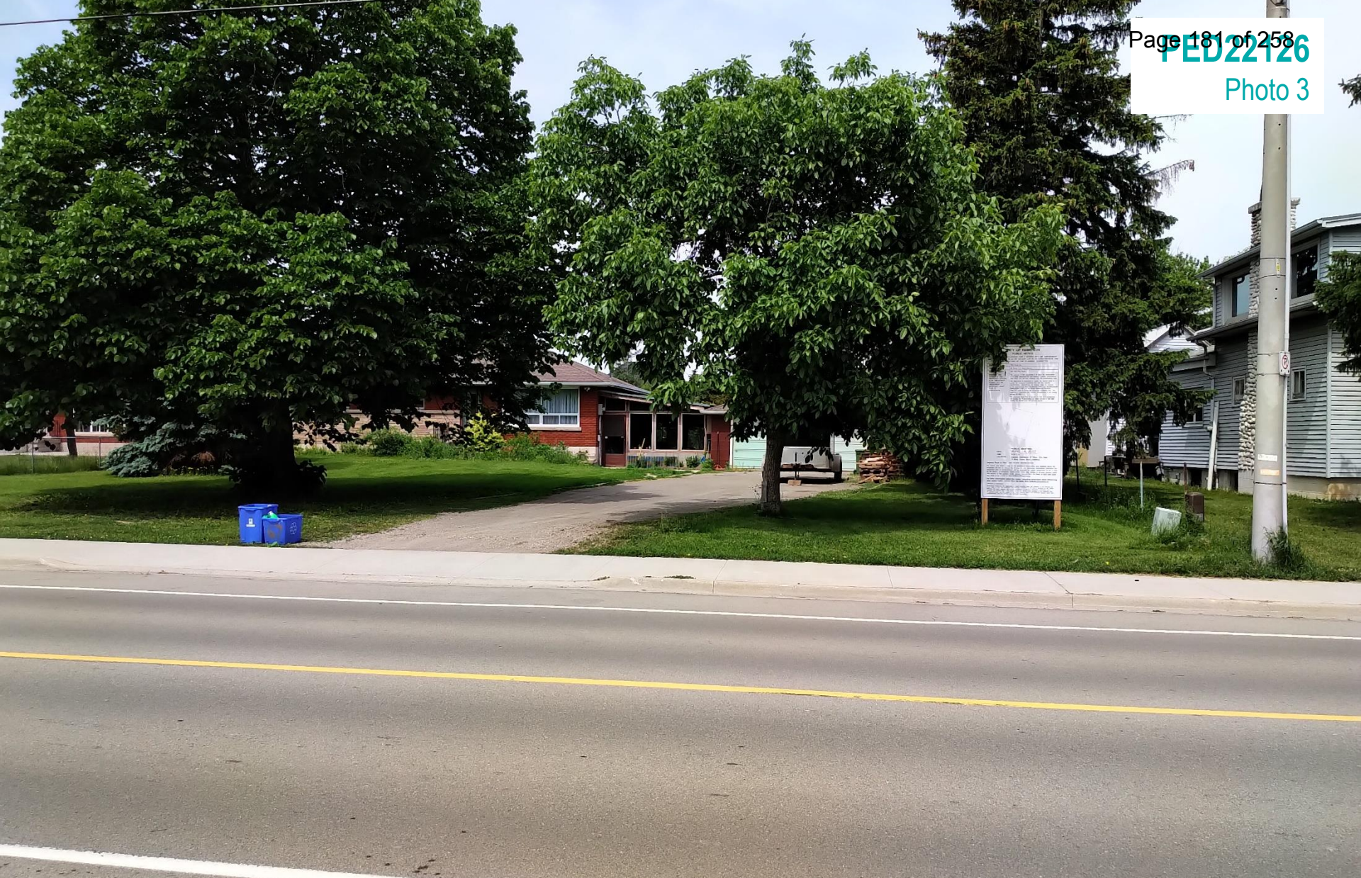
View of 541 Fifty Rd
