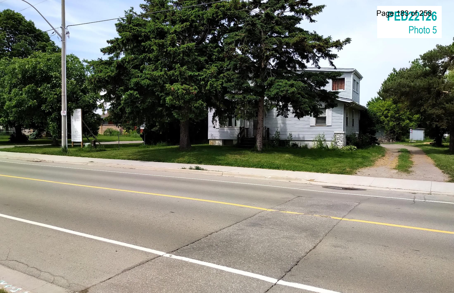
View of 545 Fifty Rd
