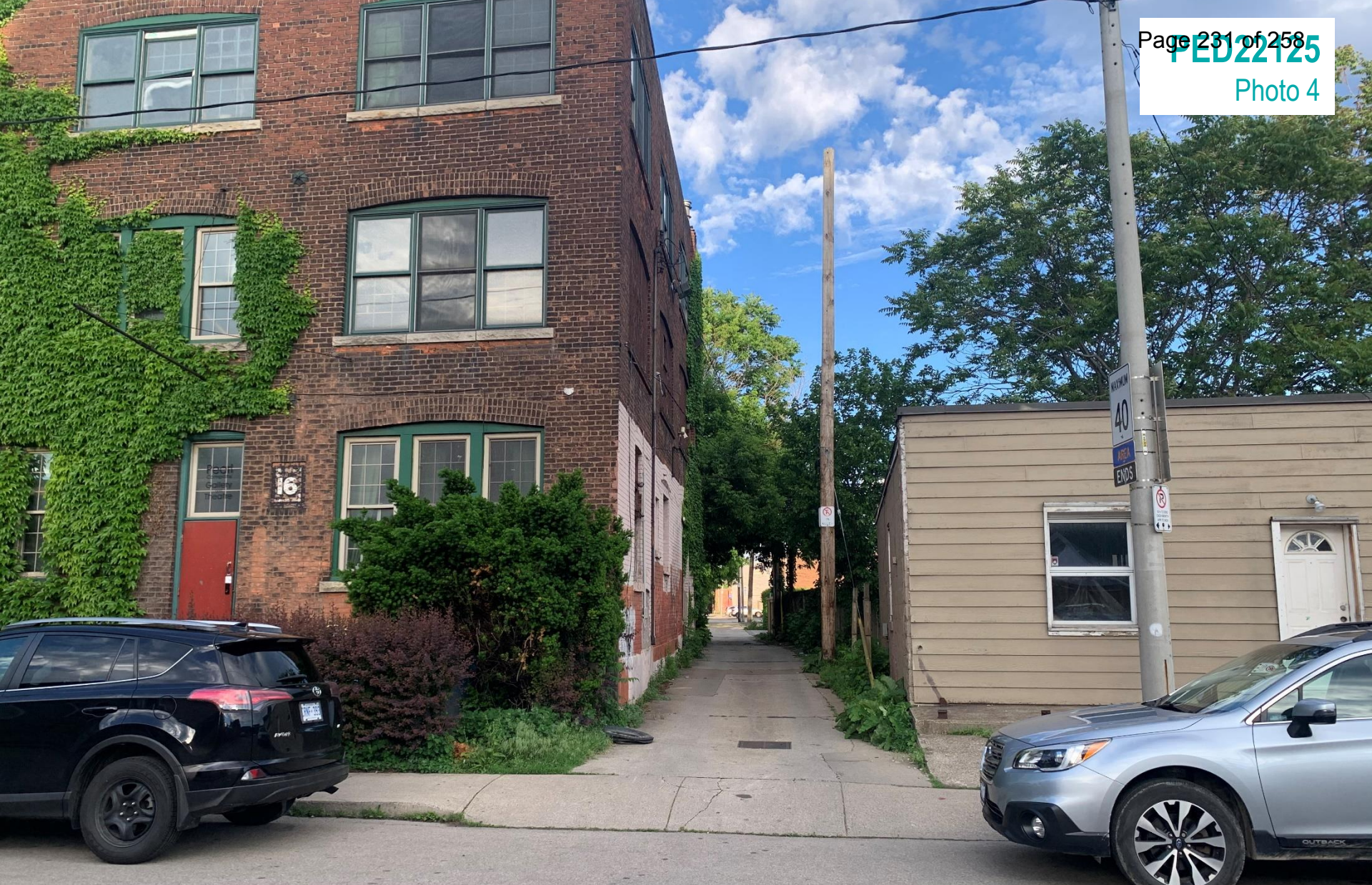
View of adjacent alleyway looking east on Steven Street
