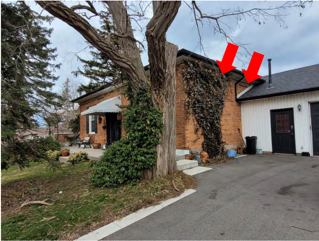
Figure 37: View of front and east side of the dwelling, noting locations of charred inset boards.
