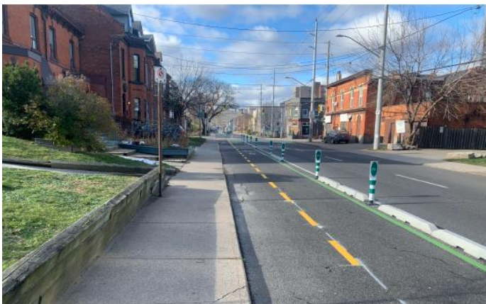
Hunter St, Hamilton Flexposts and precast curbs
