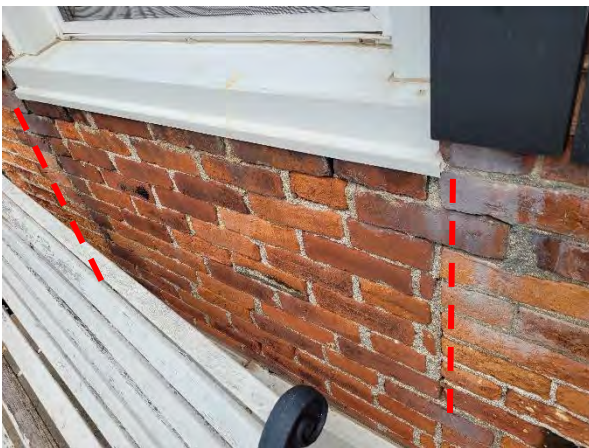
Figures 27 & 28: (left) Detail front elevation under west window (outlined in red), (right) Detail of front elevation under east window, noting areas where brick has been altered to remove original French windows (Source: MHBC, 2022)
