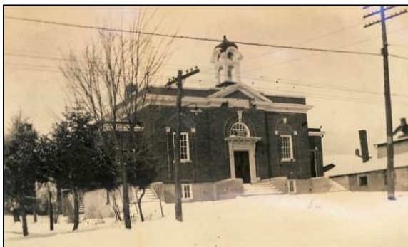
Figure 37: Memorial Hall, no date (Flamborough Archives)
