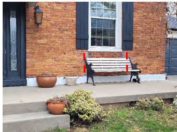
Figures 27 & 28: (left) Detail front elevation under west window (outlined in red), (right) Detail of front elevation under east window, noting areas where brick has been altered to remove original French windows (Source: MHBC, 2022)
