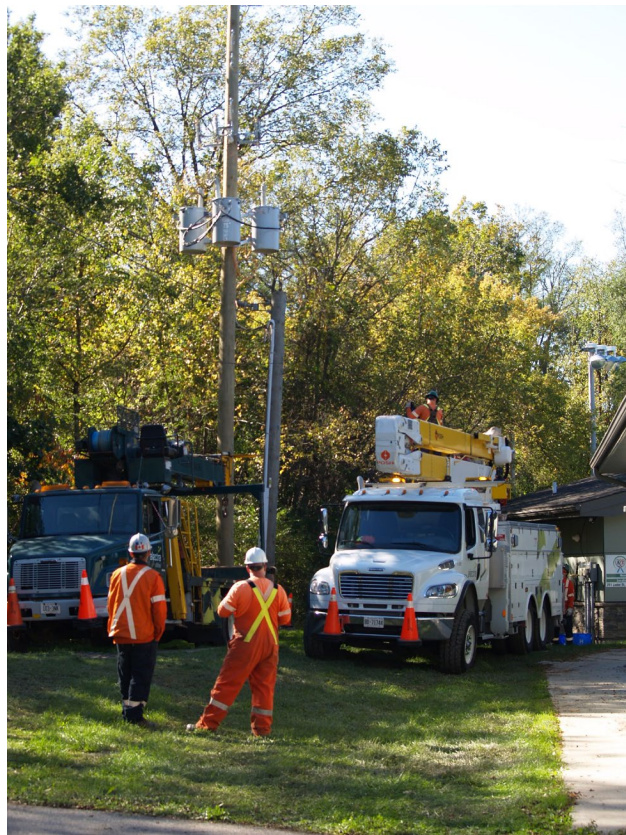
3 - Installation of the three phase transformer and additional wiring..
