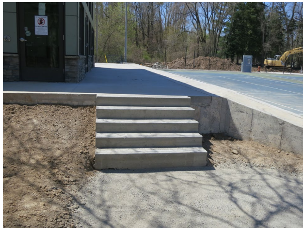
104 - 1st. week of May. Deck steps and concrete deck.
