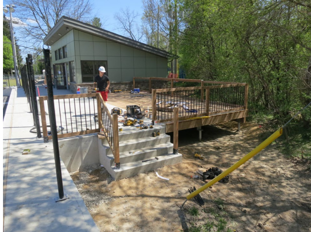
114 - May 13th. Wood deck and railings near completion.
