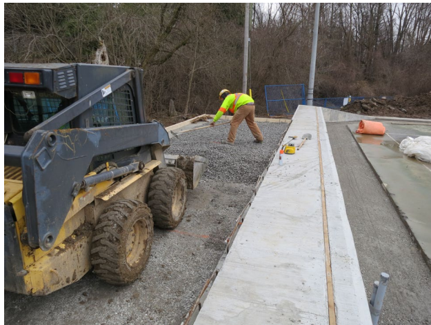
93 - April 19th. Granular base for the concrete deck
