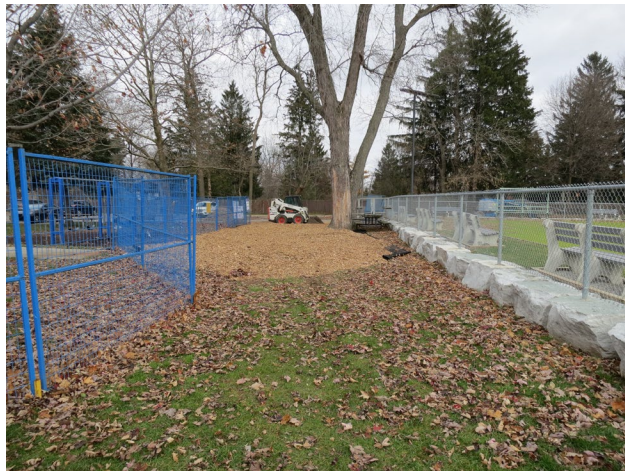
17 - Spreading of wood chips to protect the tree roots.
