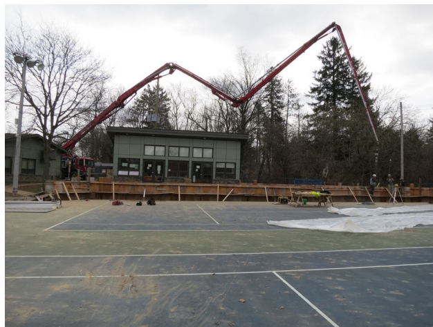
86 - April 13th. The long extension of the pumper's arm.
