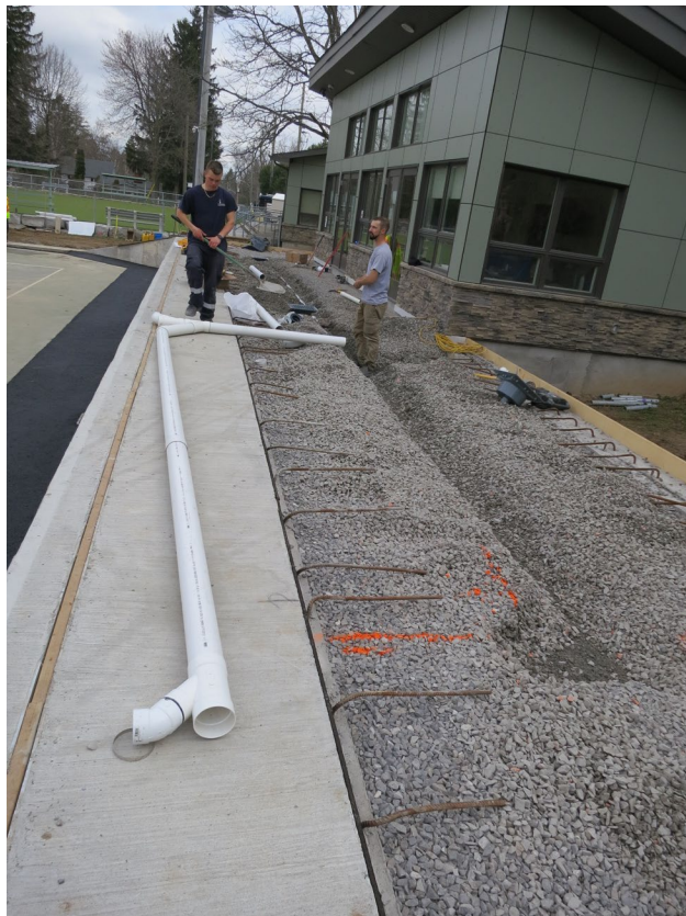
99 - April 25th. Installation of the deck drainage system.
