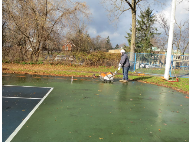
14 - Cutting of the asphalt.
