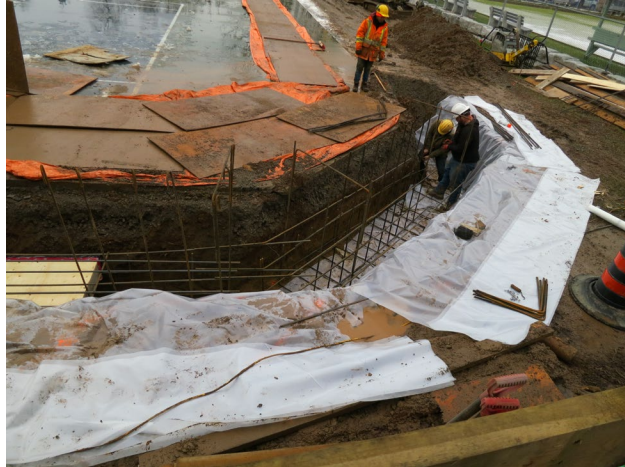
43 - Dec.30th. View of the construction at the North/East corner.
