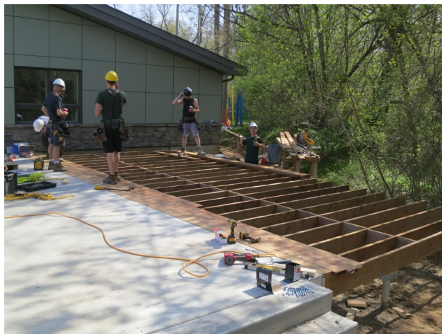
110 - May 12th. Construction of the deck extension.
