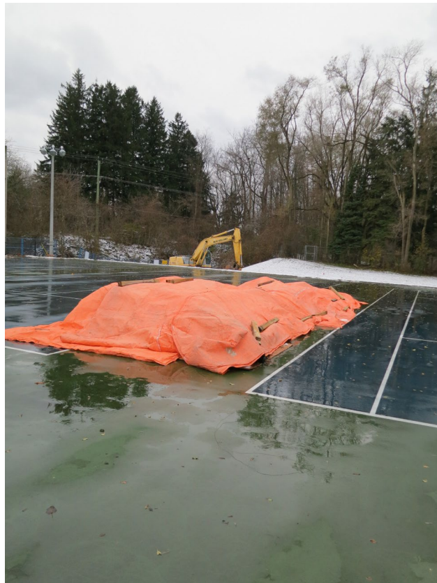
11 - Tarp on fencing materials.
