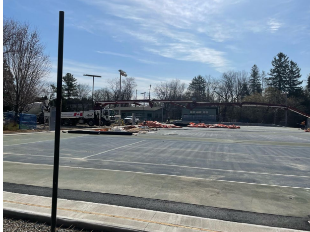
103 - April 29th. Pumping concrete for the mechanical and storage shed pad.
