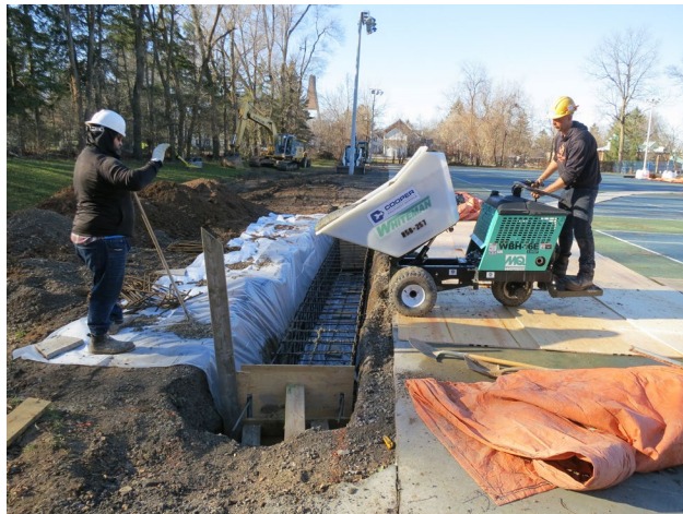
28 - Construction of the grade beam.
