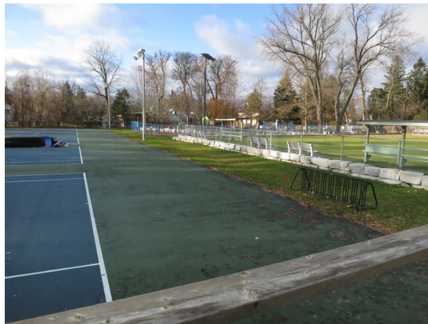
8 - View of the courts without fences.
