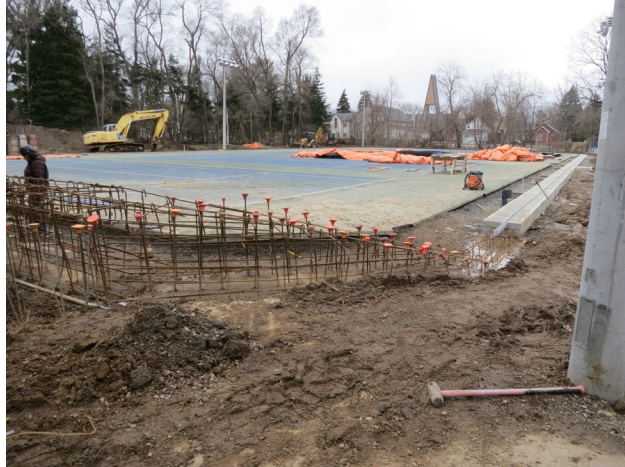
78 - April 1st. Reinforcing steel for the transition wall installed.
