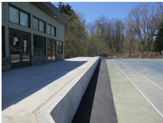
105 - 1st. week of May. View of completed concrete deck from Court 1.
