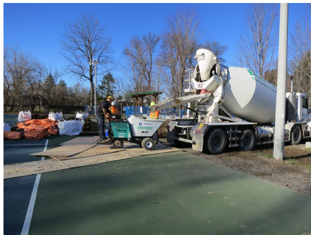
26 - A 9 cubic meter concrete delivery truck.
