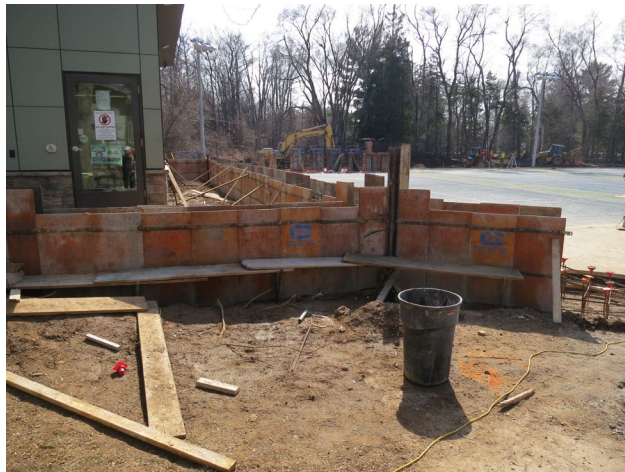
81 - April 5th. A side view of the formed deck walls.
