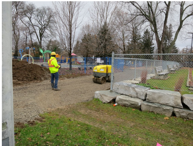
19 - Compaction of access road gravel base.
