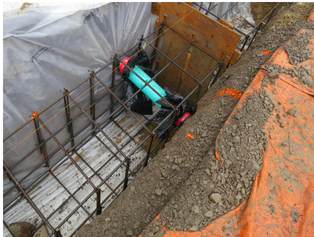
31 - Close up of 6" diam. PVC pipe.
