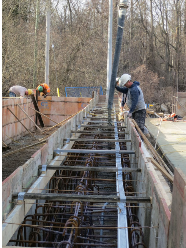
87 - April 13th. Construction of the deck wall.
