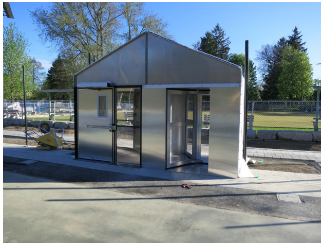
112 - May 13th. Completed Combo unit.
