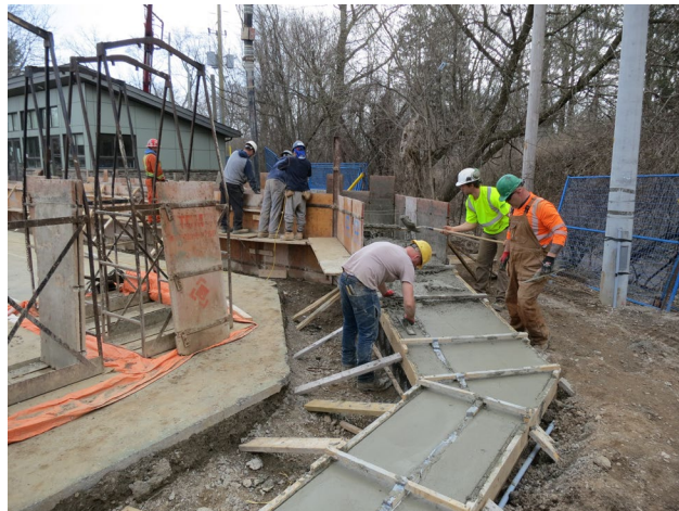
88 - April 13th. Working on the transition wall.
