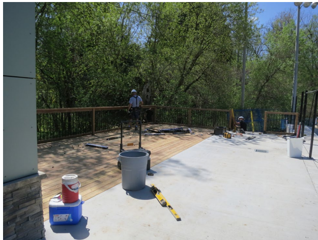
115 - May 13th. Another view of the larger wood deck extension.
