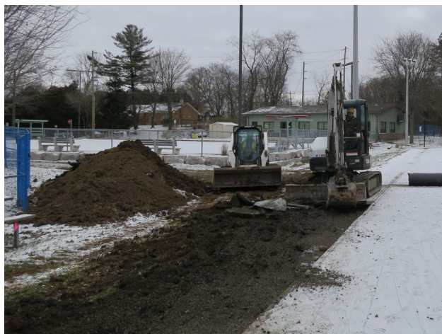
20 - Removal of asphalt.
