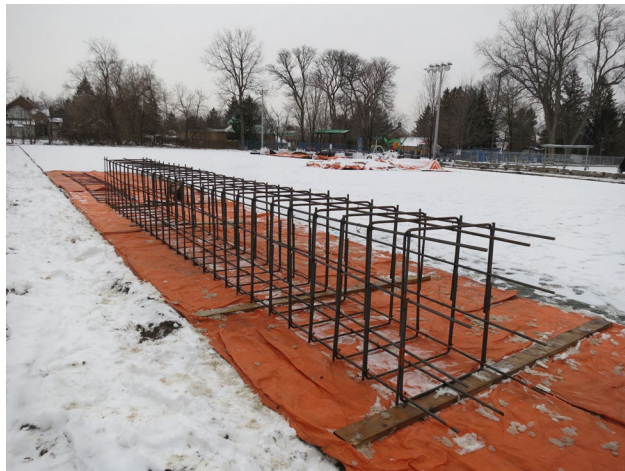
24 - Reinforcing steel cage for the grade beam.
