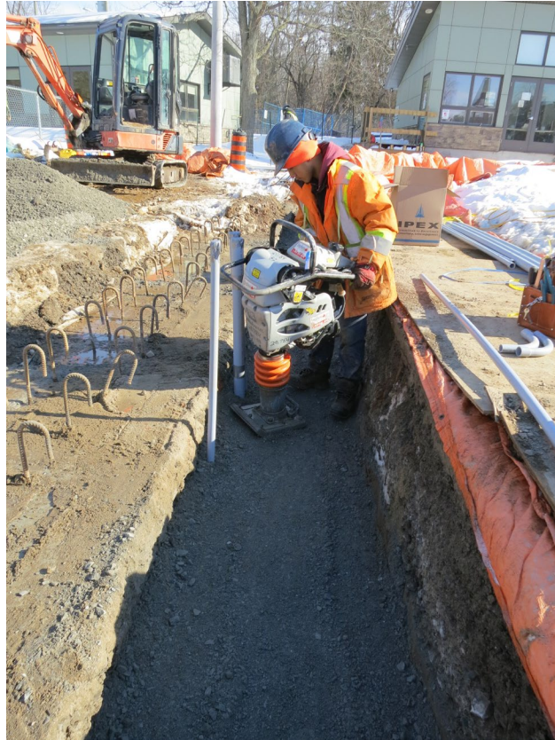
57 - Feb. 9th. Compaction of the granular fill.
