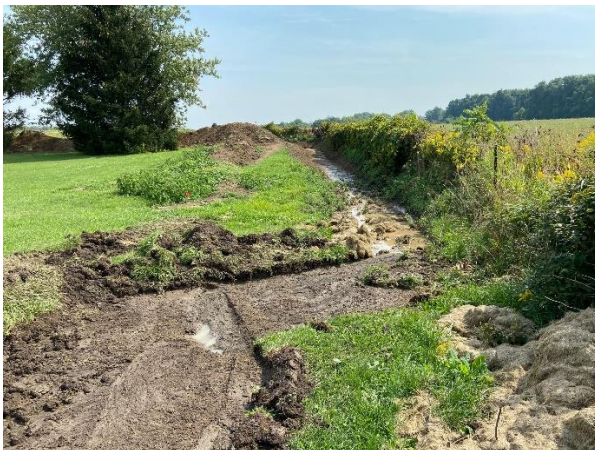
Creek was diverted to the periphery of the ground in order to maximize the ground radius
