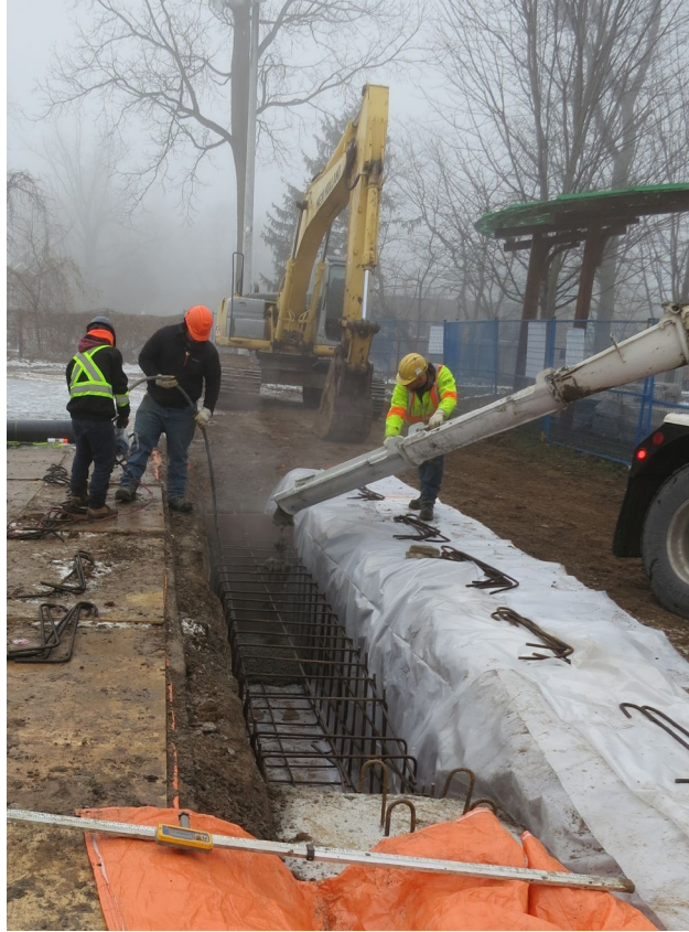
49 - Jan. 13th. Please note the steam coming off the heated concrete. In winter, most producers will try to have the concrete be between 20C - 25C when it leaves the plant.
