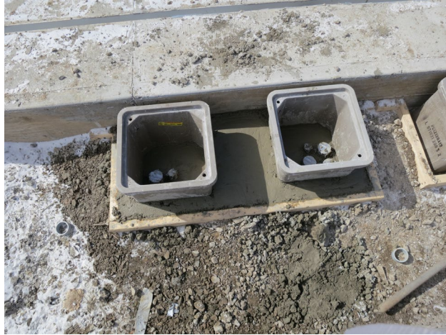
76 - March 28th. Installation of PVC junction boxes by Hillmer Electric.
