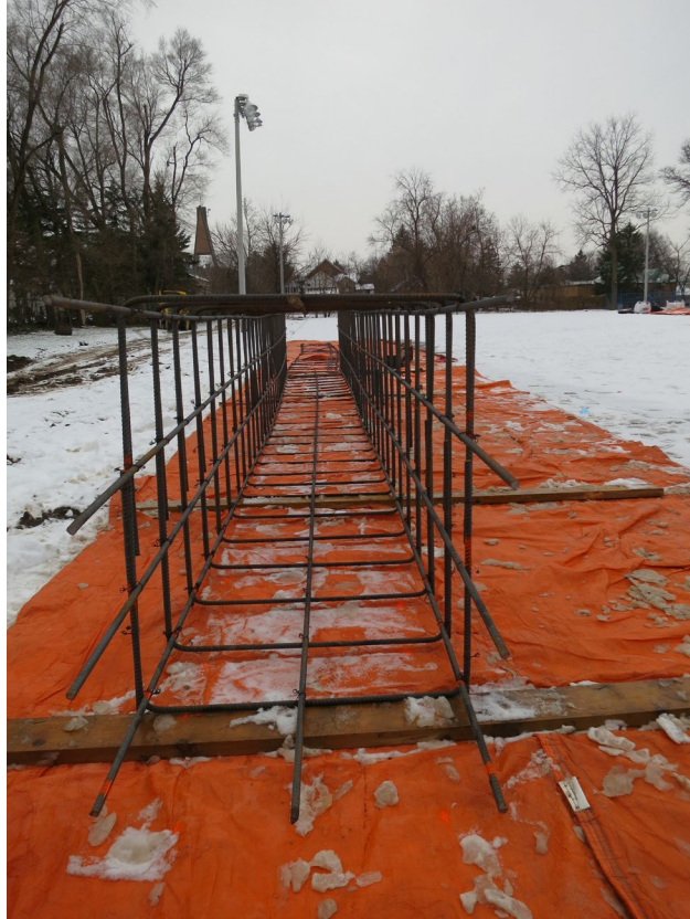
23 - Reinforcing steel cage for the grade beam.
