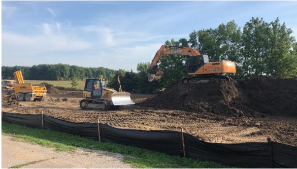
Grading in process
