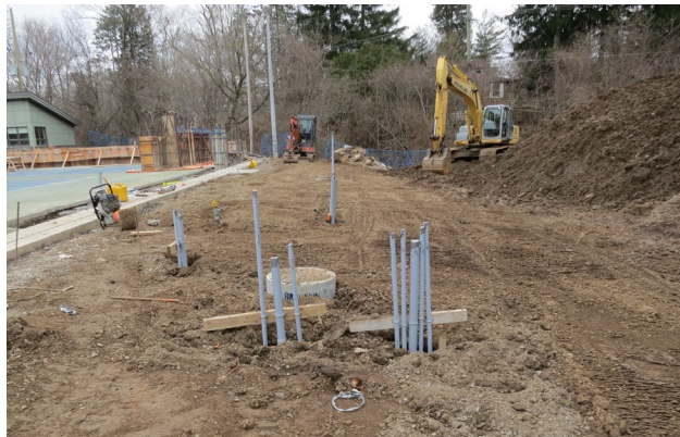
84 - April 8th. Trenches have been backfilled.
