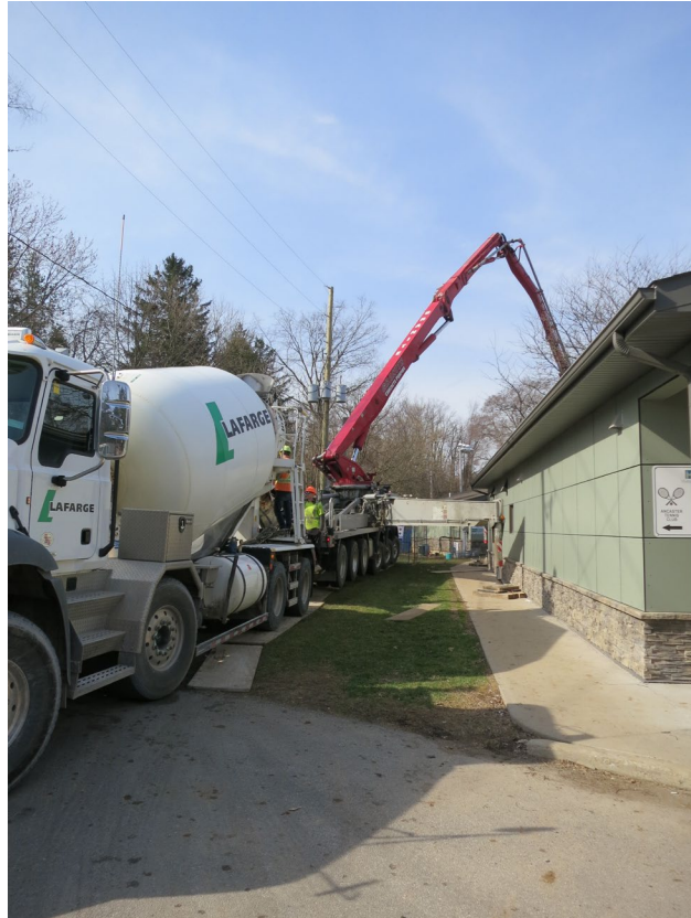
85 - April 13th. Big day for pouring/pumping concrete, 54 cubic meters
