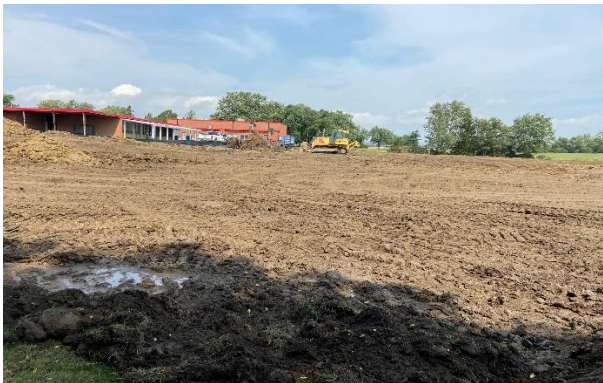
Grading in process
