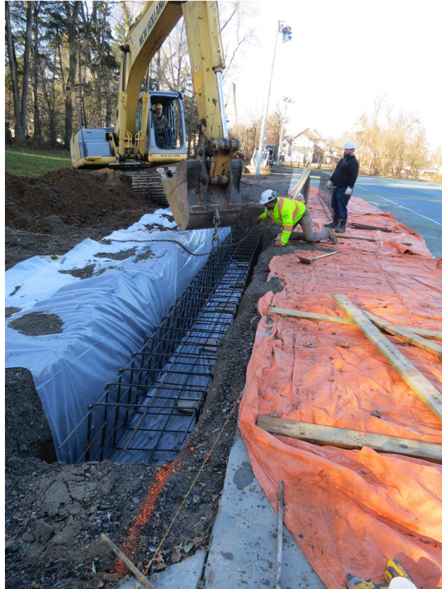
25 - Dec. 13th. Grade beam trench ready to receive concrete.
