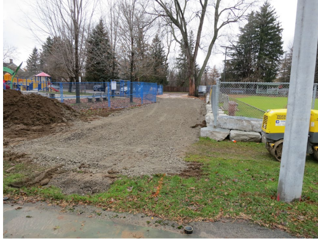
18 - North access route.
