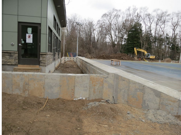
89 - April 14th, Deck walls and the forms were removed today.
