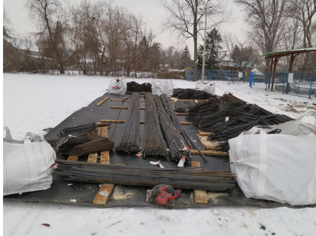
21 - Delivery of reinforcing steel.
