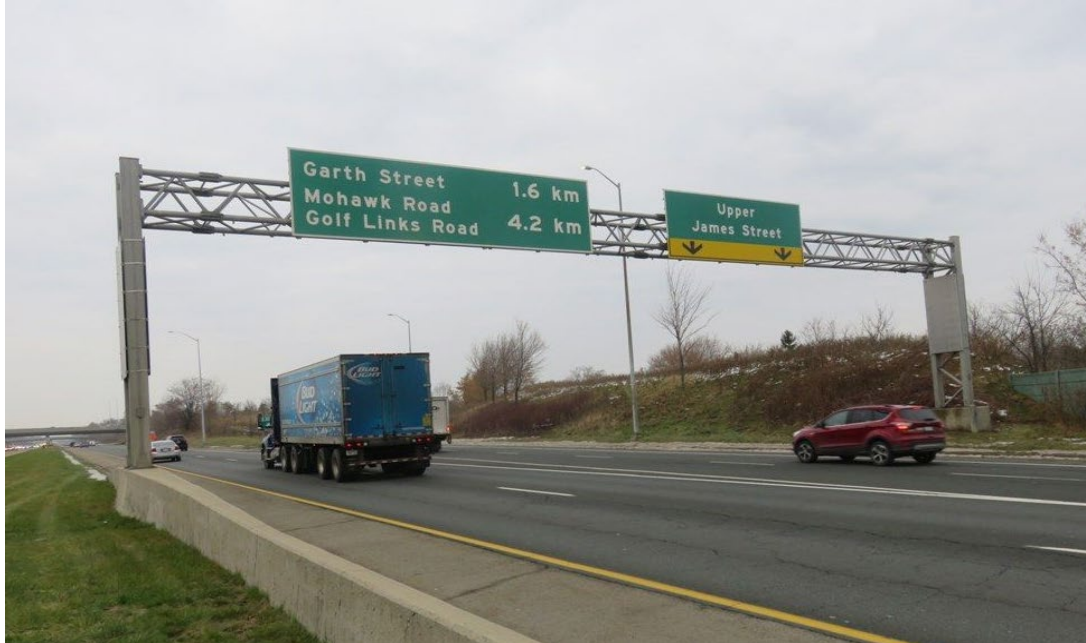
Figure 24: Example of ARL OSSS on the Lincoln Alexander Parkway
