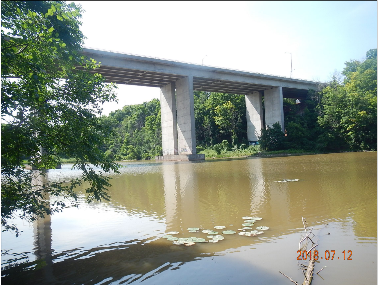
Figure 19: Example of an I-Beam / Girder Bridge on York Blvd
