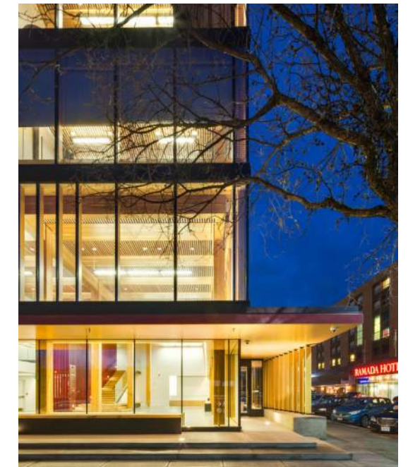
Wood Innovation and Design Centre UNBC, Prince George | Michael Green Architecture
