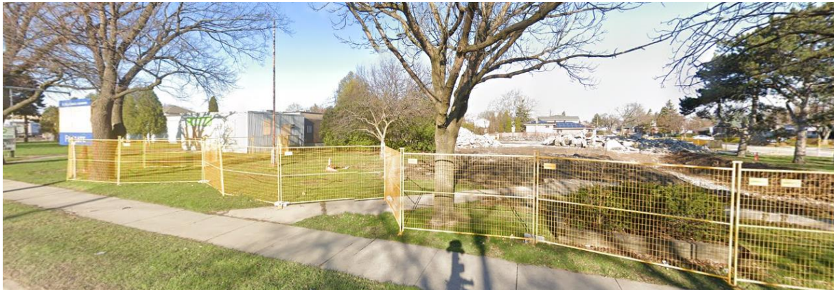
Existing Conditions (April 2022) – 488 and 500 Upper Wellington Street, Hamilton viewed looking southwest from Upper Wellington Street (Source: maps.google.ca)
