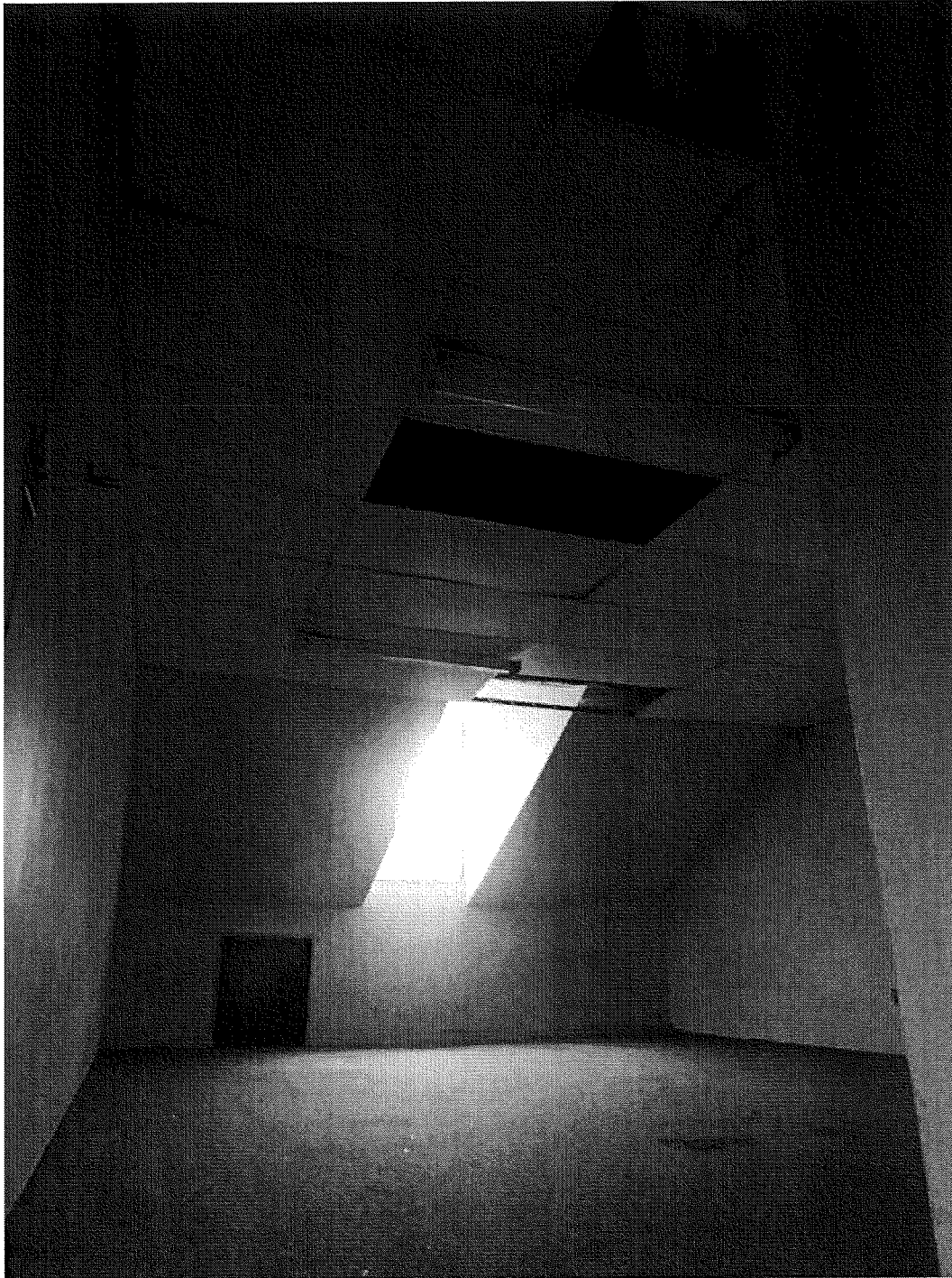
ATTIC – modern drywall and acoustic tile ceiling – no historic fabric
