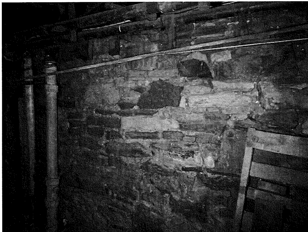
BASEMENT – original rubblestone foundation beneath the historic portion of the building
