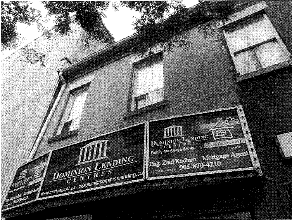
MAIN FAÇADE – original exterior wall and two window openings on the 2 nd floor are intact but the masonry has been painted and vinyl windows have been installed
