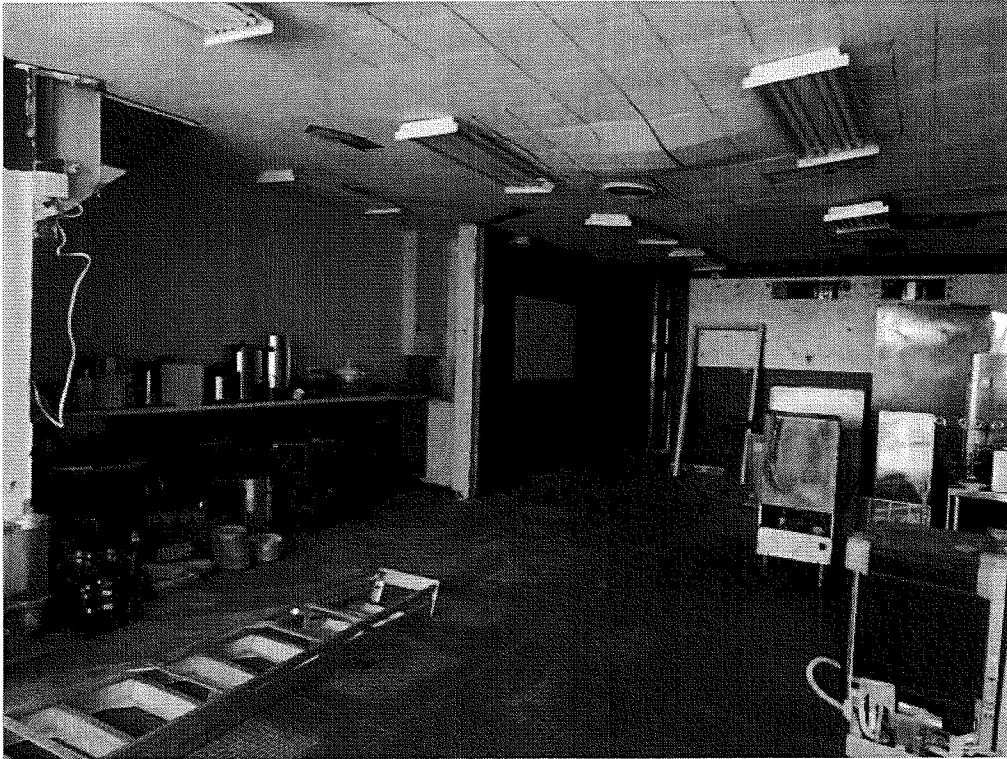
1 ST FLOOR COMMERCIAL SPACE – no historic fabric
