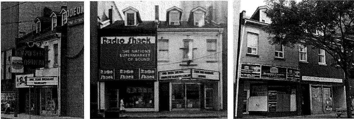
164 - masonry above the storefront was parged after the Public Optical signage was removed
