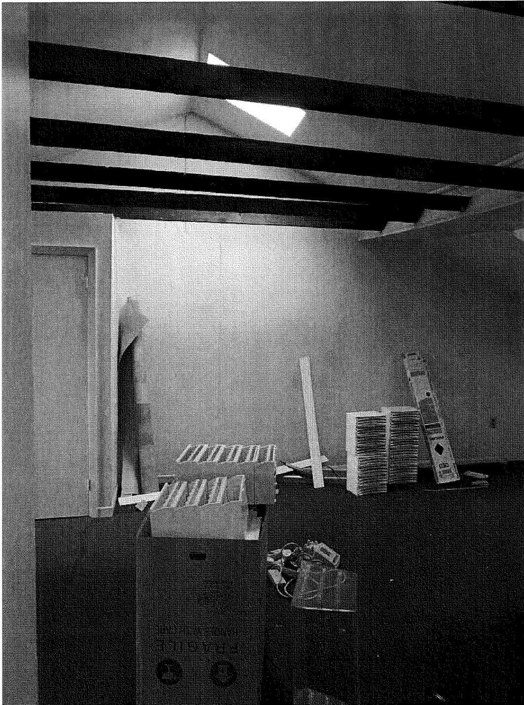
ATTIC – modern drywall and popcorn ceiling – framing timbers are exposed
