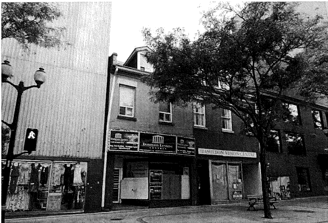
KING STREET EAST – two roof dormers
