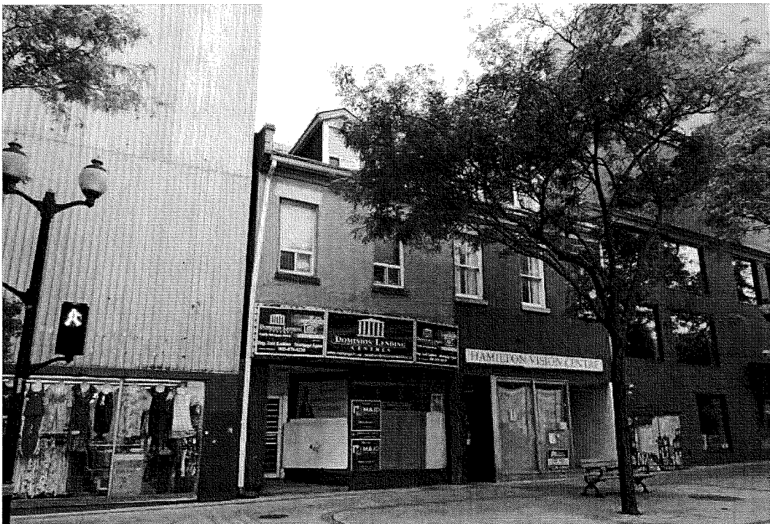
KING STREET EAST – one roof dormer
