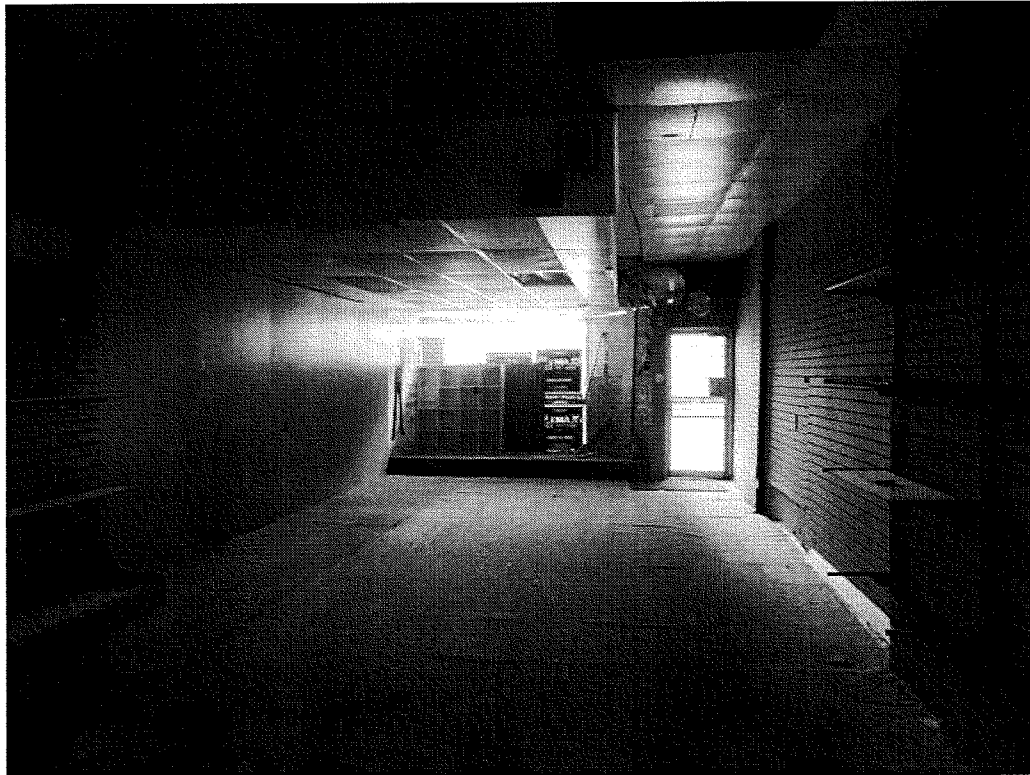
INTERIOR 1 st floor – no historic fabric
