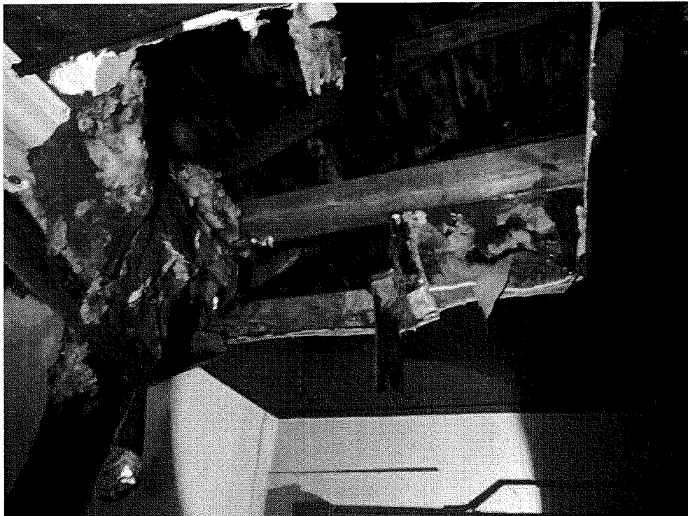
2 nd FLOOR – rear section – original roof framing visible through a hole in the ceiling – evidence of water and fire damage
