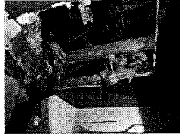
SATURATED INSULATION & COLLAPSED CEILING TILES
