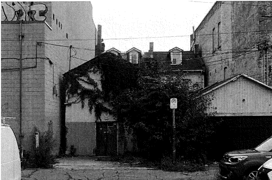
BRICK STORAGE SHED – there is a brick storage shed attached at the rear that backs onto the alleyway
