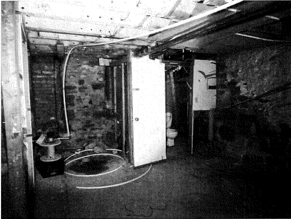
BASEMENT – rubble stone foundation below the front portion of the building
