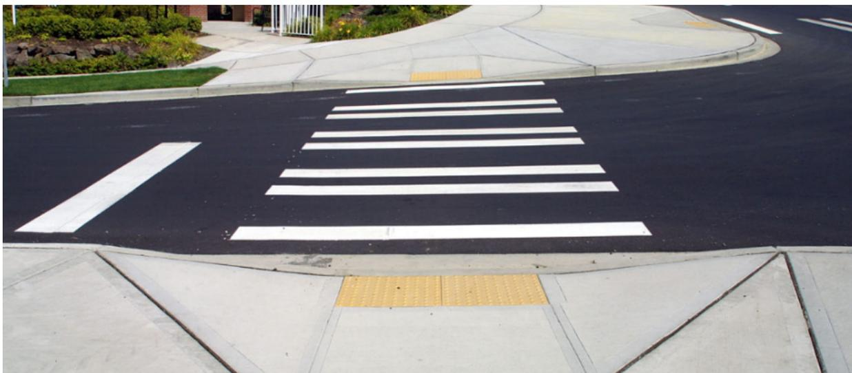
*Example of a depressed curb ramp at a pedestrian crossing in Washington State. Source: Pedestrian Safety Guide and Countermeasure Selection System*
