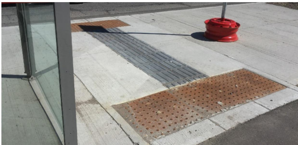
*A guidance TWSI in grey used to guide pedestrians between a bus stop (left) and a cycle track crossing (right). Red attention TWSI's are used to identify hazards at each end. Ottawa, ON*
