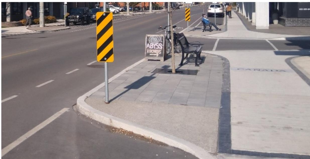
*A curb extension at an intersection offers additional seating and an extended pedestrian crossing.*
