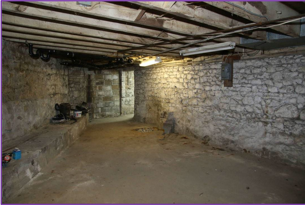
Another view of the basement area (orientation unknown).
