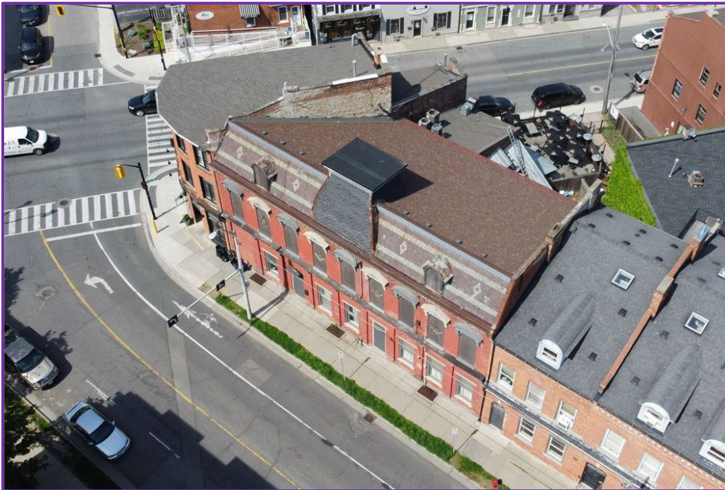
Aerial view of the building showing the Mansard roof face, the cupola and the gently sloping roof from the peak of the Mansard to the rear façade. Brick masonry parapet walls separate this building from the adjacent earlier commercial blocks. (courtesy of Craig Knapman)
