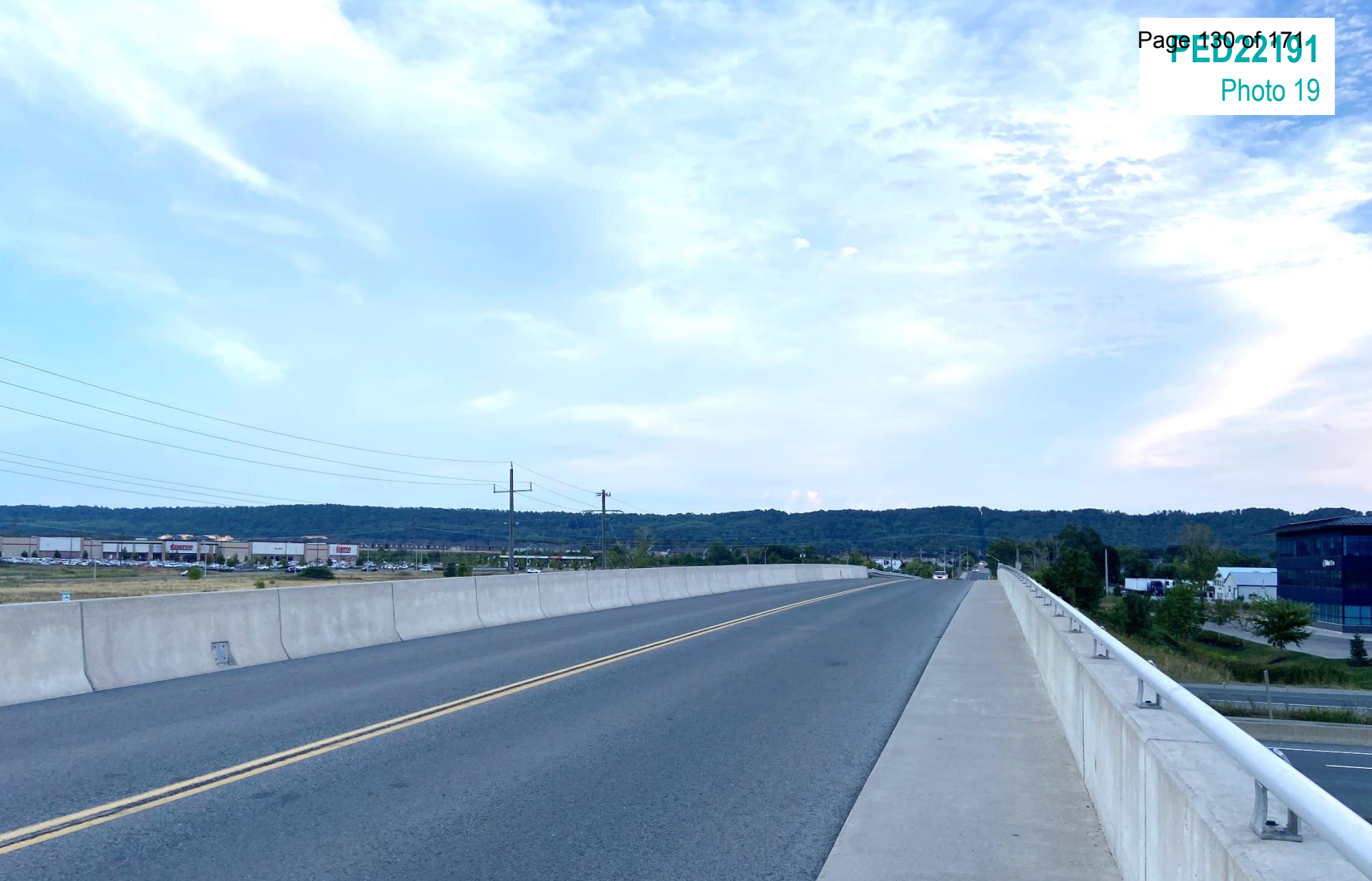
View looking south on Winona Road bridge
