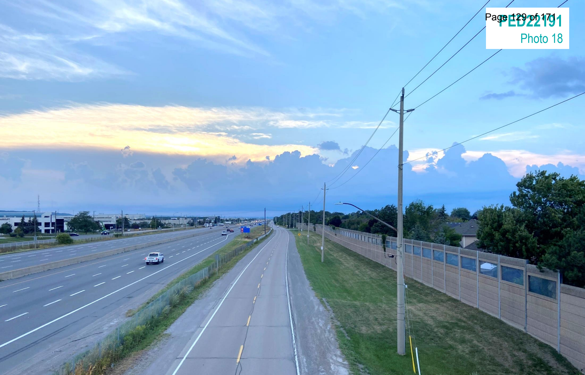
View of QEW looking west
