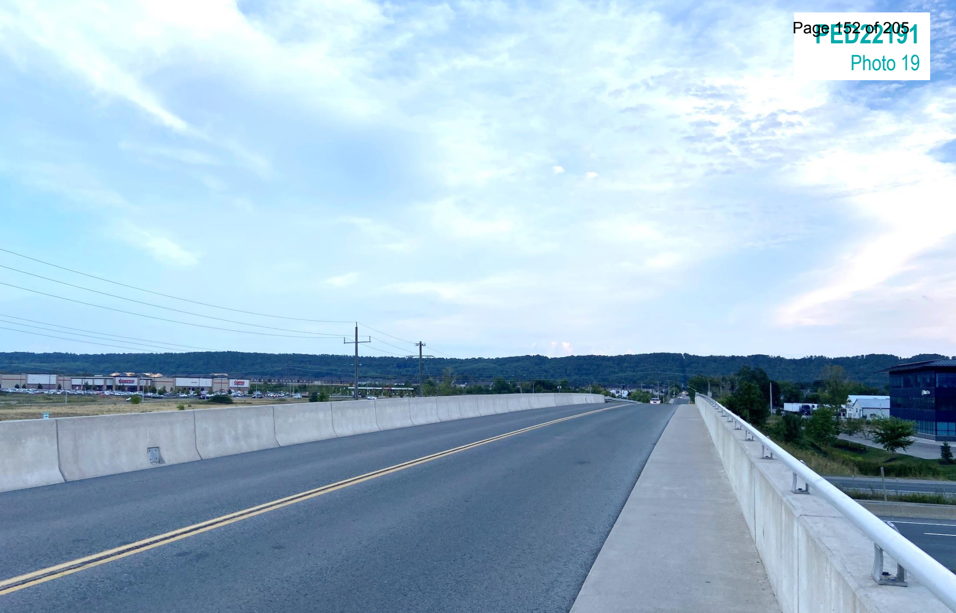
View looking south on Winona Road bridge
