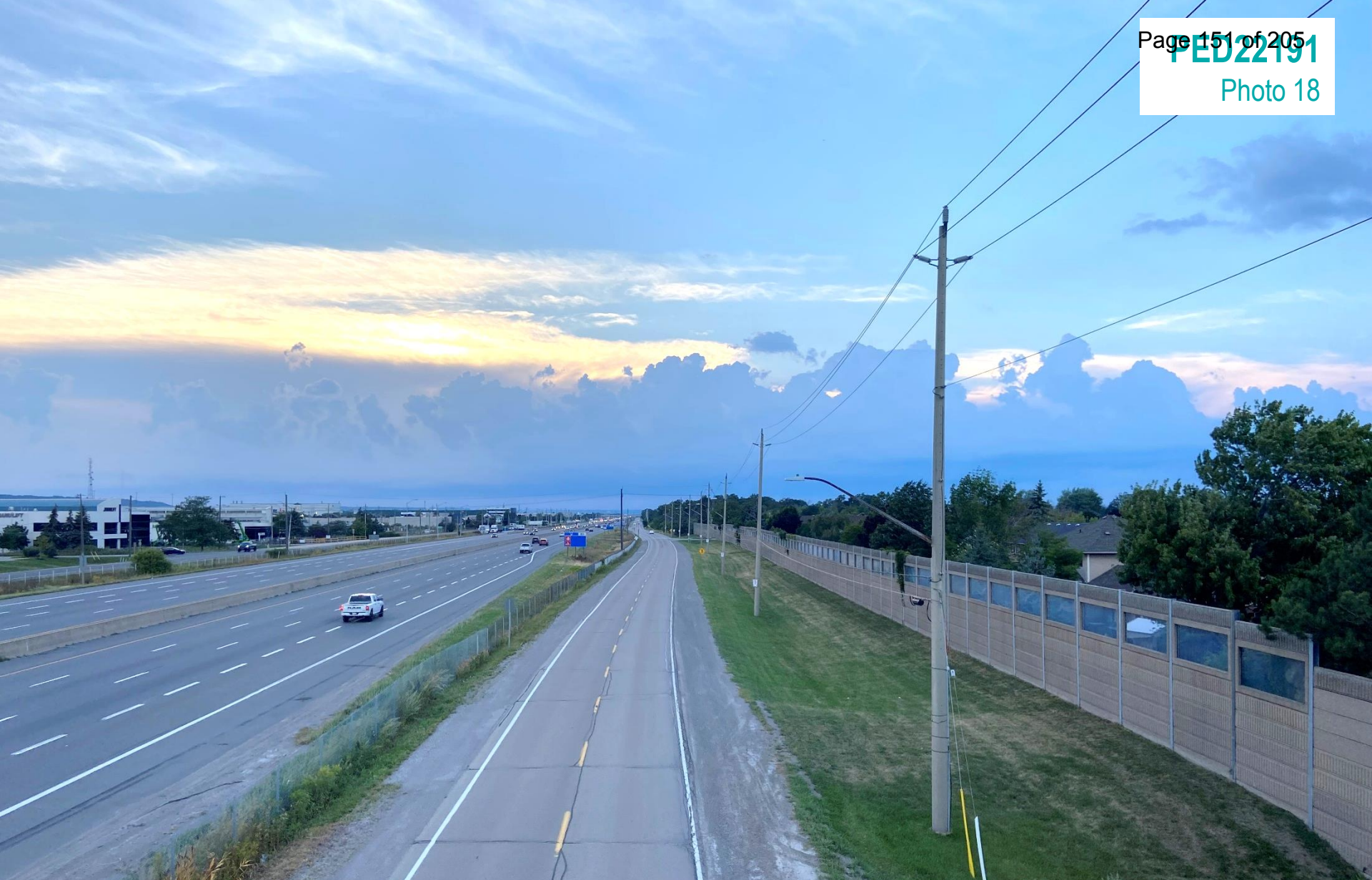
View of QEW looking west
