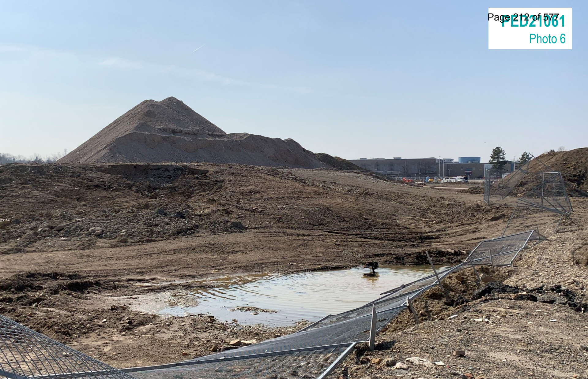
Looking west from the south
