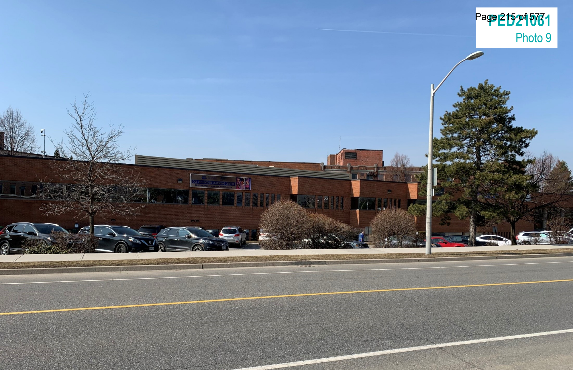
565 Sanatorium - building north of Southam
