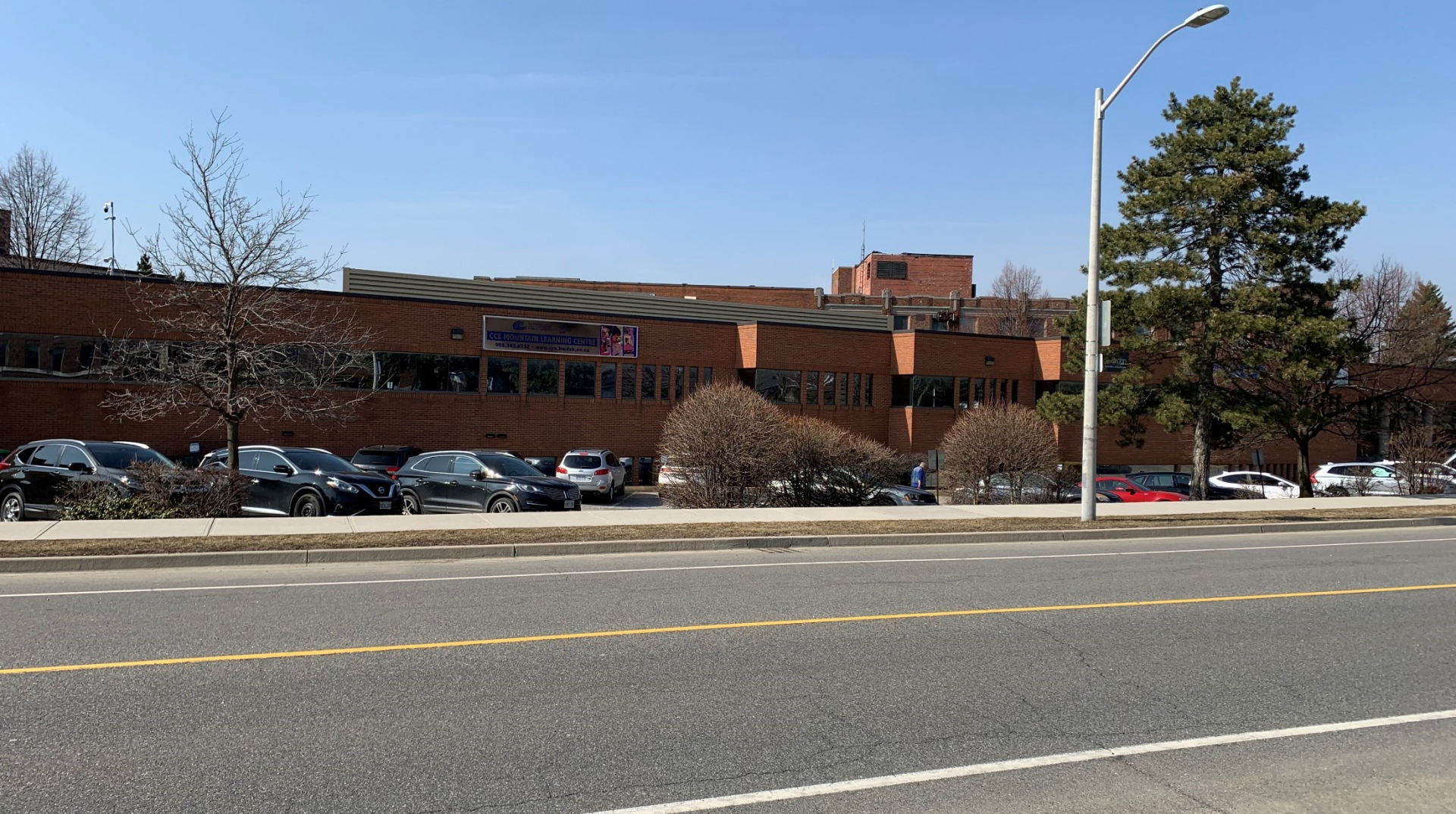
565 Sanatorium - building north of Southam
