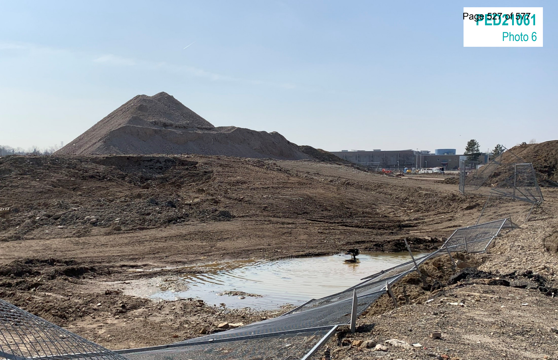
Looking west from the south
