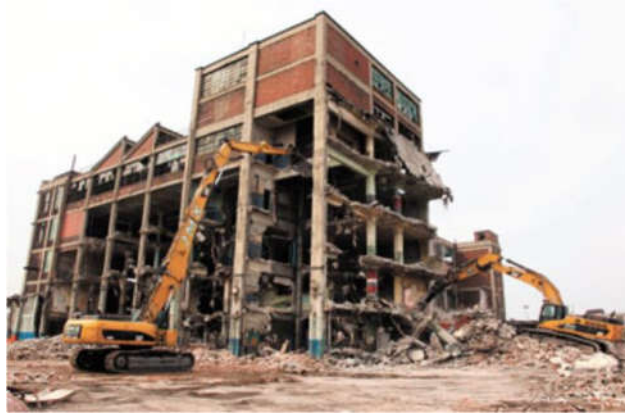
Demolition of Firestone Tire plant in Hamilton, Ontario – Source Construct Connect
