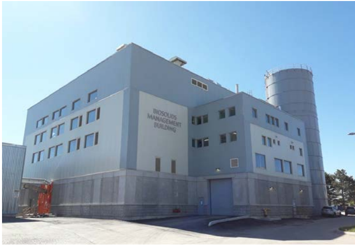
Biosolids building, Woodward WWTP
