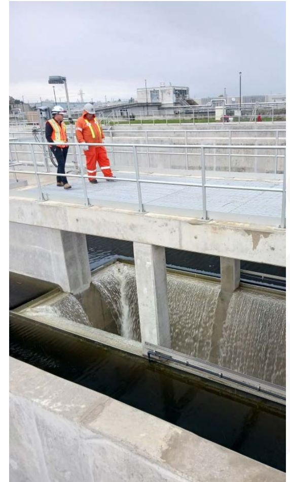
Tertiary Treatment - Woodward WWTP
