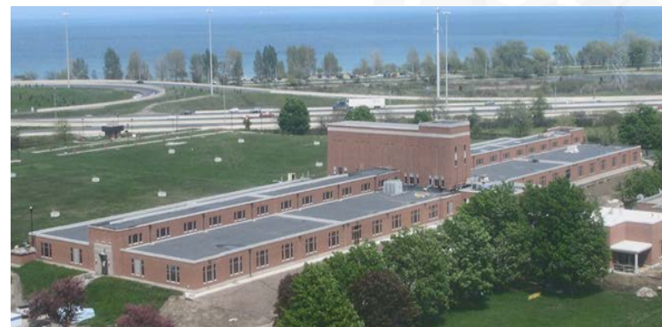
Woodward WTP Pre-treatment and Filter Building
