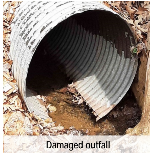
Erosion, damaged infrastructure
