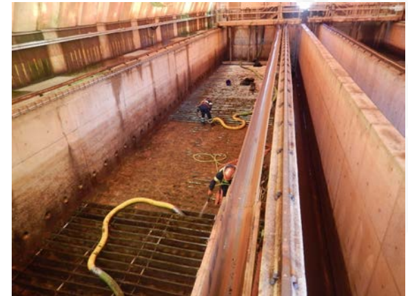
Dundas WWTP upgrades
