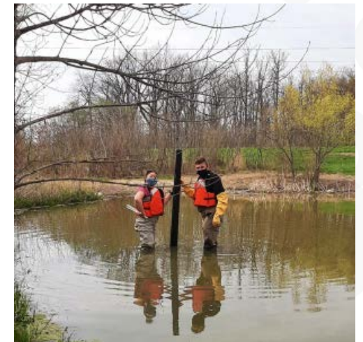
Stormwater management facility requiring dredging
