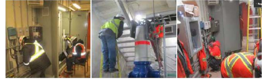
First Street Wastewater Pumping Station Capacity Upgrades – $4.4M
