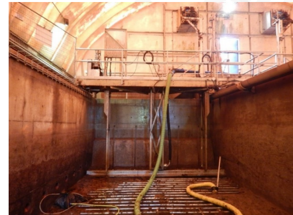
Dundas WWTP repairs
