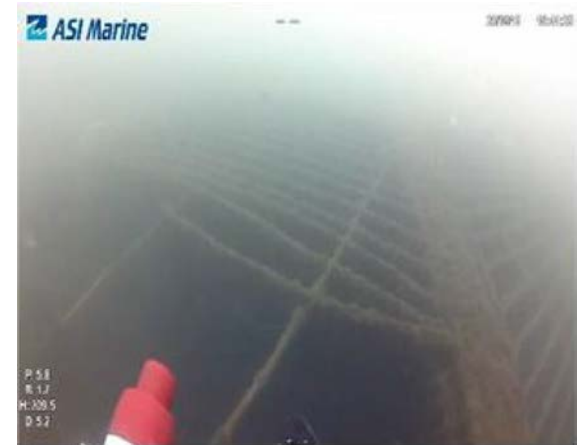
Low lift raw water intake
