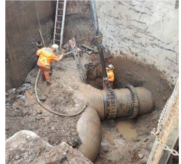
Woodward WTP upgrades
