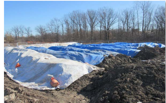
Excess soils, Woodward WWTP
