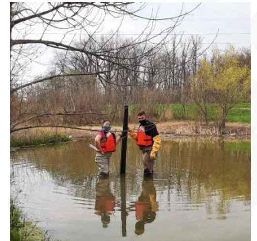
Stormwater management facility requiring dredging
