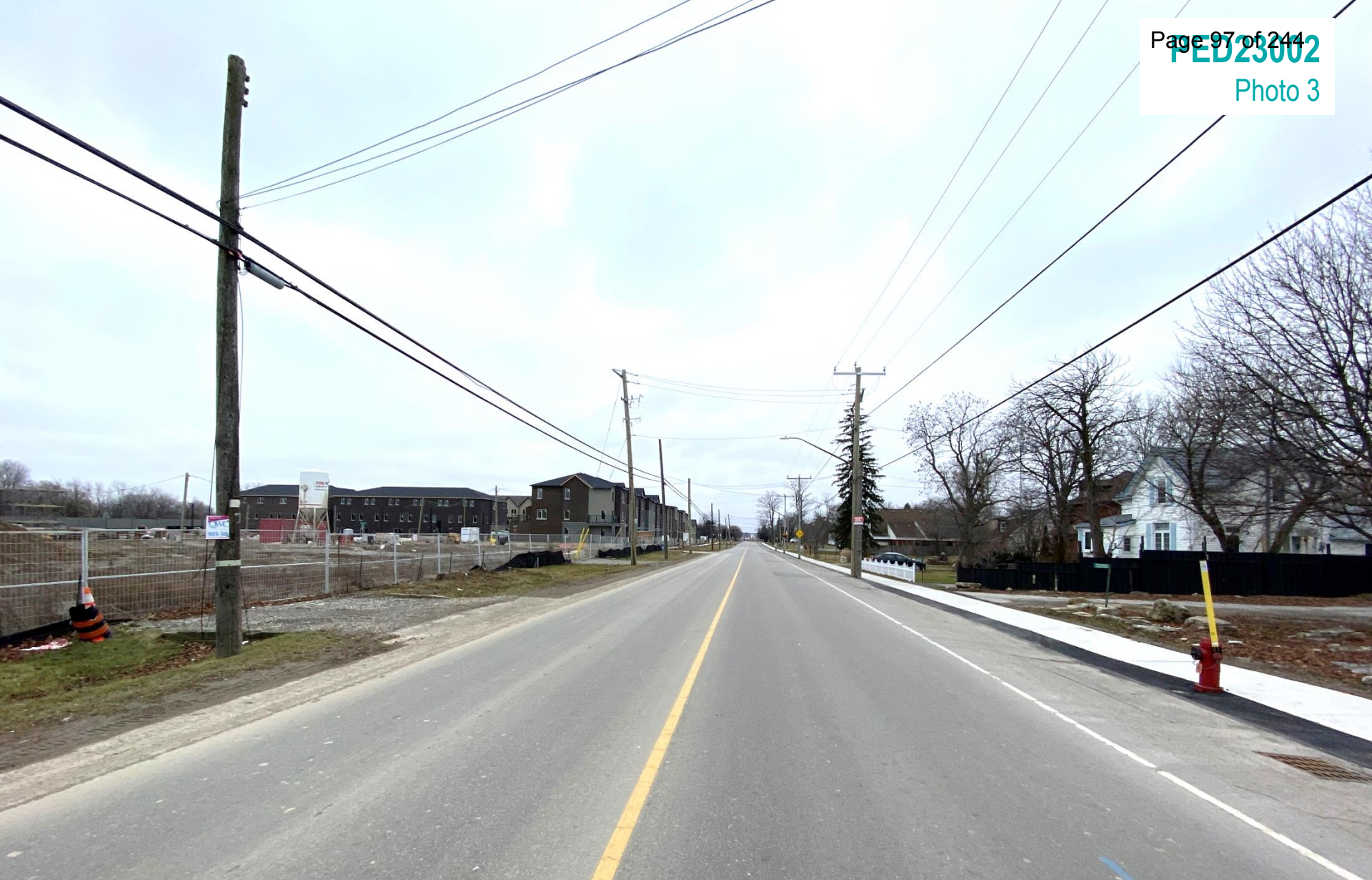
Looking South on Homestead Drive
