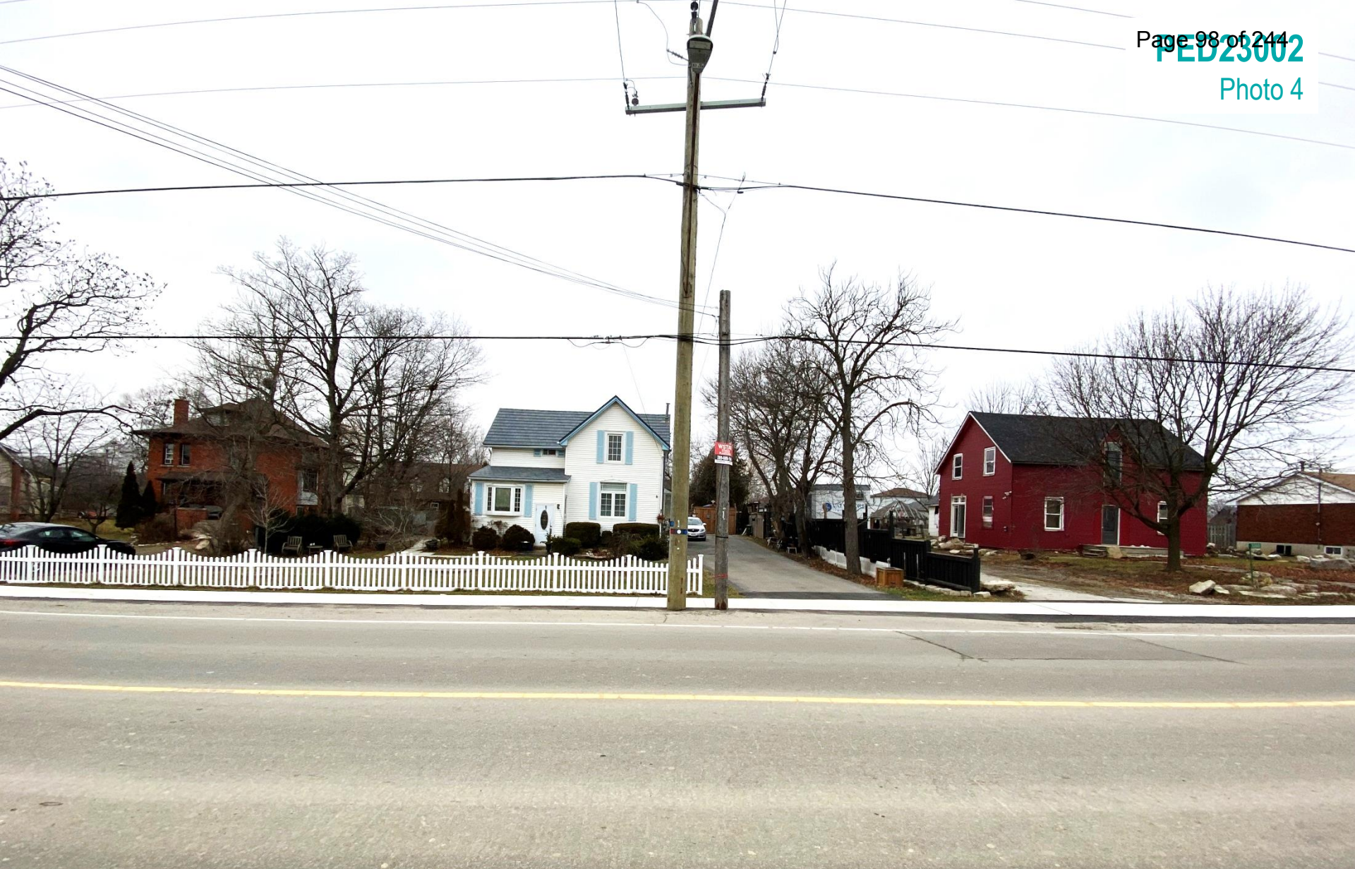
View of neighbouring property south of site
