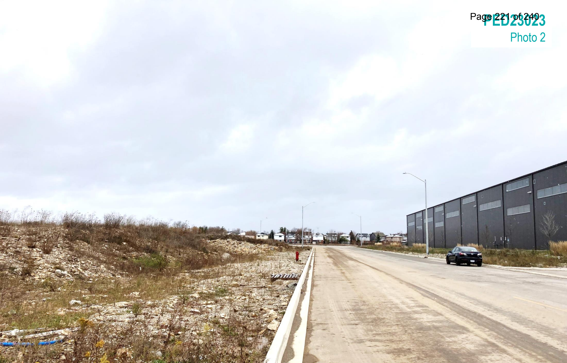
Looking east from Enterprise Crescent
