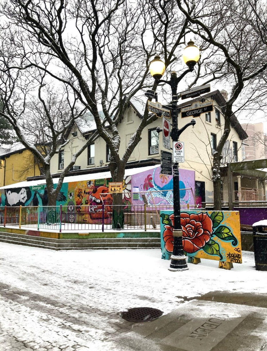
Looking at the building of 115 and 117 George which will be retained as part of the application
