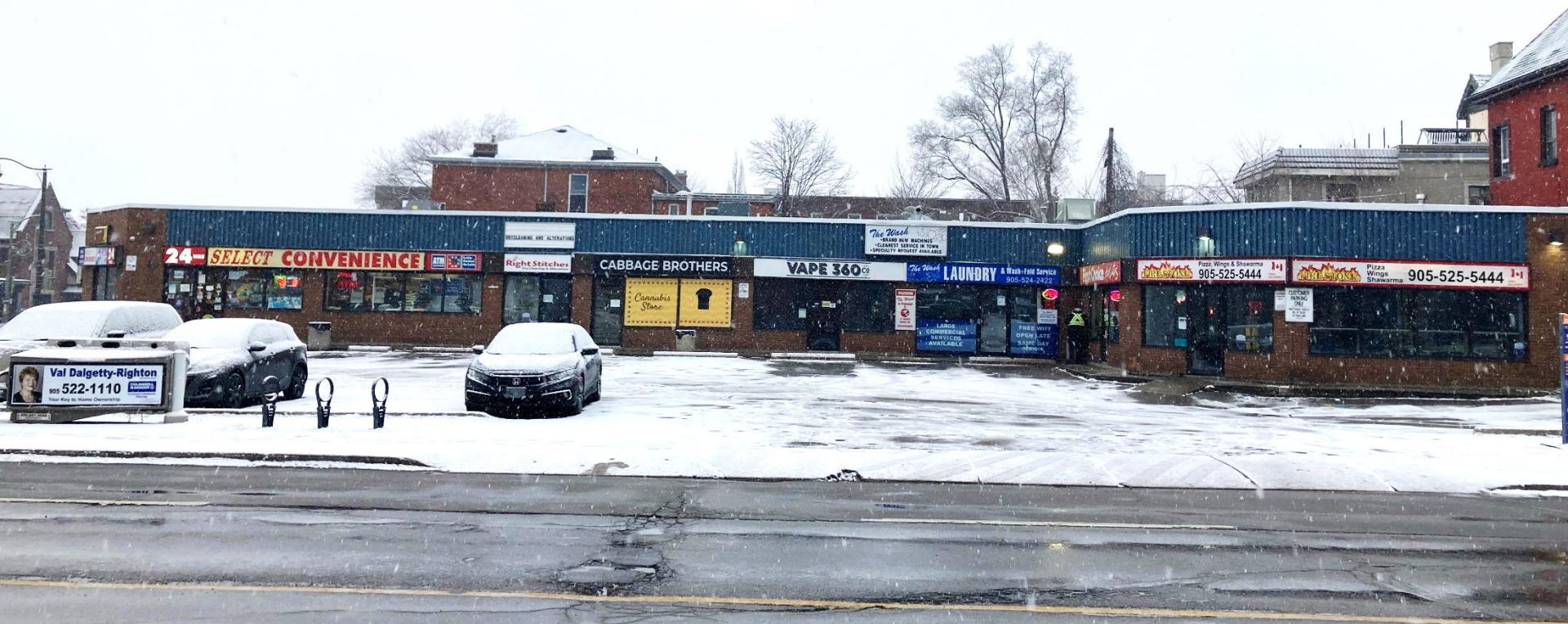
Looking west of the Subject Lands (Northwest corner of the intersection of Queen Street South and Main Street West)
