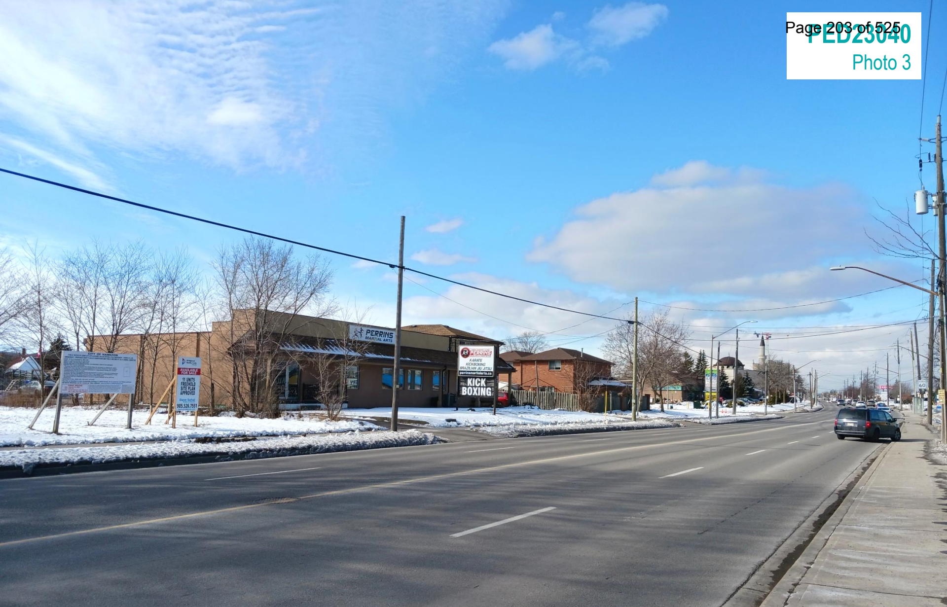
Adjacent commercial property to west
