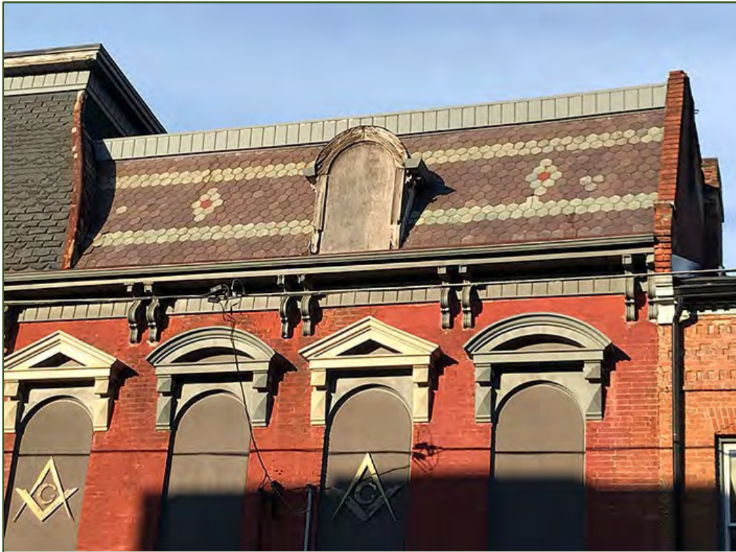
Close-up-view of four of the upper storey galvanized-iron window hoods, bracketed cornice and the deteriorated state of the dormer windows with the exposed woodwork of the window frame. The installation of ribbed aluminum sheathing to the fascia panels at the top of the cupola and main roofs and the bracketed cornice was an adverse alteration made since 1996 (likely as a weather-proofing measure and to replace deteriorated metalwork). Photo by the author, August 2022
