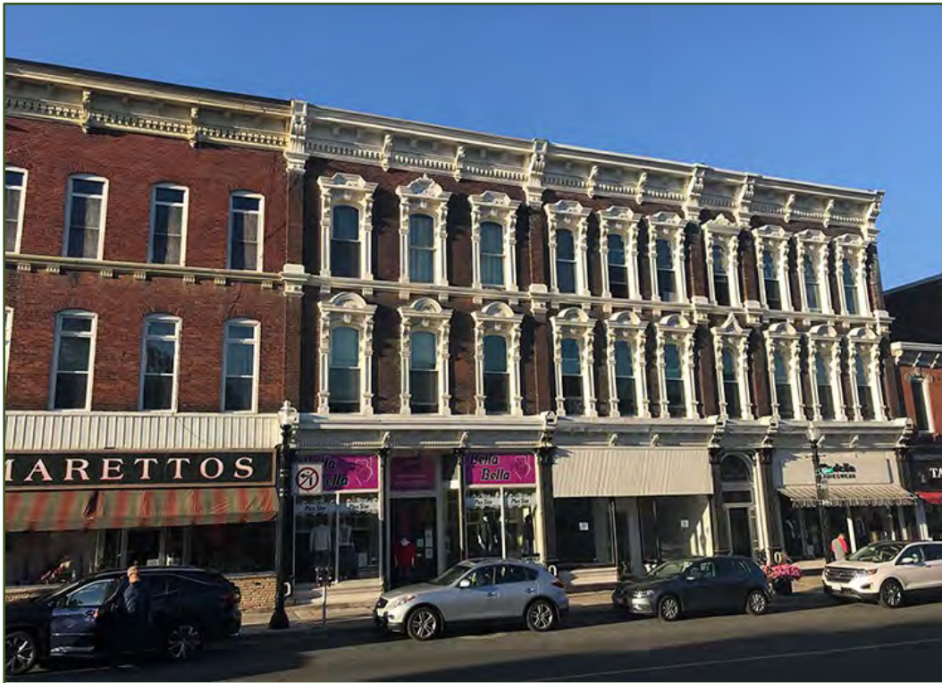
Restored façade of 11-13 King Street West. Photo by the author, September 2021.
