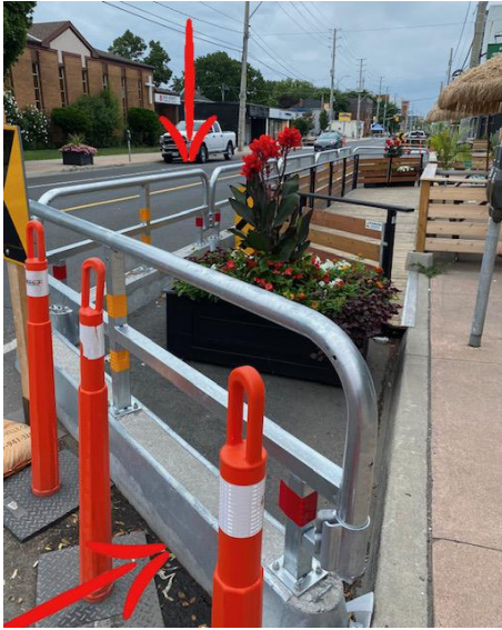
Metal frame to protect the patio or pedestrian walkway. Pylons included for added visibility .
