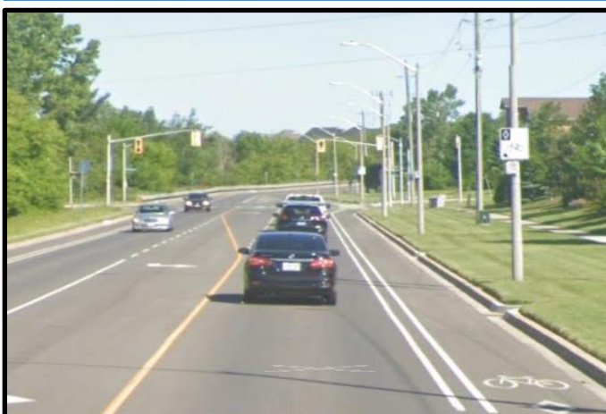
Stone Church Rd, Hamilton Uni-directional Bicycle Lanes with Painted Buffers
