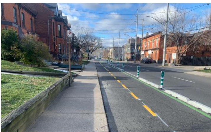
Hunter St, Hamilton Flexposts and precast curbs
