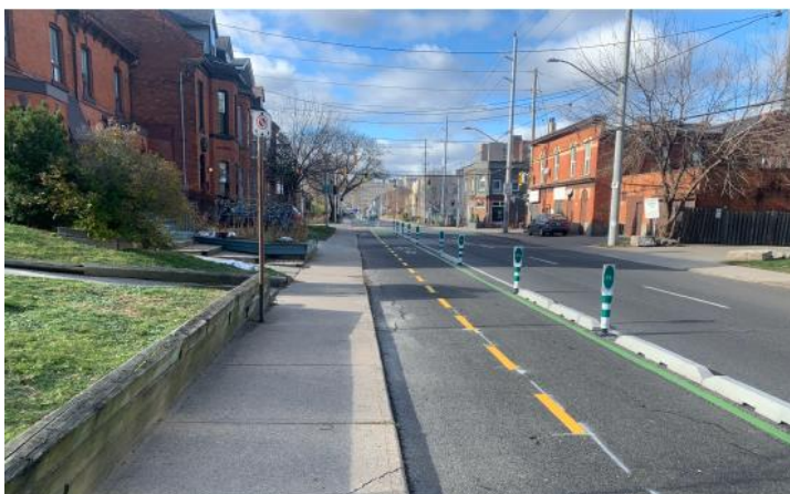
Hunter St, Hamilton Flexposts and precast curbs
