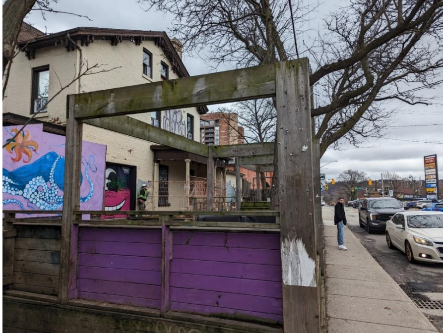
115-117 George Street, North and West (Front and Side) Elevations City of Hamilton, January 20, 2023
