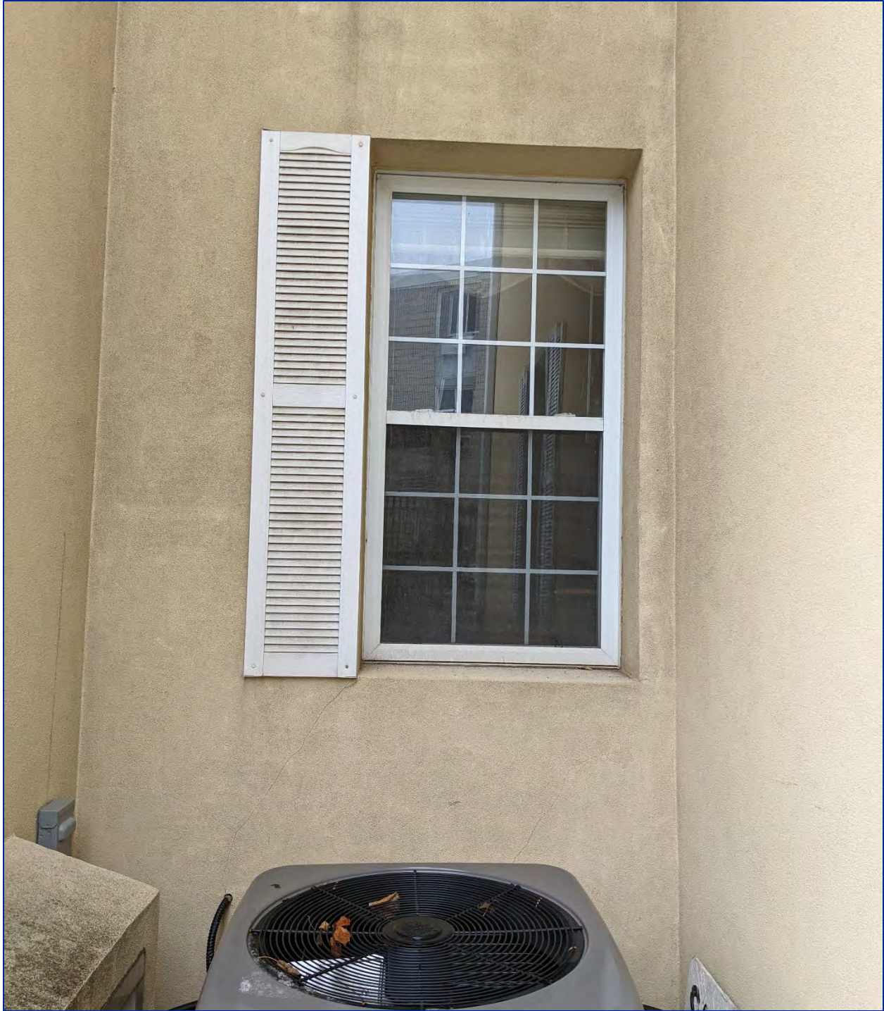
Figure 28: View of the windows in the sunken section of the east elevation
