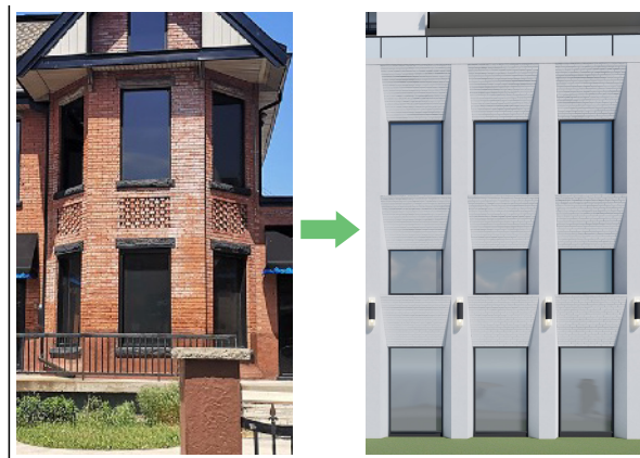
The main bay gable wall of 222 Main Street West is shown on the picture above. Bay gable walls are noticeable as a design feature on this building and have been considered in the design of the facade pilasters of the new building. The image on the right is an extract of an exterior facade wall showing this language used between each window bay. While the scale is different, the proportions are similar and articulate nicely the facade.
