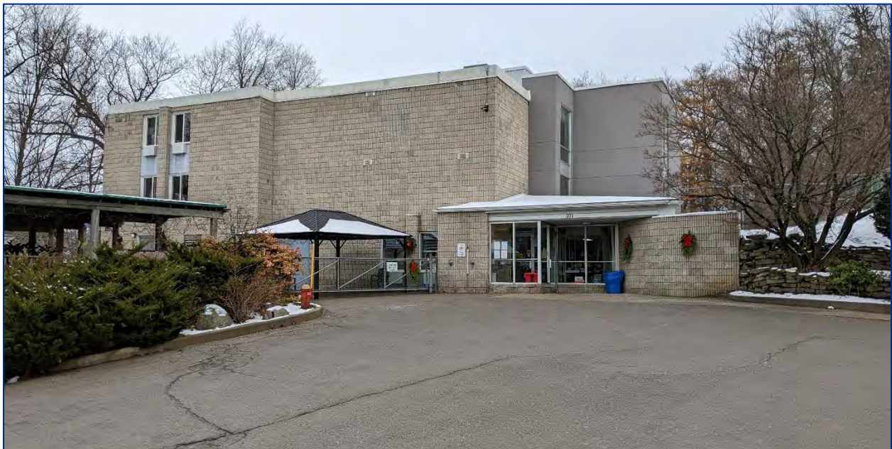
Figure 30: View of the west elevation of the continuing care centre
