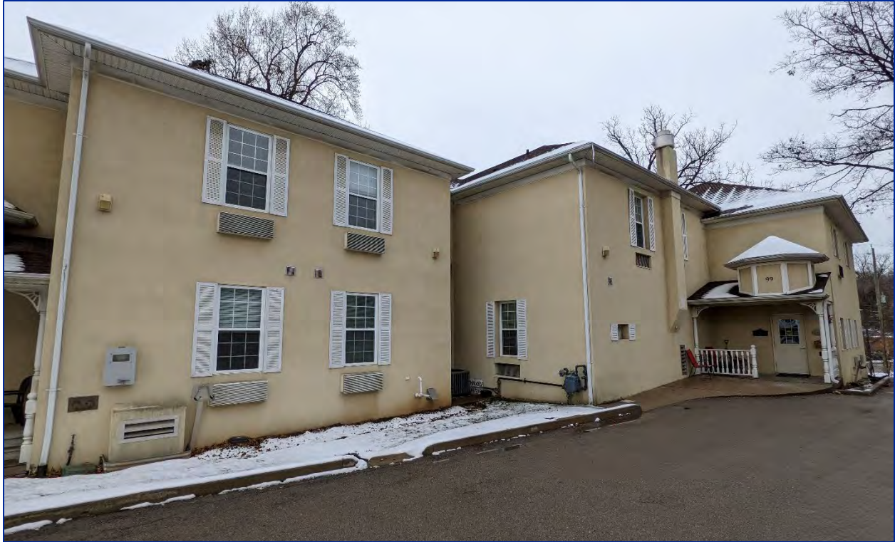
Figure 21: View of the east elevation of the retirement residence
