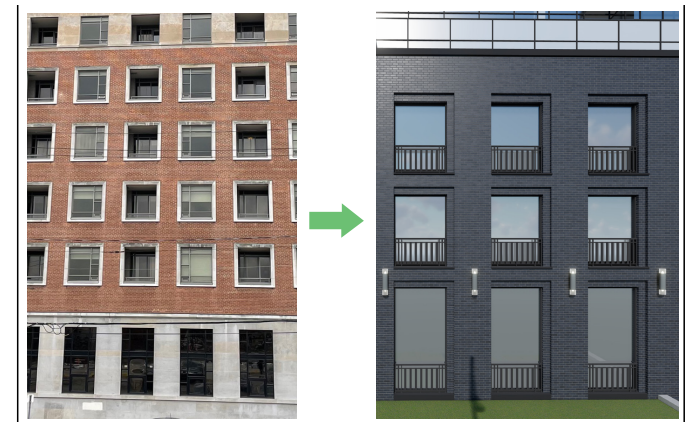
The left image is a portion of the facade of the former Revenue Canada building (an, located at the northeast corner of Caroline Street and Main Street, nearby the subject site). This fenestration pattern served as some guidance to suggest variance in the facade design for the project as can be seen on a fragment of the Main Street West facade.
