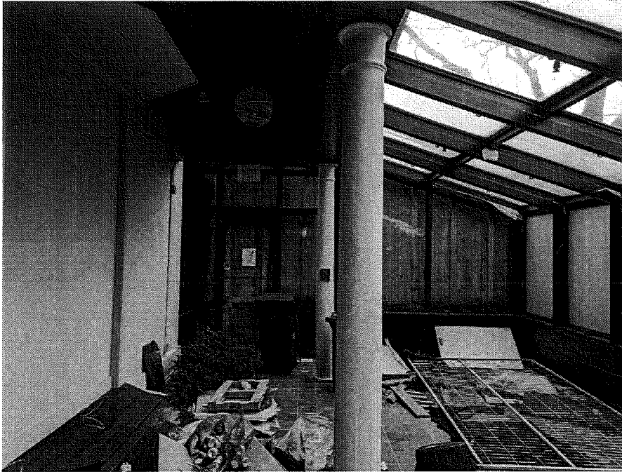
115-117 George Street, Front Sunroom Addition Facing West City of Hamilton, January 20, 2023
