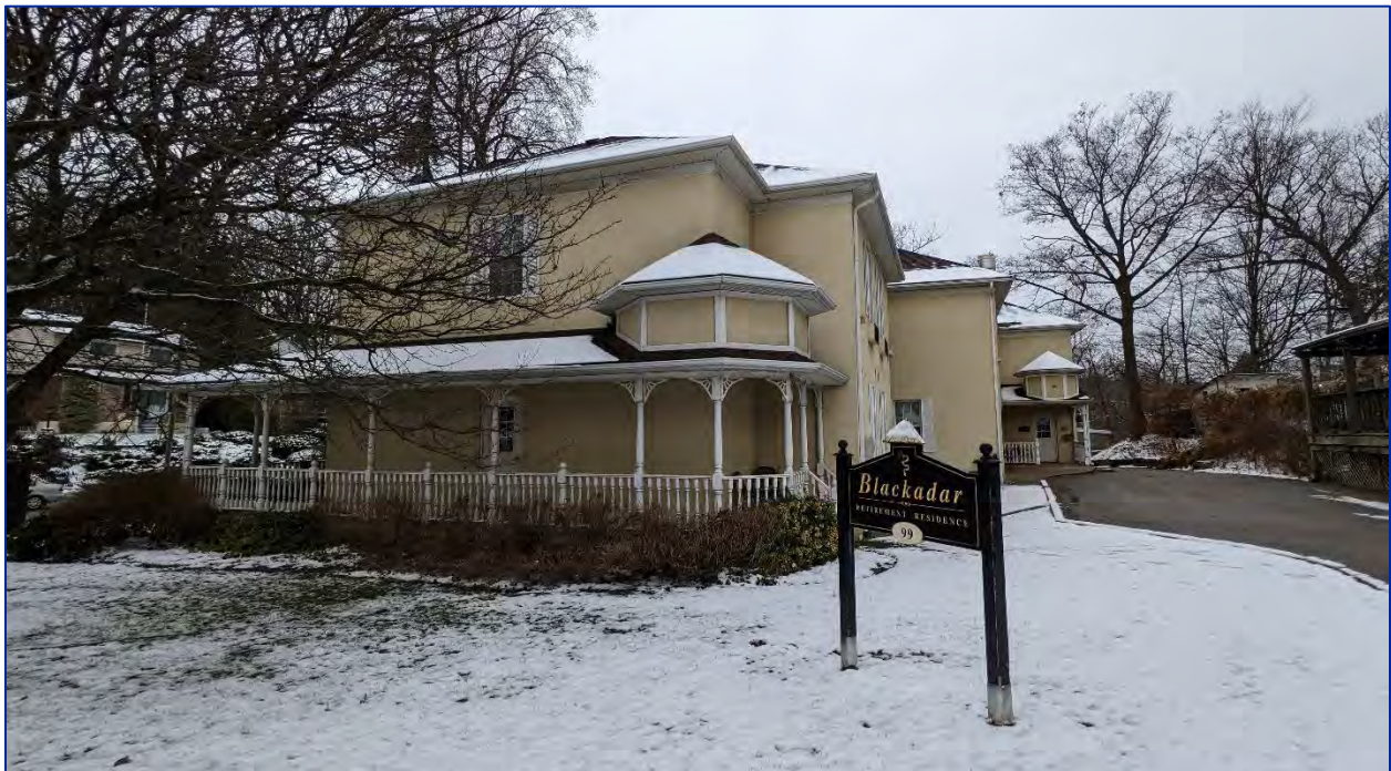
Figure 22: View of the south elevation of the retirement residence
