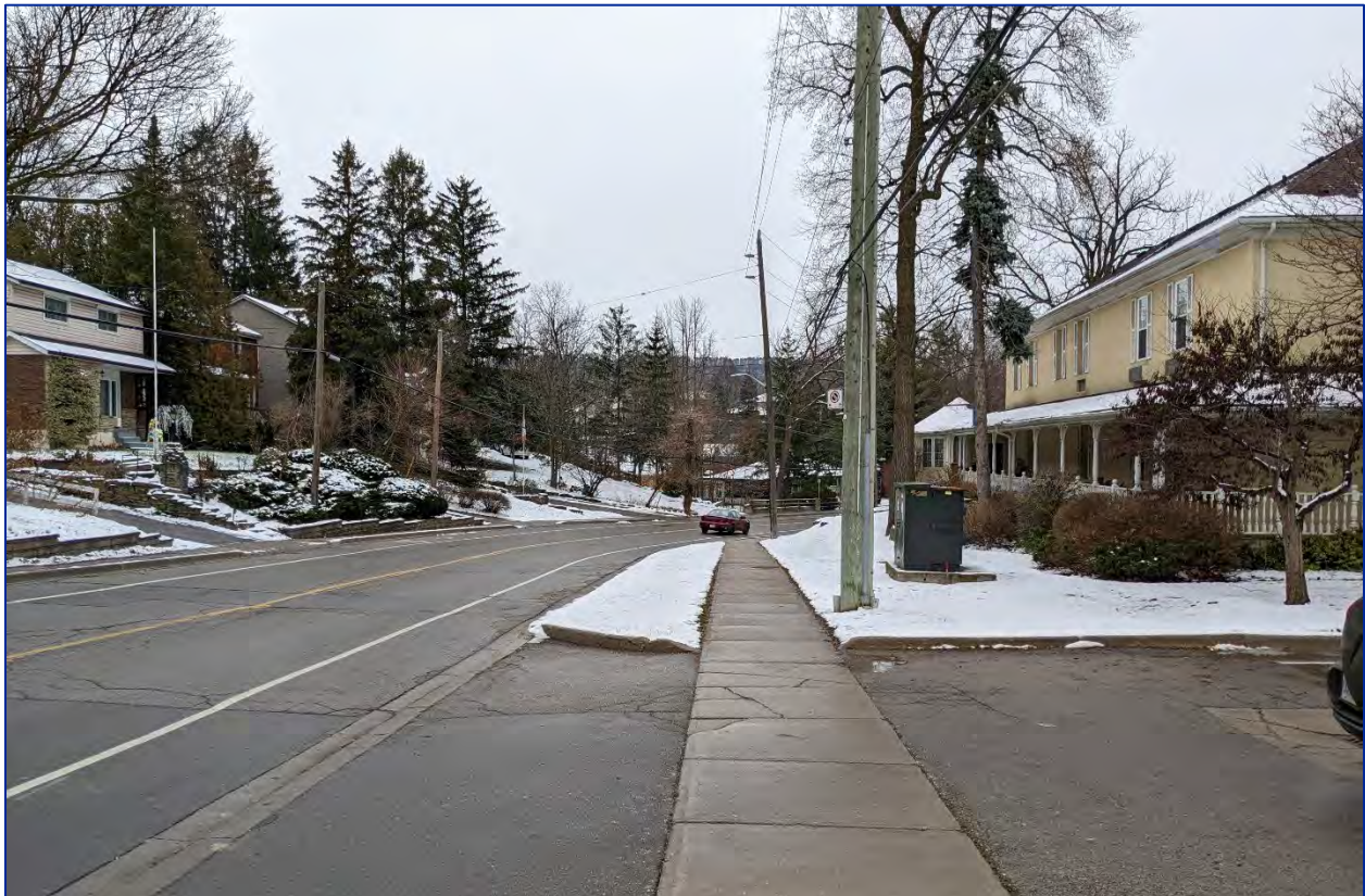
Figure 9: View north along Creighton Road from the ring-road driveway
