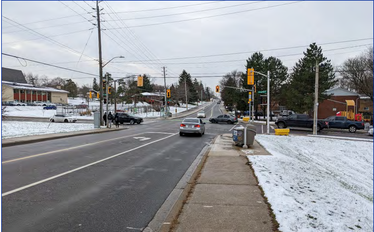
Figure 20: View of the intersection of Creighton Road and Governor's Road from east of the intersection
