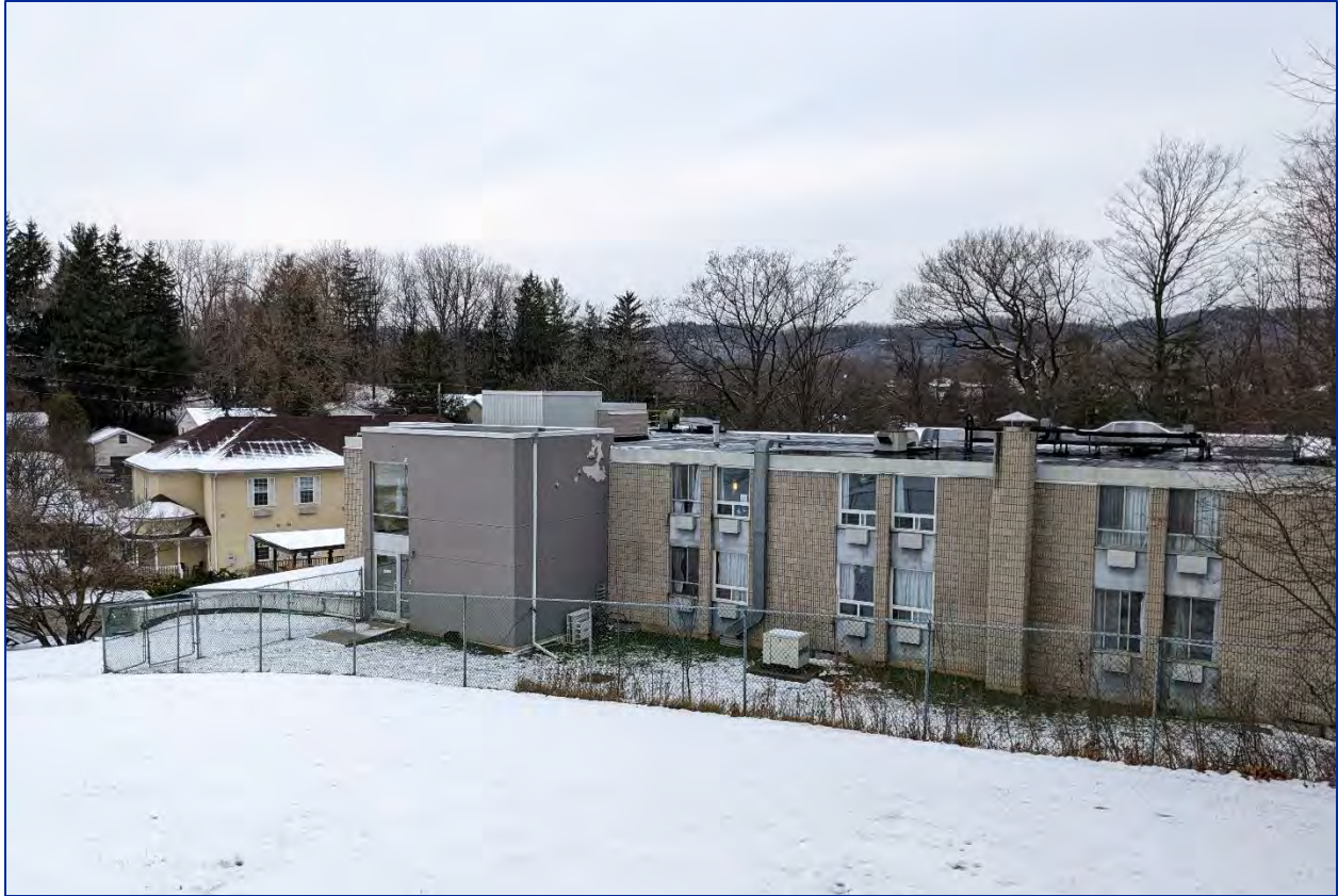
Figure 31: View of the south elevation of the continuing care centre
