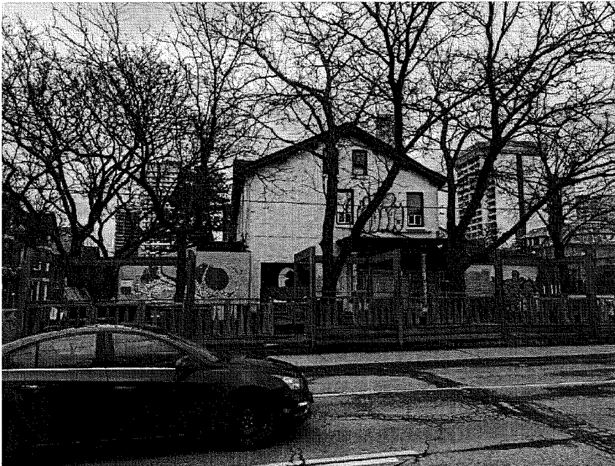
115-117 George Street, West (Side) Elevation City of Hamilton, January 20, 2023
