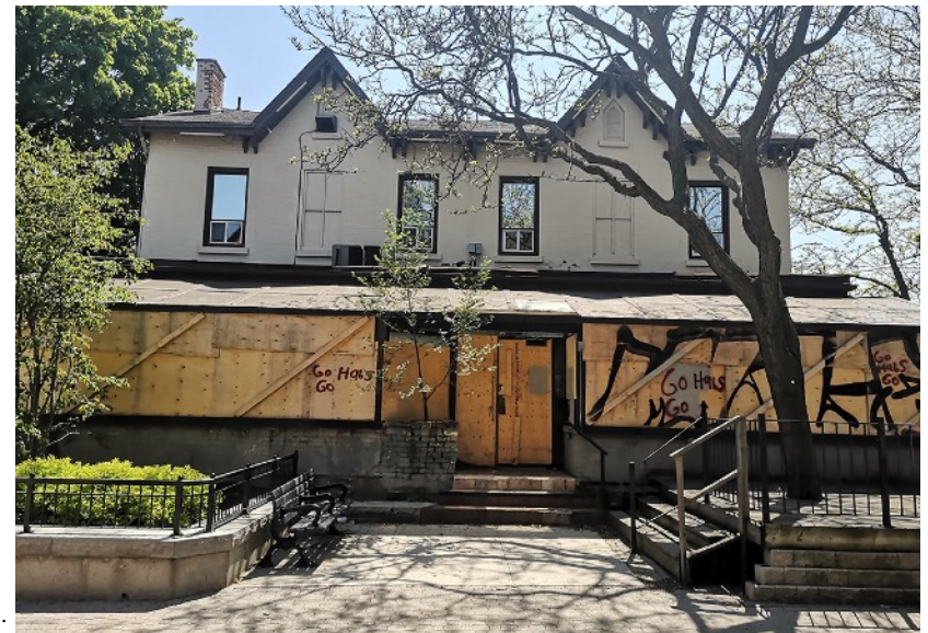
115-117 George Street in its current condition.
