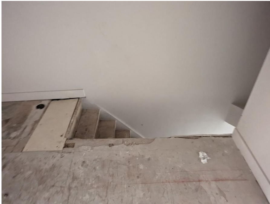
115-117 George Street, Attic Stairs City of Hamilton, January 20, 2023
