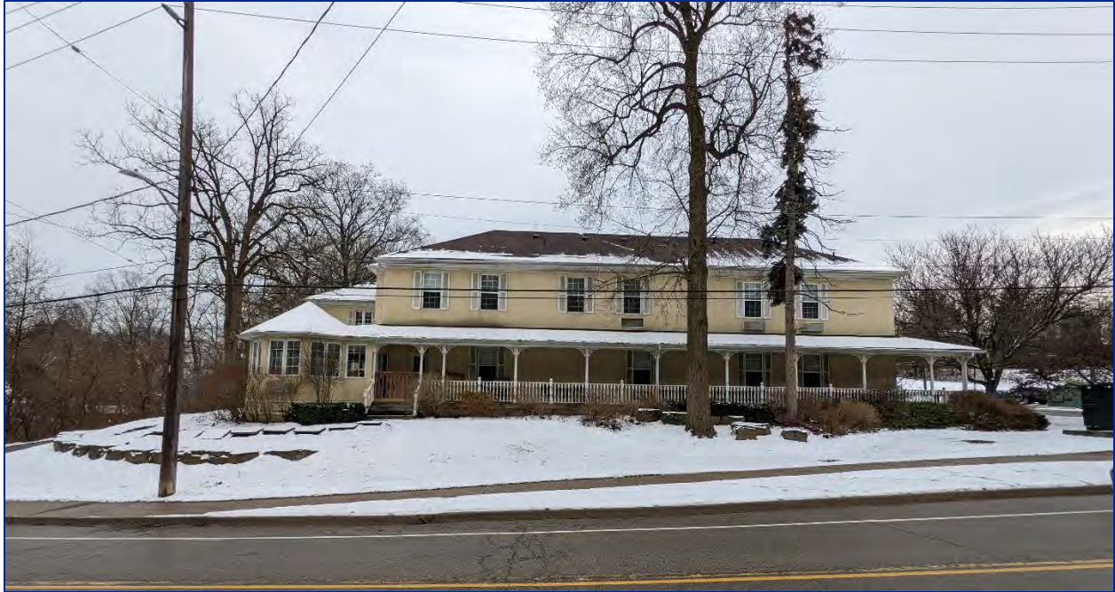
Figure 23: View of the west elevation of the retirement residence
