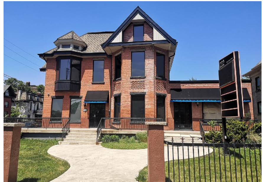
222 Main Street South in its current condition.
