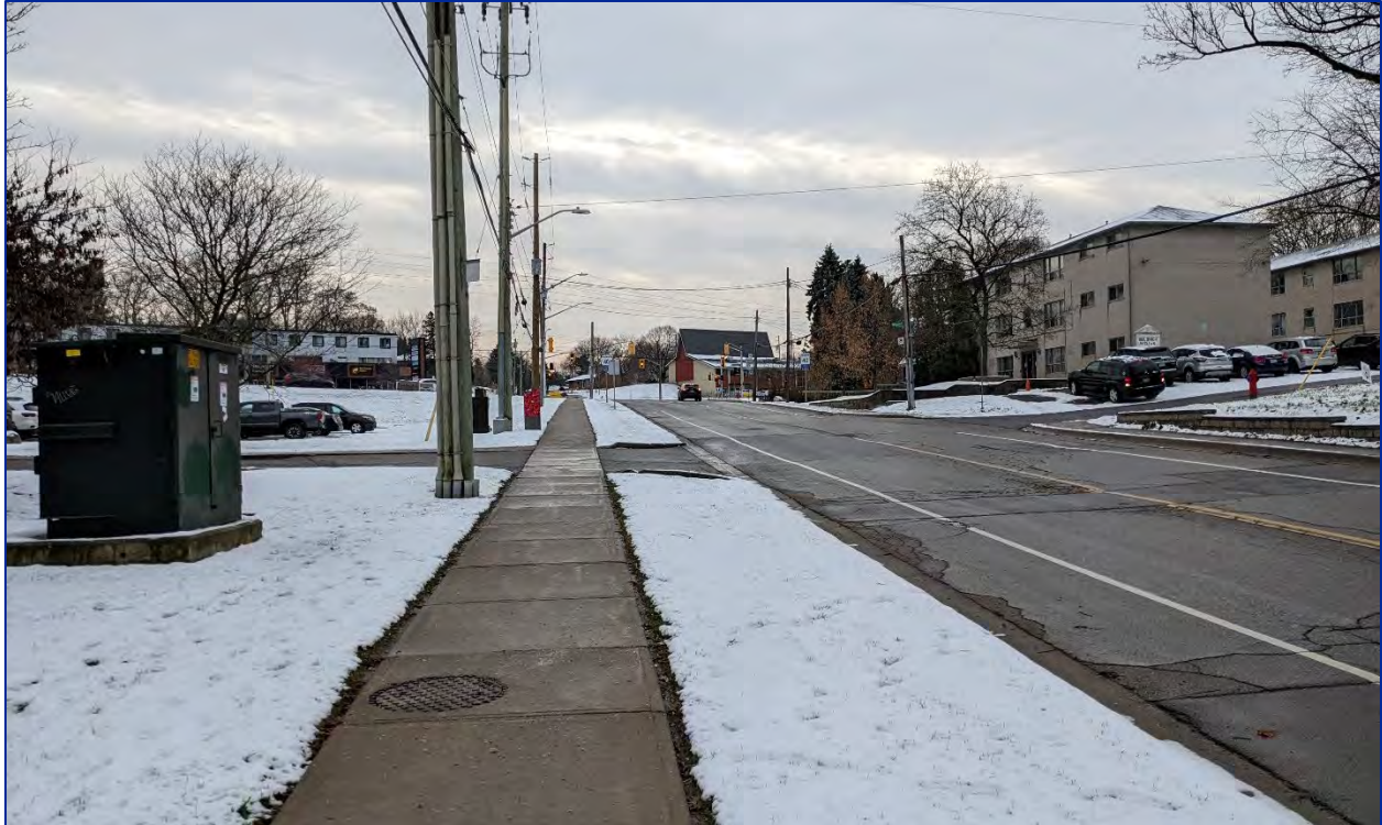
Figure 10: View south along Creighton Road from between the ring-road driveway entrances
