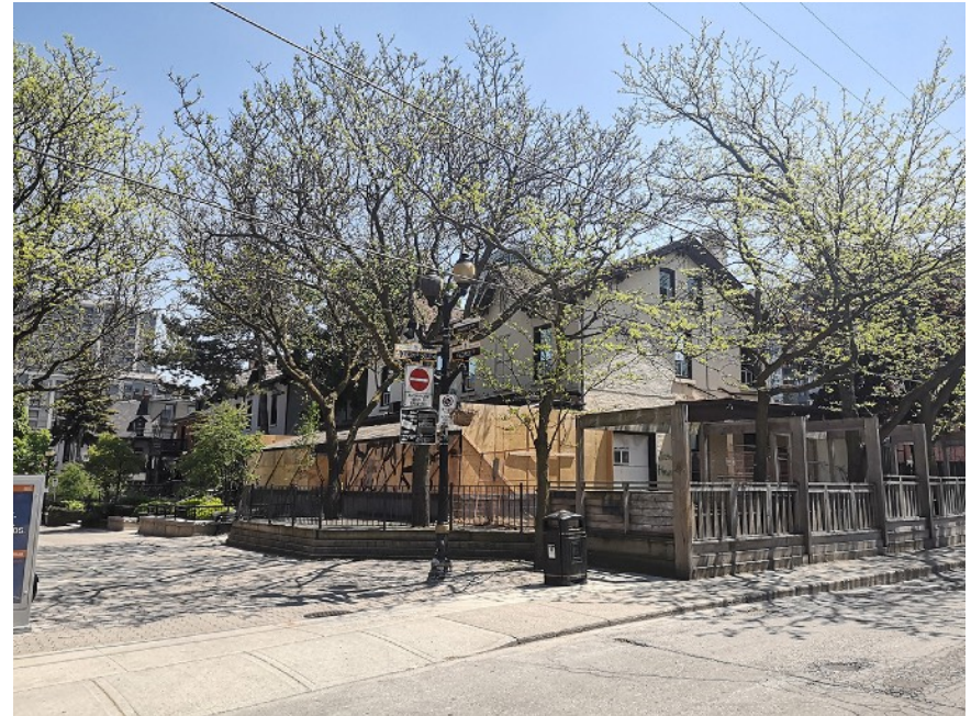
115-117 George Street as seen from the intersection of George Street and Queen Street South, which is partly obscured by trees, and later additions when the building was converted for commercial usage.
