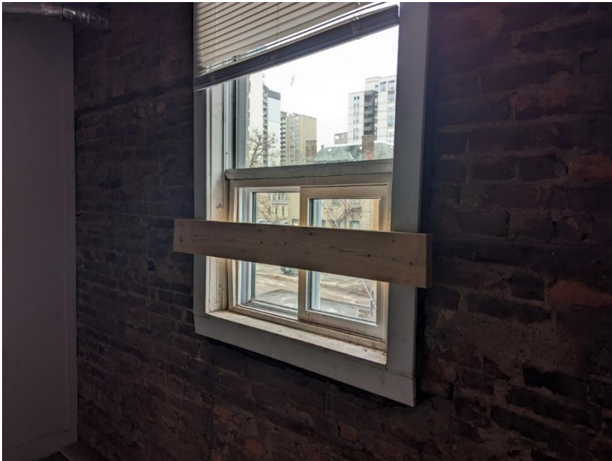
115-117 George Street, Window Opening City of Hamilton, January 20, 2023
