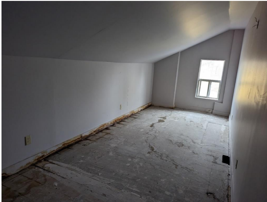
115-117 George Street, Attic room City of Hamilton, January 20, 2023
