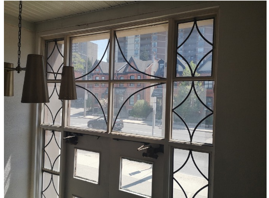
Interior view of 220 Main Street, taken inside the front addition, looking towards Main Street. and the new front entrance assembly. Windows are painted metal units with single pane glazing with lead came.
