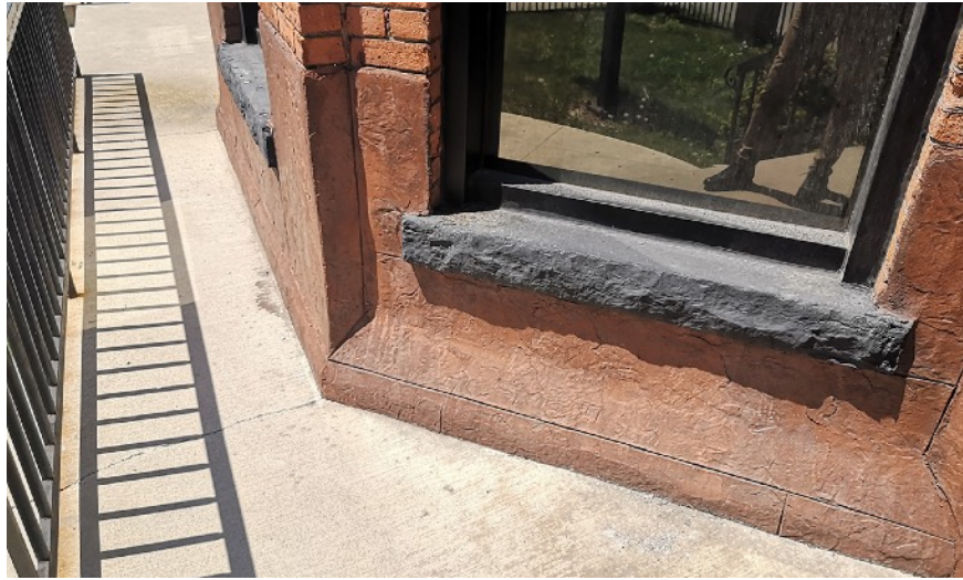
Close-up of base, showing parging over brick surface at base.
