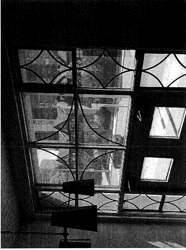
Interior view of 220 Main Street, taken inside the front addition, looking towards Main Street. and the new front entrance assembly. Windows are painted metal units with single pane glazing with lead came.
