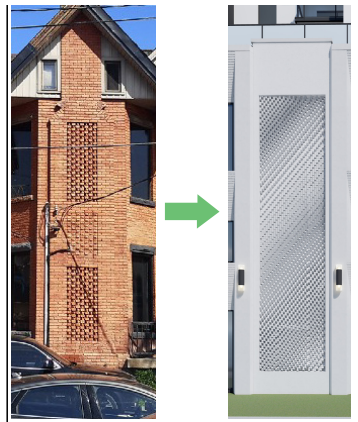
The side bay gable wall of 222 Main Street West includes some decorative brick pattern. This brick treatment on the existing building can be used to propose a contemporary brick pattern on a proposed segment of the new massing.
