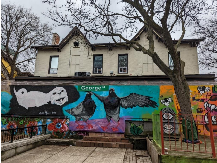
115-117 George Street, North (Front) Elevation City of Hamilton, January 20, 2023
