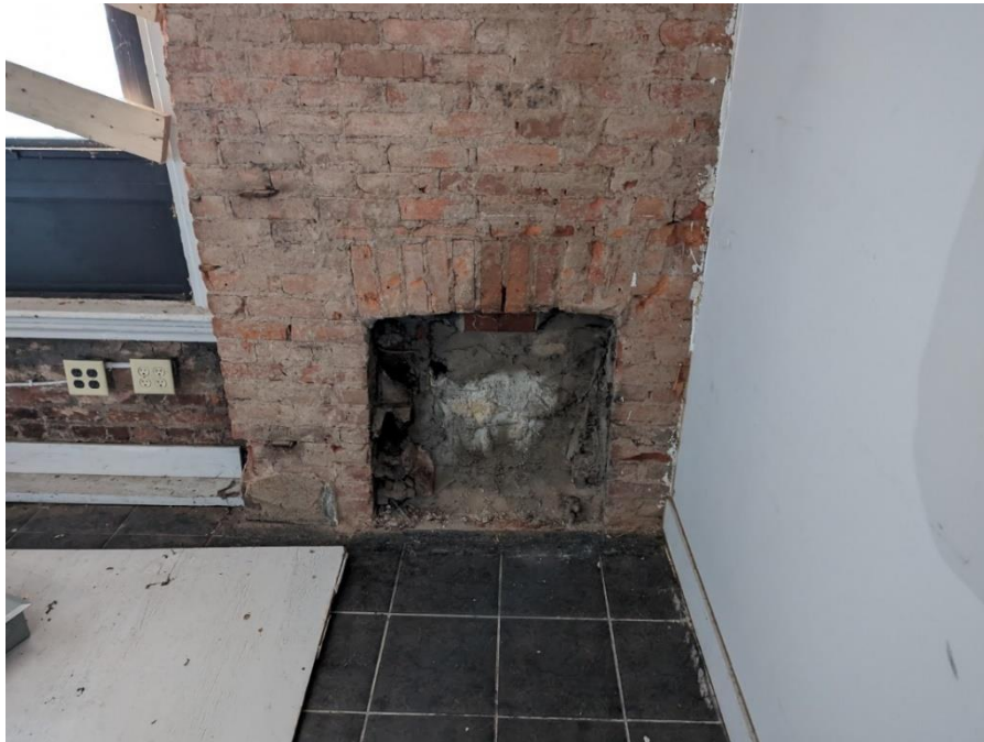
115-117 George Street, Interior Brick Fireplace City of Hamilton, January 20, 2023
