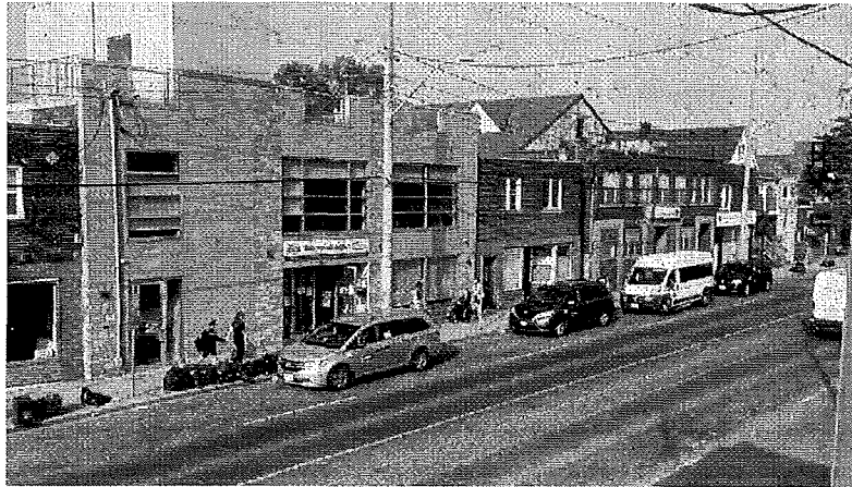
Figure 5 Morning drop off at PSSQL, on foot and by DARTS vehicles. The proposed injection clinic is ~30m away, indicated with the arrow.
