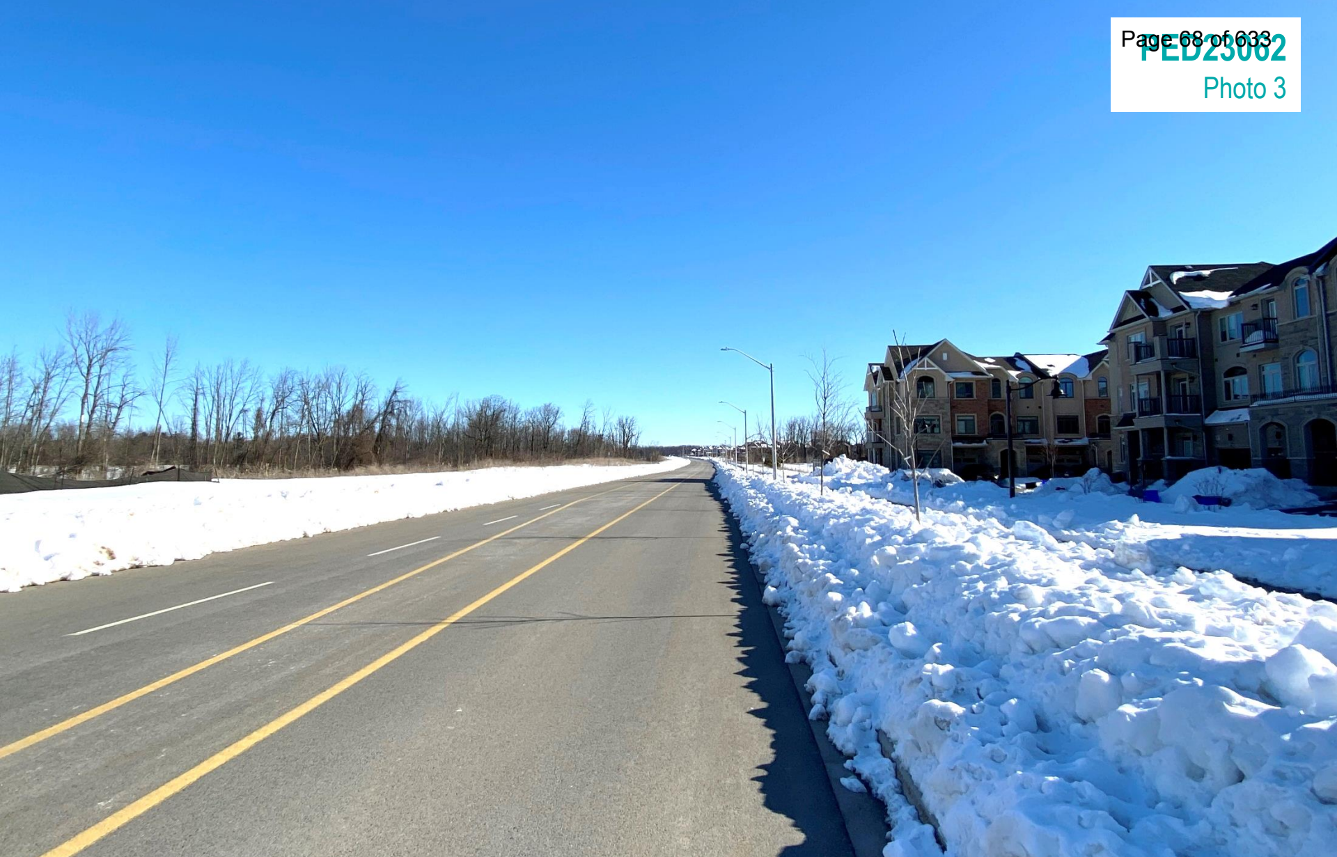
View on North Waterdown Drive looking away from Mosaic Drive
