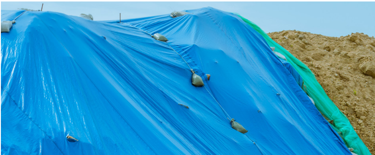
■ Protecting a stockpile.
