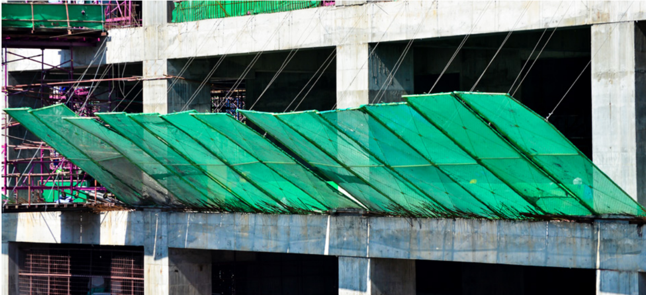
■ Above: Construction screen on temporary panels blocks vision, dust and debris
